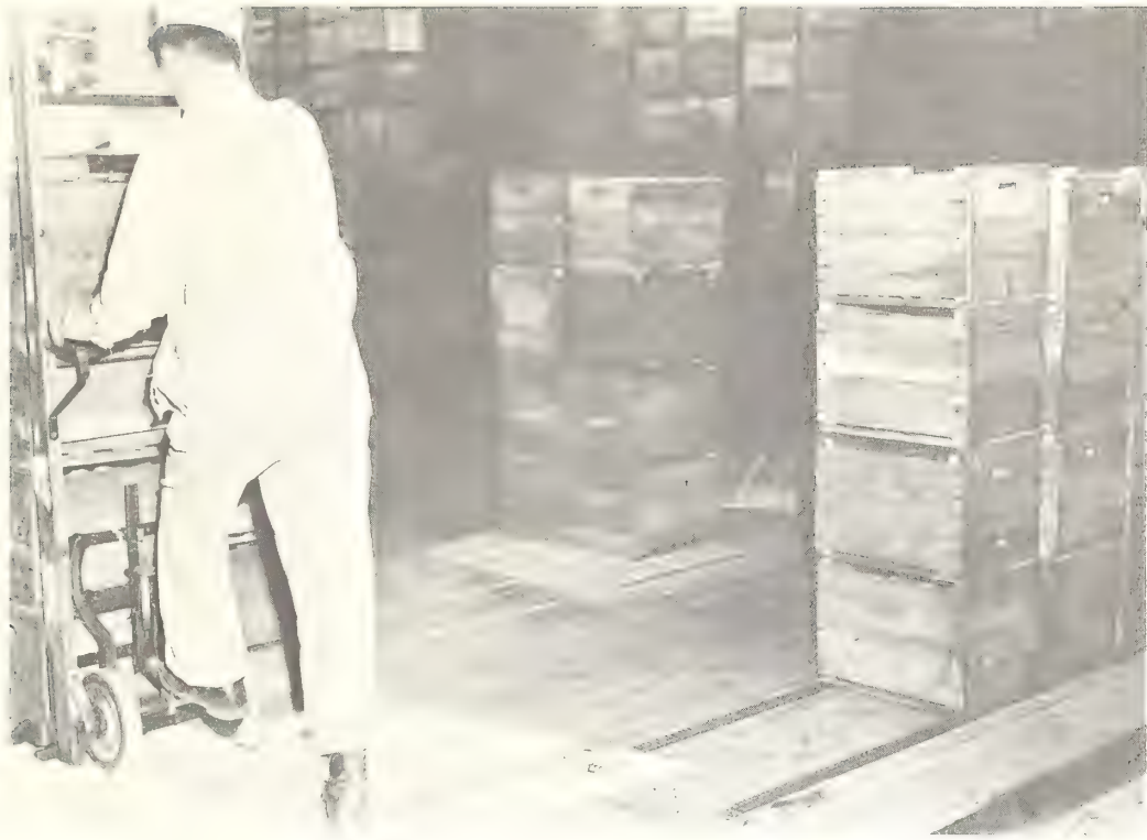
Figure 8.--Clamp type 2-wheel handtruck operator pushing his truck across the surface of an empty pallet in order to reach a load.
