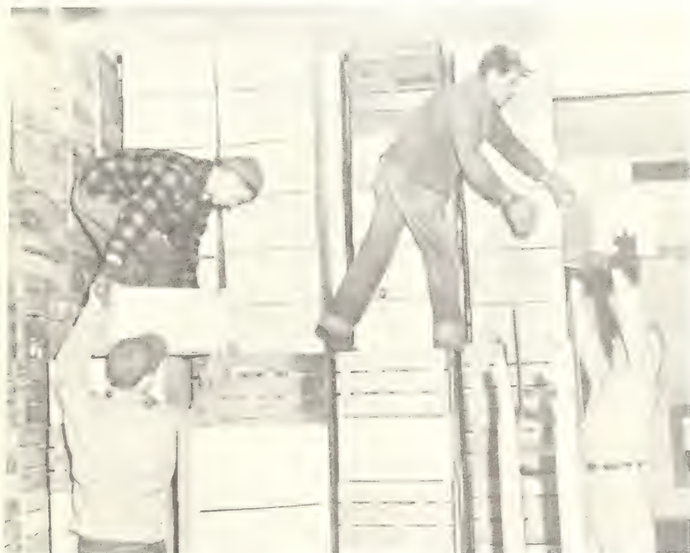
Figure 1.--Manual high-piling. One stacker lifts crate up to second stacker who places it in storage.
