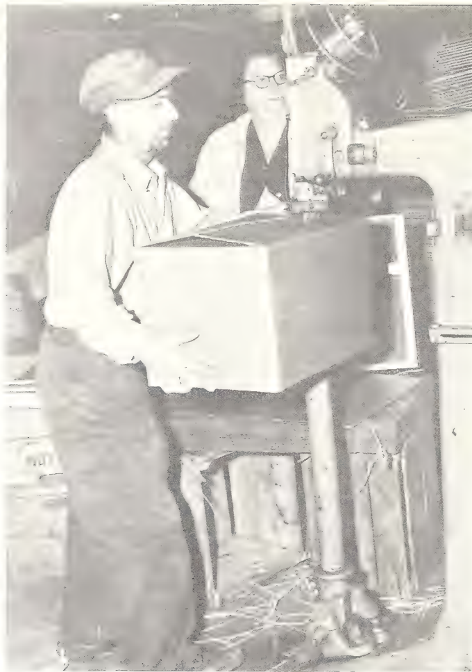
Figure 25.--Worker stapling carton together with a motorized stapling machine.
