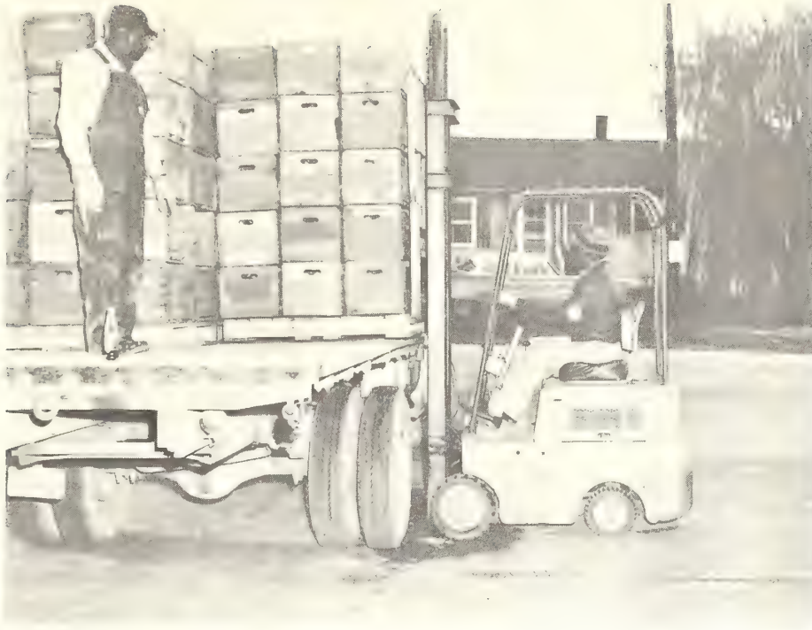
Figure 5.--Forklift truck removing loaded pallet from orchard truck. Note concrete apron and uncluttered appearance of receiving area.
