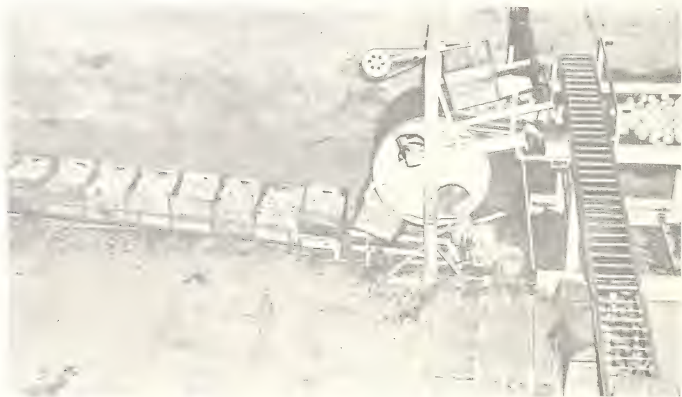
Figure 11.--Two workers at a manual dumping station. One worker keeps a full crate in readiness for second worker who tips apples out onto spreader belt. Dumper disposes of empty crates on belt conveyor.
