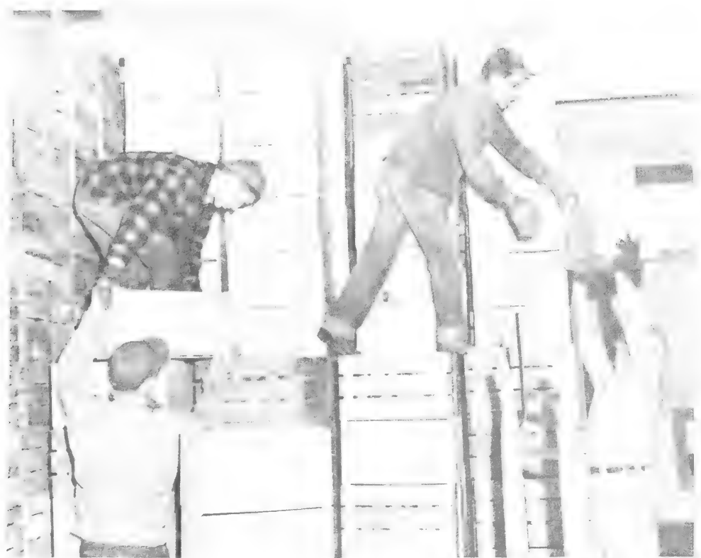
Figure 1.--Manual high-piling. One stacker lifts crate up to second stacker who places it in storage.
