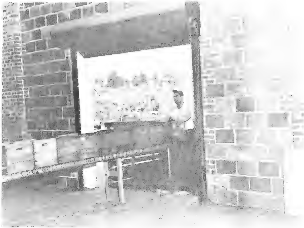
Figure 3.--An unloader places crate on gravity conveyor from an orchard truck.
