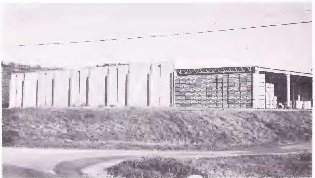
Figure 14.--Wall panels braced in position ready for joining with poured pilasters; suspension frame for blower units and catwalk in foreground.
