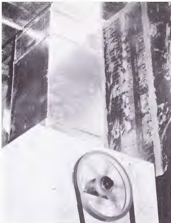
Figure 5.--Cold diffuser in a controlled-atmosphere room. (Note the sealing of the metal wall sheets).
