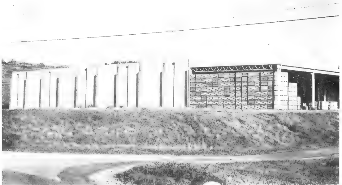
Figure 14.--Wall panels braced in position ready for joining with poured pilasters; suspension frame for blower units and catwalk in foreground.
