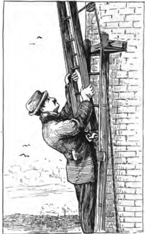
CHIMNEY OF CLARK THREAD WORKS, SHOWING METHOD OF ASCENT.
