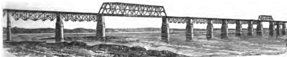
VIADUCT BRIDGE AT LOUISVILLE.
