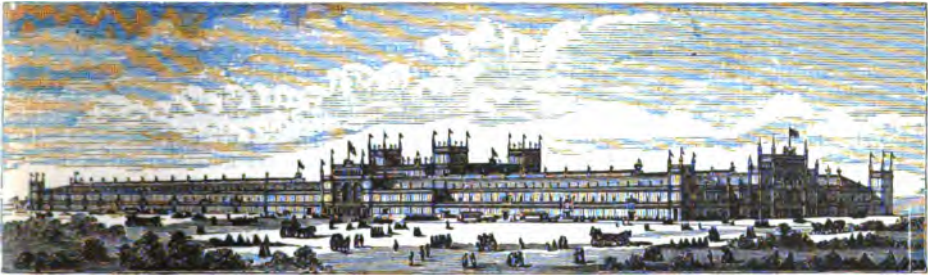
MAIN EXHIBITION BUILDING.
