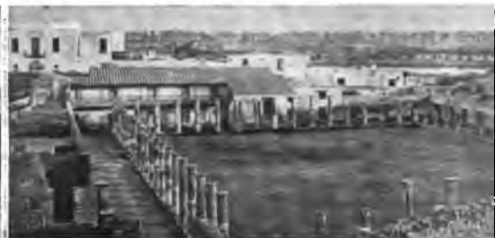
THE BARRACKS OF THE GLADIATORS, BUILT AT THE BACK OF THE THEATRE AND USED ALSO FOR A PRACTICE COURT.
