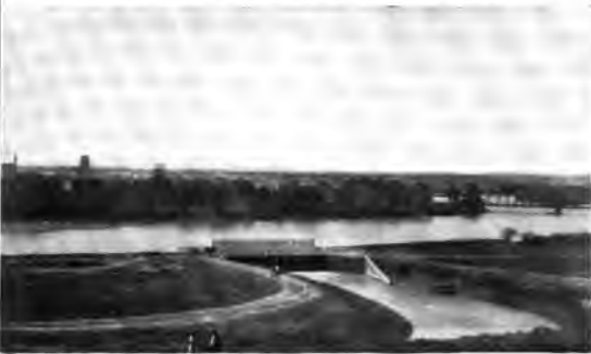
THE MAIN CANAL OF CANADA'S 3,000,000-ACRE RECLAMATION PROJECT.
