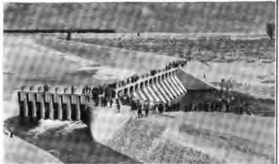
THE OPENING OF THE UNITED STATES TRUCKEE-CARSON PROJECT (NEVADA). THIS SYSTEM WILL ULTIMATELY IRRIGATE 575,000 ACRES. THE DAM IS BUILT OF SOLID CONCRETE.
