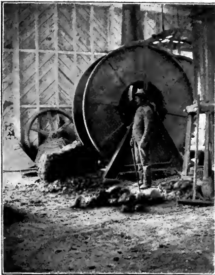
HORRY FURNACE, SHOWING CARBIDE JUST REMOVED.
