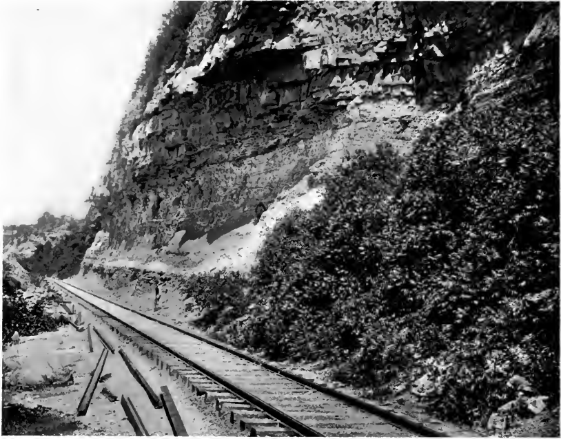
FIG. 5.—Showing extent of erosion at base of the Niagara shale since 1854. (See description in the text.)
