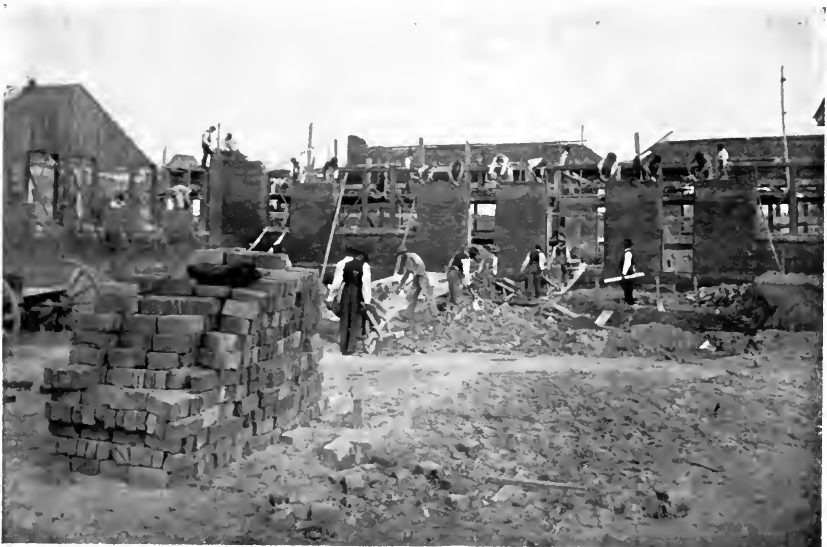
STUDENTS AT WORK ON NEW TRADES-SCHOOL BUILDING.
