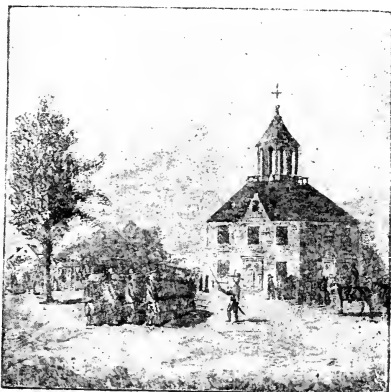
THE OLD TUNNEL MEETING HOUSE.
