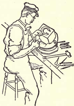
FIG. 204.—Die-sinking.
