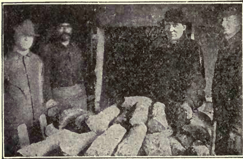
FIG. 184.—Inspection of Pig Iron. The amount and kind of pig iron is carefully determined before it is placed in the cupola. This illustration shows the inspection of the pig iron before it is dumped into the furnace. Notice the shape of the bars.
