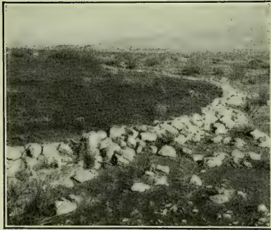
FIG. 6(b). Partially breached rock spreader built by C.C.C. about 1938. San Simon Valley near Rodeo, New Mexico. Photo shows slight increase in vegetation on alluvial fill behind spreader. Photo taken October 1948.
