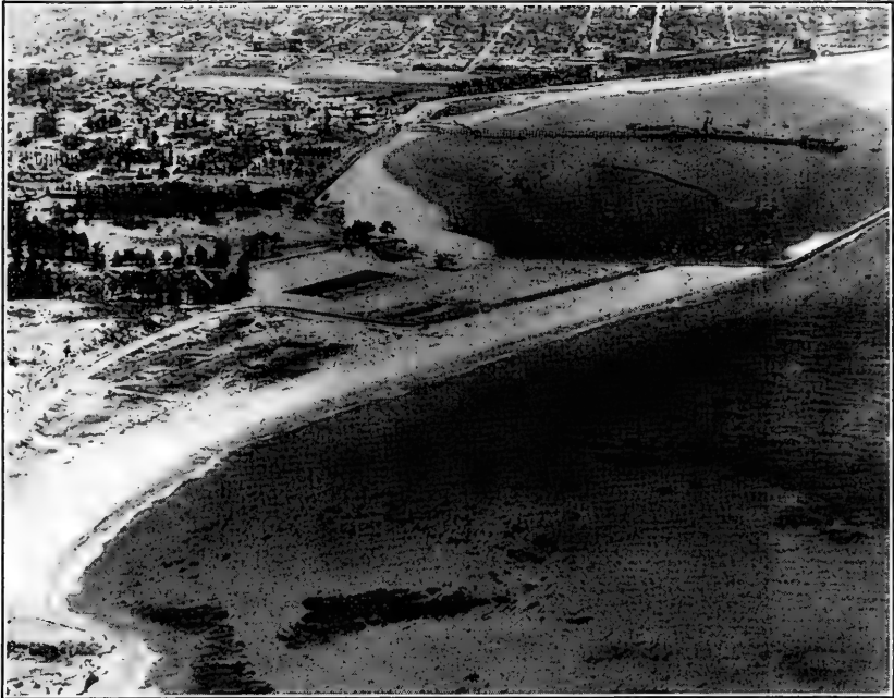
FIG. 3. Santa Barbara, California. Littoral material impounded by harbor breakwater and passing into harbor. June 1938. (Photo by Beach Erosion Board.)
