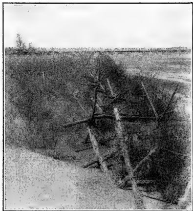
FIG. 7(c). Deposition induced by tetrahedrons with willows and other types of shrubs. Chinle Wash near Chinle, Arizona.
