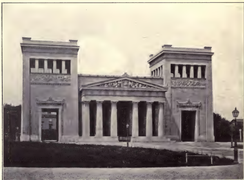
GATEWAY BUILDING (PROPYLAEA), MUNICH
