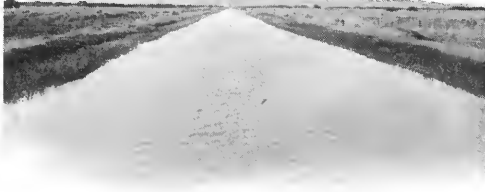
Palo Verde's Main Irrigation Canal
