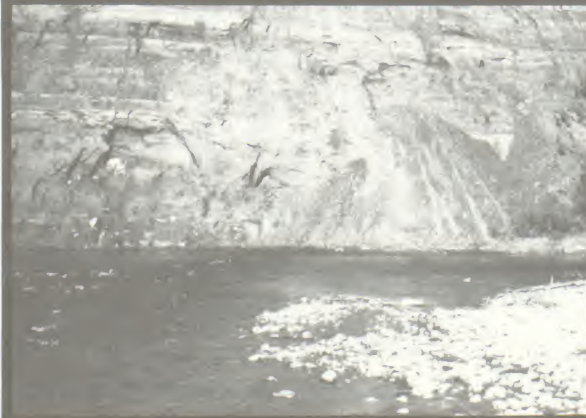
High, unstable sand and gravel bank at km 15.
