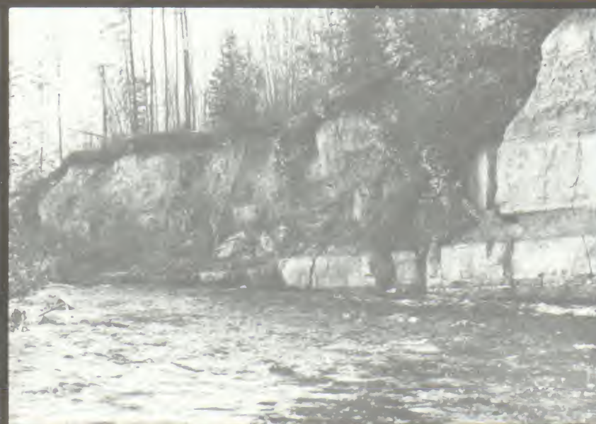
Unstable bedrock and gravel bank at km 7.
