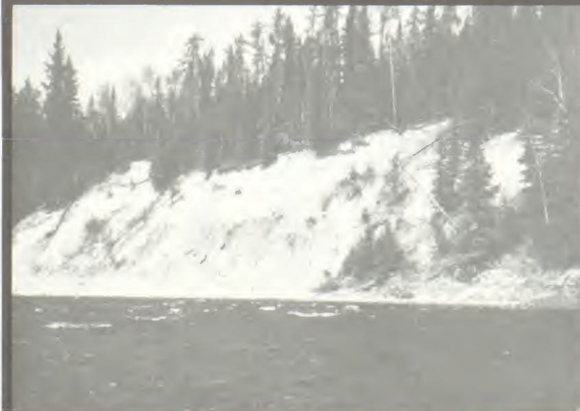
Unstable sand and clay bank at km 109.5.
