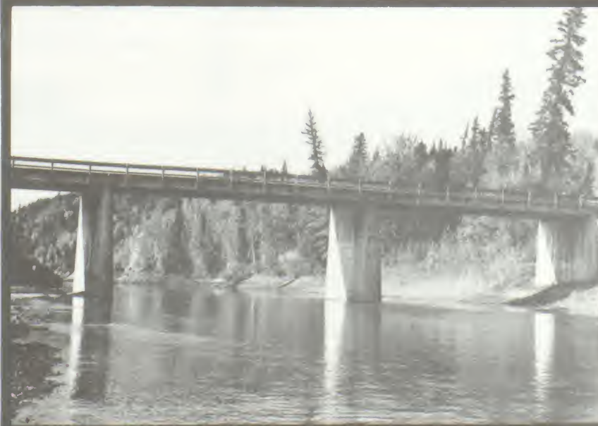
Bridge on highway 63 at km 0.6
