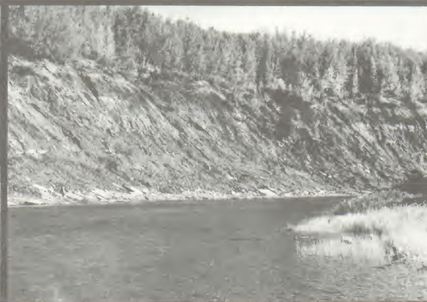
High, eroding bank of sand and silt at km 63.8.
