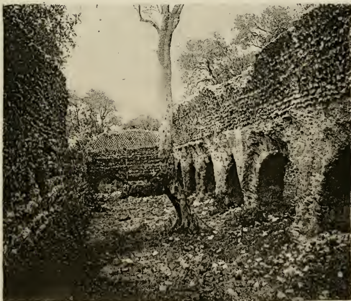
RESERVOIR OF AQUA MARCIA INTERIOR
