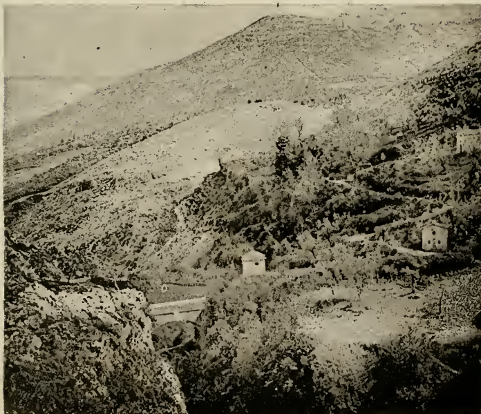
THE THIRD LOCH AND THE BRIDGE
