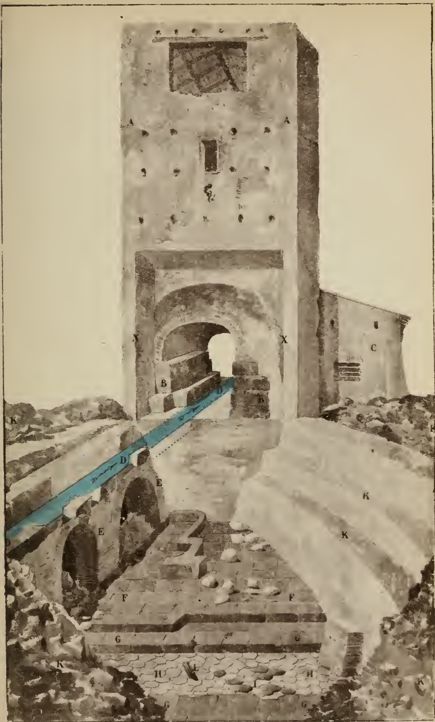
THE APIAN AQUEDUCT PASSING OVER THE PORTA CAPENA AND THROUGH THE TOWER
