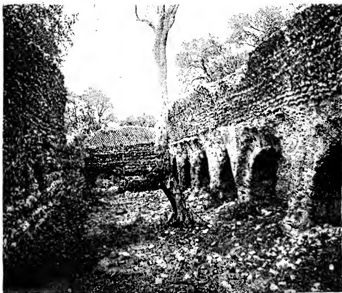
RESERVOIR OF AQUA MARCIA INTERIOR.
