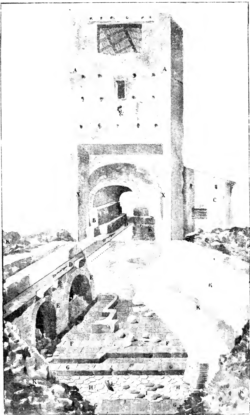
THE APPIAN AQUEDUCT PASSING OVER THE PORTA CAPEÑA AND THROUGH THE TOWER
