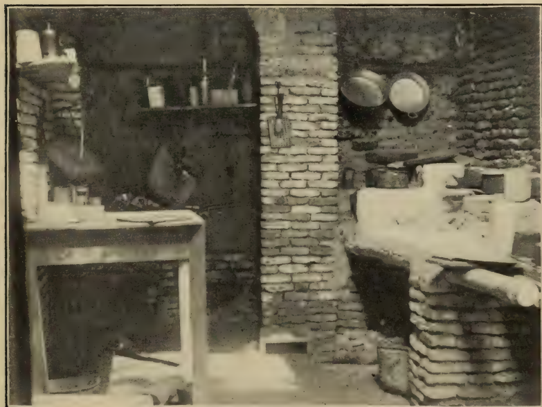
THE KITCHEN OF THE OLD MISSION HOUSE, BUSRAH
