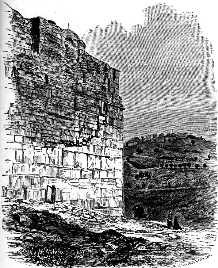
EAST END OF SOUTH WALL.
