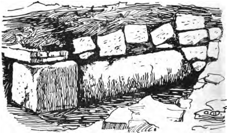
FIG. 18.—PILLAR BUILT INTO ANGLE OF A BARRACK-BLOCK.
