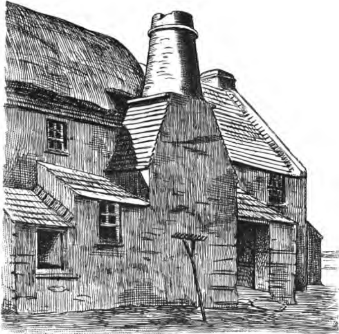
Fig. 12.—Old Farm-House at Rhosson Uchaf: Exterior View of Recess, Round Chimney, and Porch.
