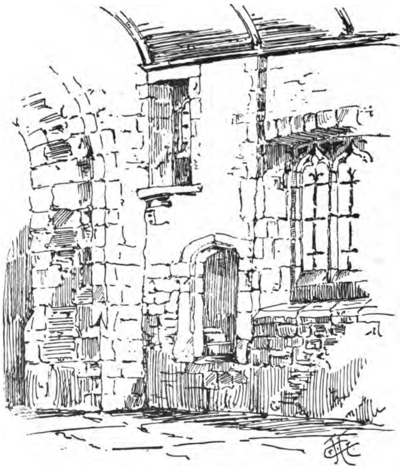
Fig. 5.—Rood-Staircase in Llandenny Church.
