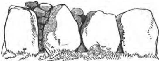
Walling on the sea side.
