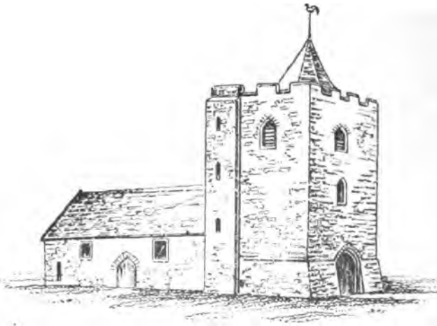
Llanilar Church before Restoration.
