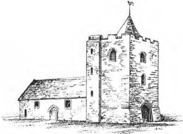
Llanilar Church before Restoration.
