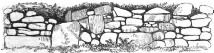
Chûn Castle. Masonry of outer Wall.
