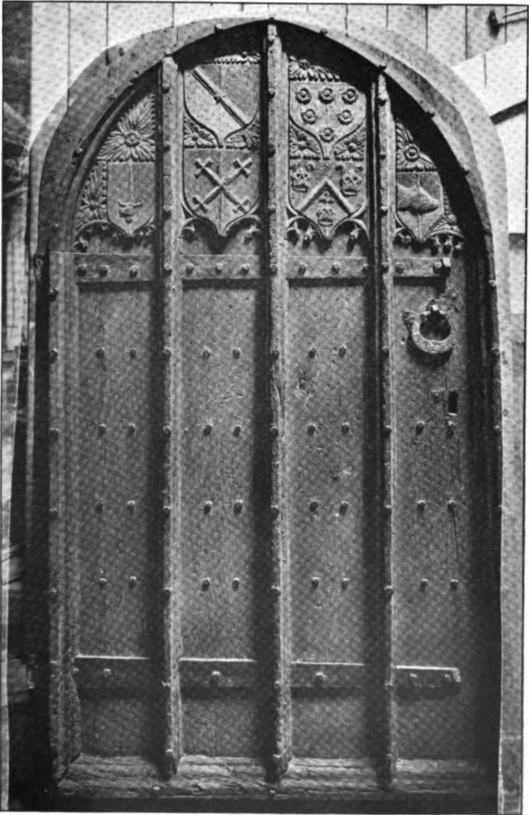
GILESTON CHURCH.—SOUTH DOOR.
