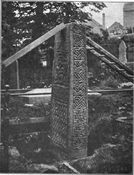
Fig. 1.—The Iltyd Cross, shored up preparatory to its removal.
