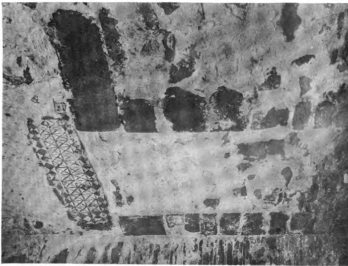
LLANVILLO CHURCH, BRECKNOCKSHIRE. BUILT-UP DOORWAY IN SOUTH WALL, WITH DIAPERED LINTEL.
