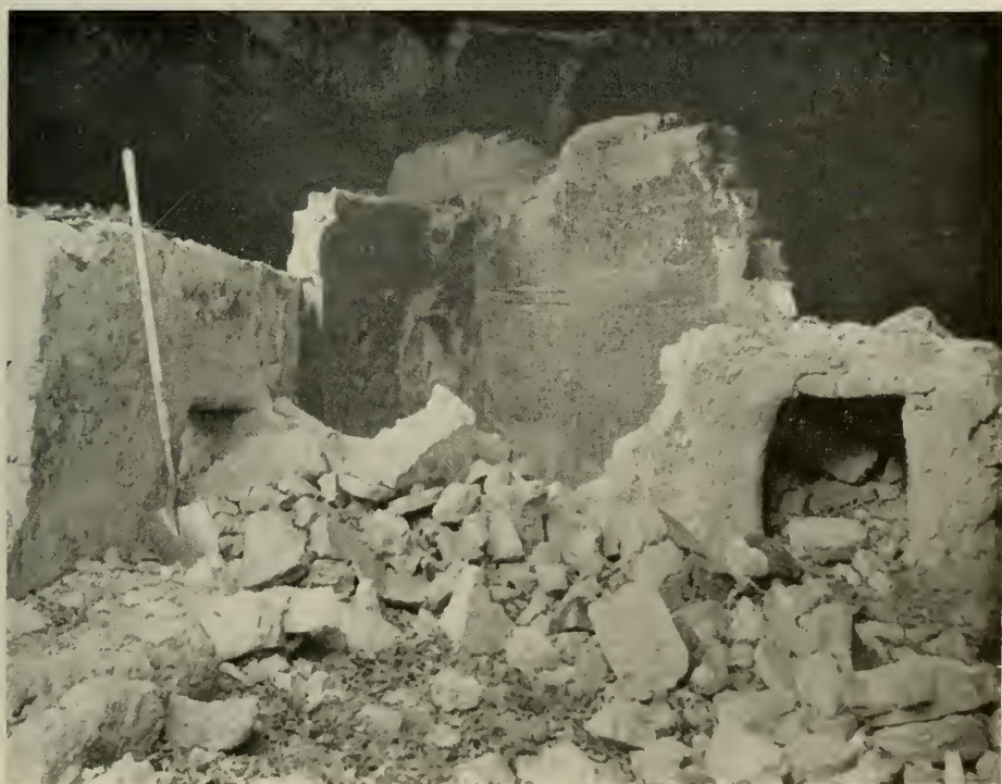
B. Dark Cave. The poorly preserved nature of the puddled adobe mud walls of rooms in the outer portion of the cave is shown.
