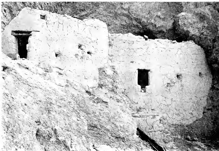
B. Arch Cave. Rooms were built on the steeply sloping floor of this shallow cave. Dirt fill was placed within the rooms to level the floors
