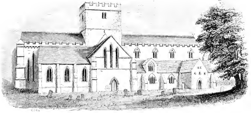
North View of St John the Evangelist, Brecon
