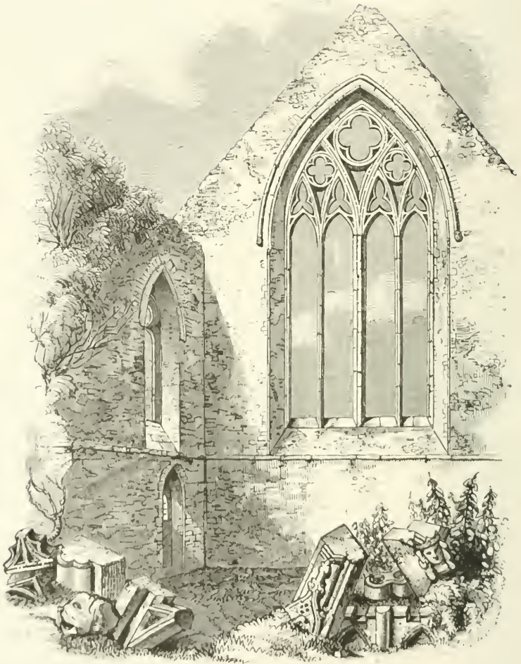
West End of the Refectory
