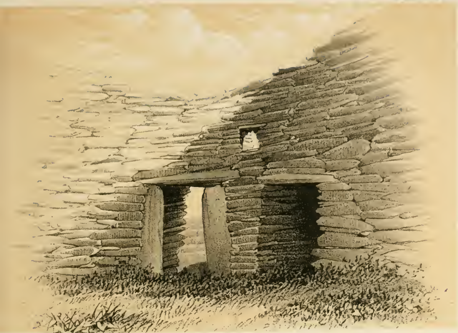
CLOGHAUN N o 12. INTERIOR VIEW
