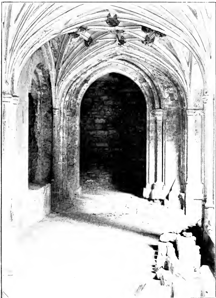
EASTERN PROCESSION DOORWAY.
