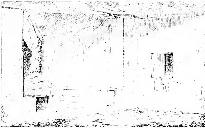
Perspective view of the hemicycle, with cornice left unfinished on the roof.
