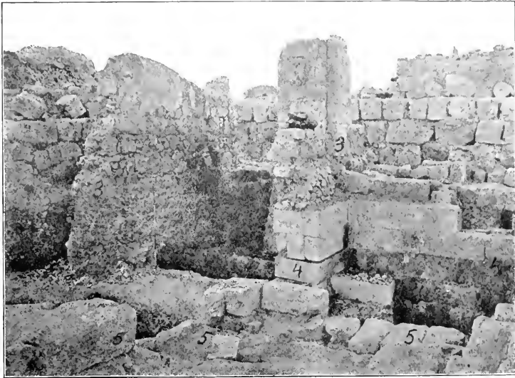
FIG. 42. WALLS OF BUILDINGS AT SAMARIA (after Reisner).
