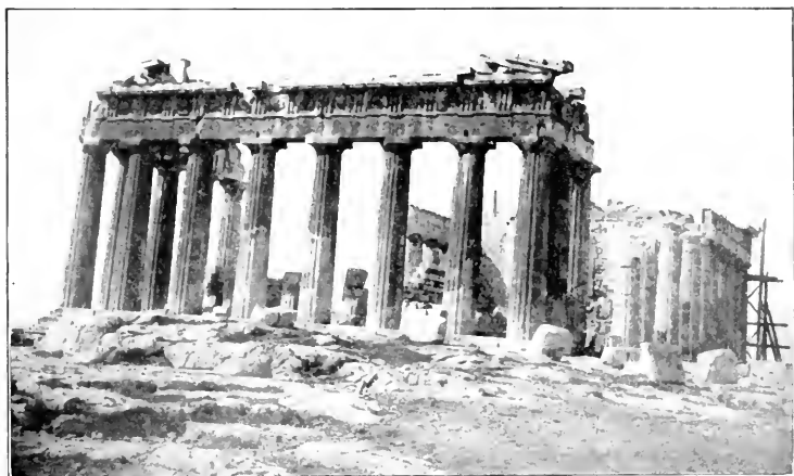
FIG. 277. PARTHENON, ATHENS, FROM THE EAST.
