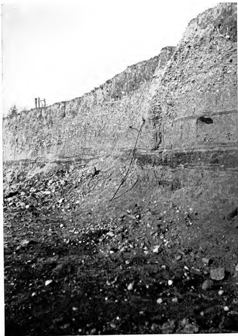
"RAILROAD CUT," LOOKING NORTHWEST, DECEMBER 1, 1899 SHOWING WHERE HUMAN FEMUR WAS FOUND
