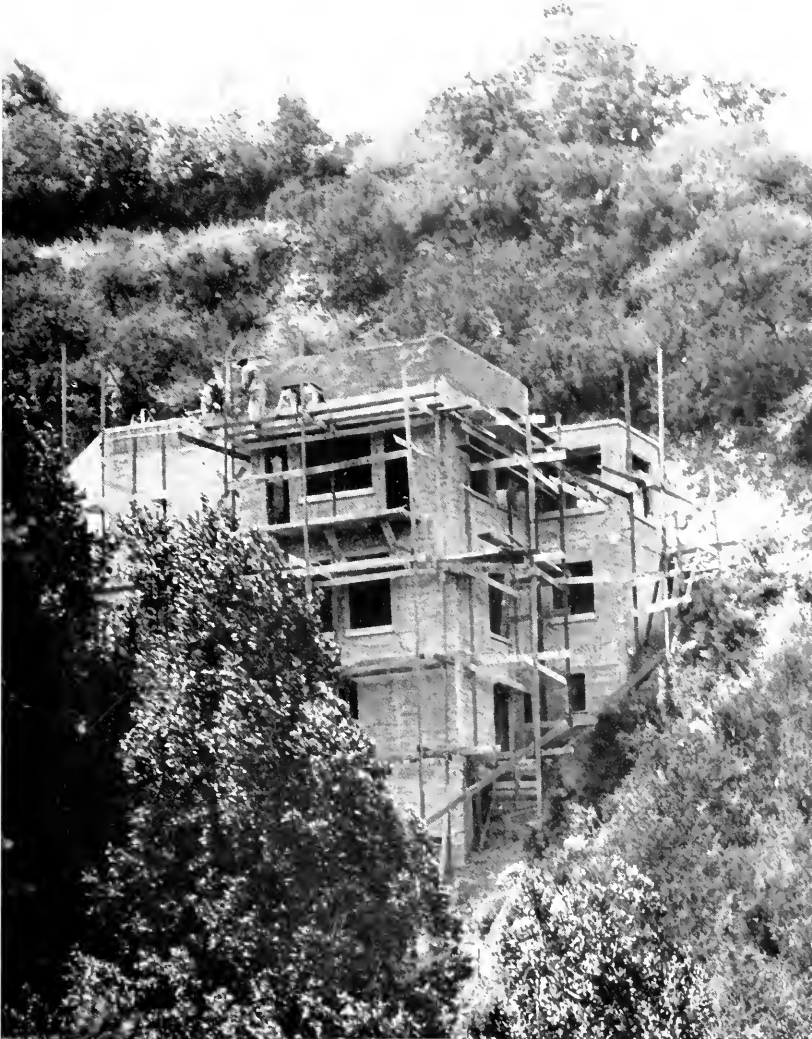
"VILLA MARENGO," LOS GATOS, CALIFORNIA UNDER CONSTRUCTION, SEPTEMBER, 1929
