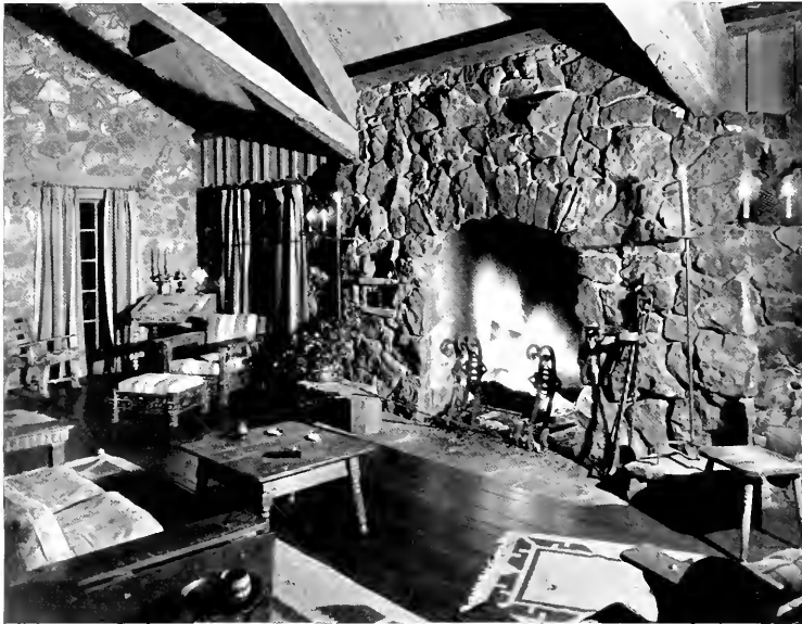
DETAIL OF FIREPLACE, HOUSE OF MRS. LAURA B. WESTPHAL, LAKE TAHOE Kent and Hass, Architects
