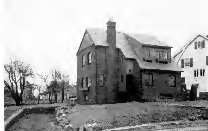
General View of the completed dwelling
