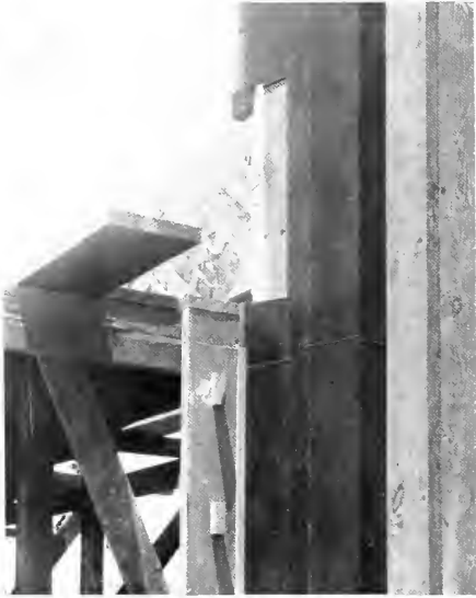
FORMS PARTIALLY LINED WITH FIBRE BOARD
