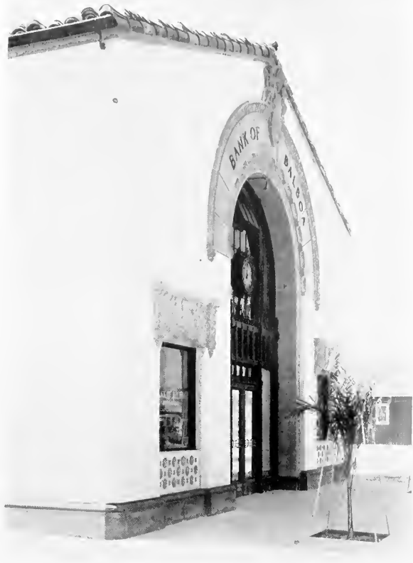
An early example of exposed concrete, employing plaster molds and ordinary board forms. BANK OF BALBOA, BALBOA, CALIFORNIA McGraw, Walls & Clements, Architects, Los Angeles.
