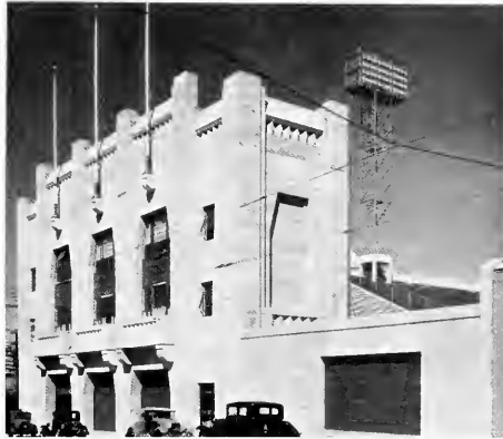
MAIN ENTRANCE AND OFFICE WING Note light tower on right with 48 reflectors
