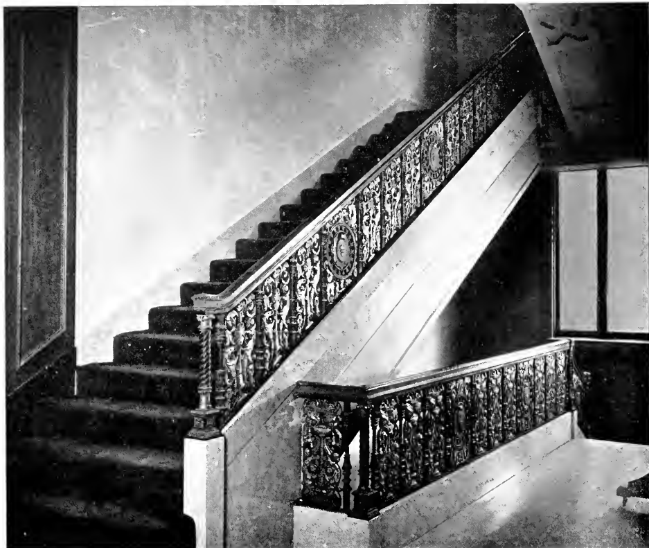
CAST IRON RAIL, MAIN STAIRCASE, SIR FRANCIS DRAKE HOTEL, SAN FRANCISCO Weeks and Day, Architects
