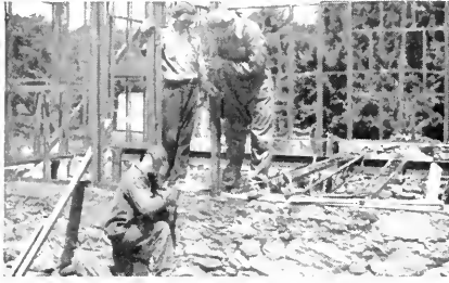
Welder at work making joint at foundations
