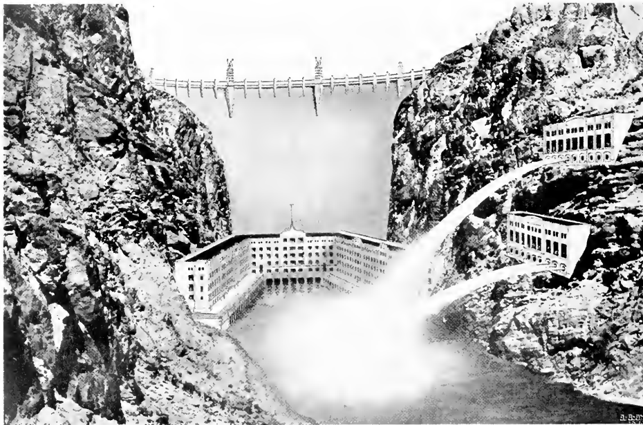
HOOVER DAM, POWER PLANT AND ARIZONA OUTLET WORKS, BOULDER CANYON PROJECT
