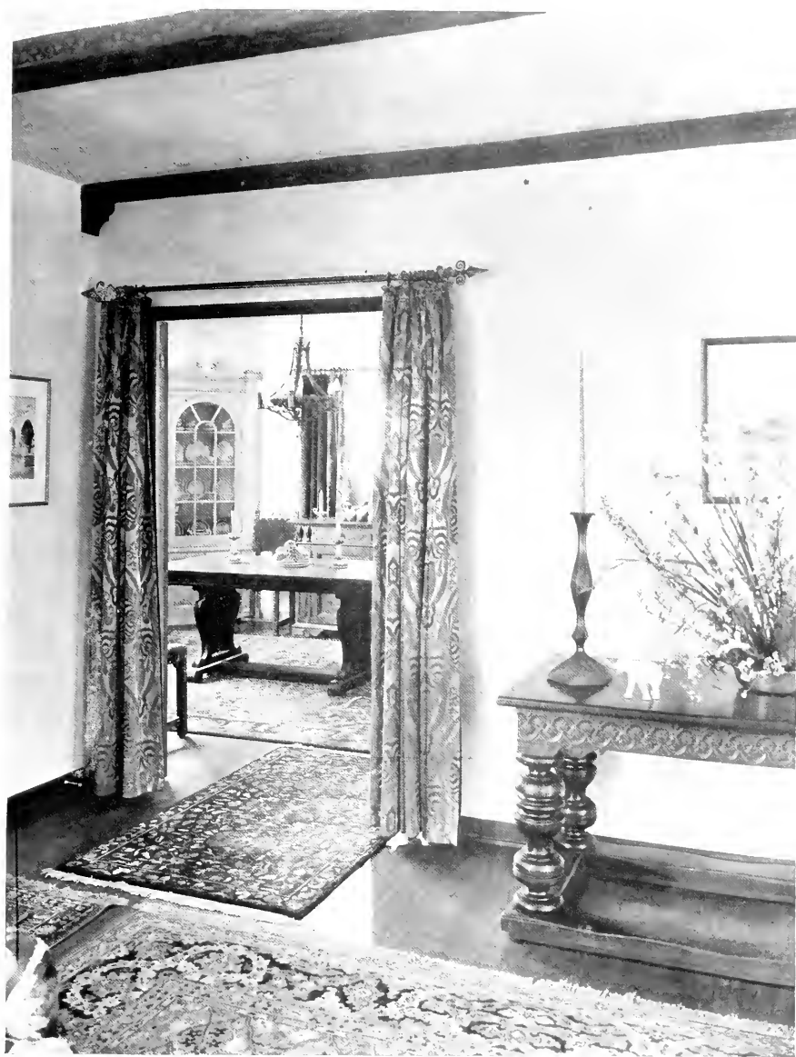
INTERIOR, BEACH HOME OF JOSEPH M. MASTEN, LA JOLLA, CALIFORNIA J. KENDALL MASTEN, ARCHITECT; MARTIN H. SHELDON, ASSOCIATED
