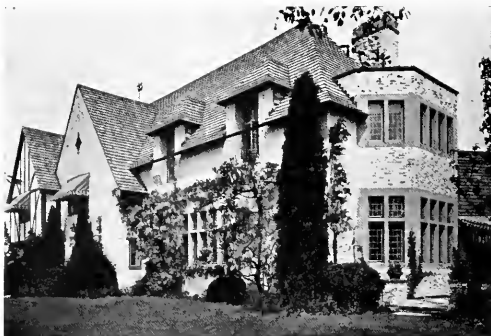
This beautiful Portland, Oregon, house is covered with Cabot's Hand Split Shakes stained with Cabot's Creosote Shingle and Wood Stains. The blended colors in grays and gray-greens harmonize perfectly with the brickwork which has been finished with Cabot's Old Virginia White.
