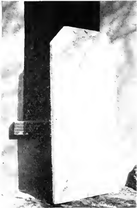
Fabricrete door to store room, 2'-0" x 3'-6" x 3 1/2". Furnace room doors 3' x 7' have been made in the same way, with a special stucco properly reinforced.
