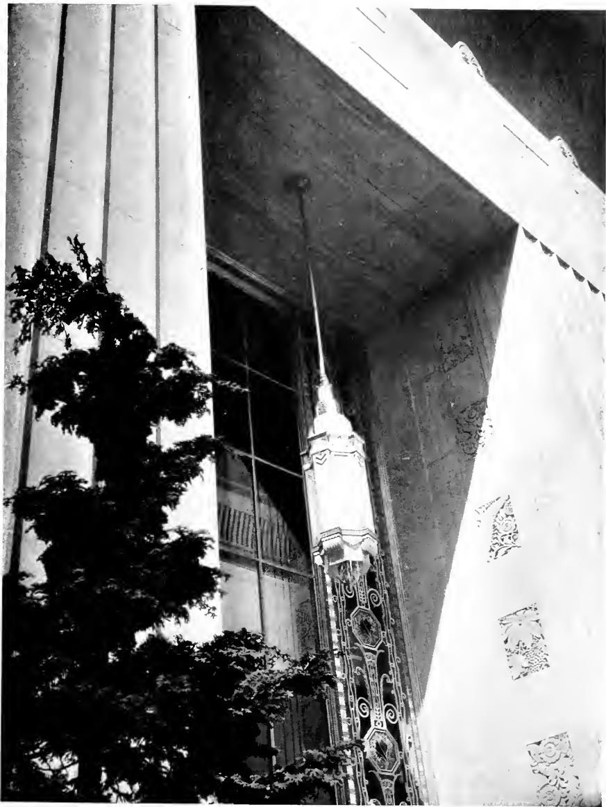
DETAIL OF ENTRANCE, SEATTLE TIMES BUILDING, SEATTLE R. C. REAMER, ARCHITECT
