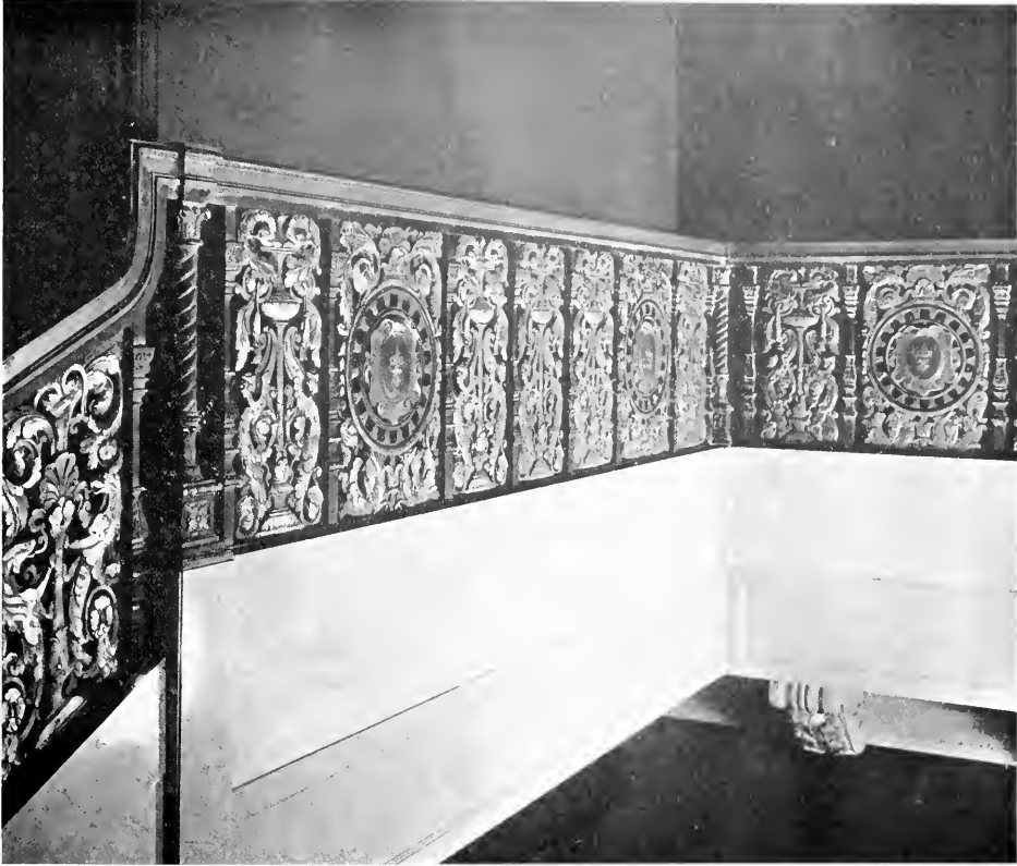
DETAIL OF ORNAMENTAL IRON STAIRCASE, SIR FRANCIS DRAKE HOTEL, SAN FRANCISCO Weeks and Day, Architects
