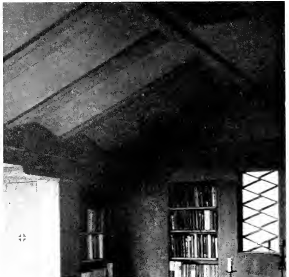
Detail of living room. Ceiling panels of fibre-board, in V form to improve acoustics. Rafters and girders of concrete (Method C). Book cases recessed in wall-hollows. Leaded sash plastered in without frame. Pivoted Fabricrete door with perforated tile as handle. General illumination of room is through ceiling panels consisting of stucco grilles glazed with flat Philippine shell.
