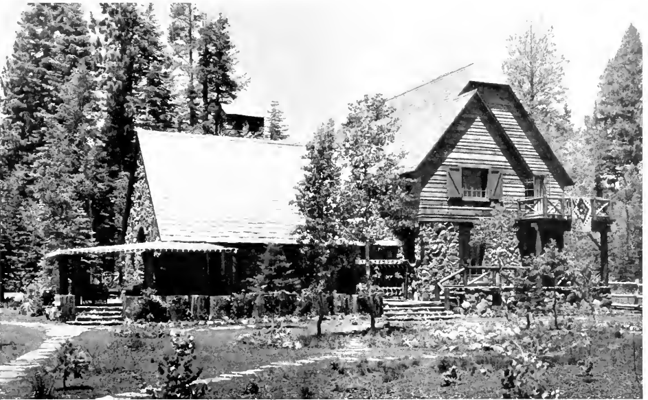
LAKE FRONT, HOUSE OF MRS. LAURA B. WESTPHAL, LAKE TAHOE Kent and Hass, Architects
