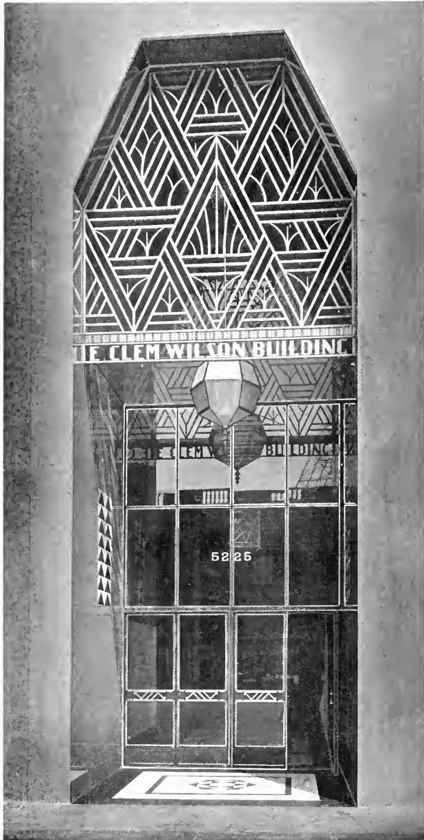
MAIN ENTRANCE. E. CLEM WILSON BUILDING. LOS ANGELES MEYER AND HOLLER, INC., DESIGNERS AND BUILDERS
