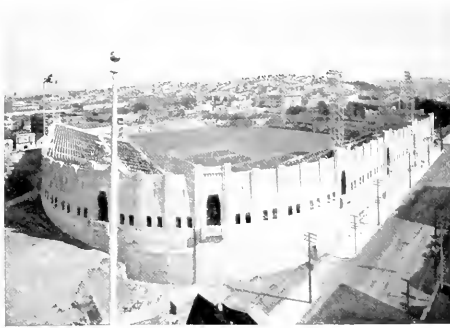
GENERAL VIEW OF STADIUM FROM OUTSIDE
