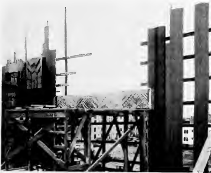
PLASTER WASTE-MOLD SET IN PLACE
