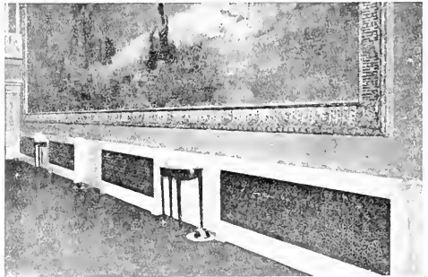
Installation of Wickwire-Spencer Grilles, Metropolitan Theater, Brooklyn, N. Y.
