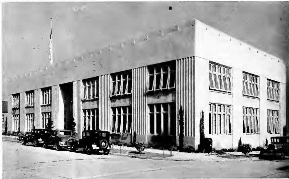
OFFICE WING, SEATTLE TIMES BUILDING, SEATTLE, WASHINGTON
