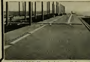
STEELEX Floor Lath is unrolled over the joists. The illustration above shows STEELEX Floor Lath in an unbroken stretch of 212'.
