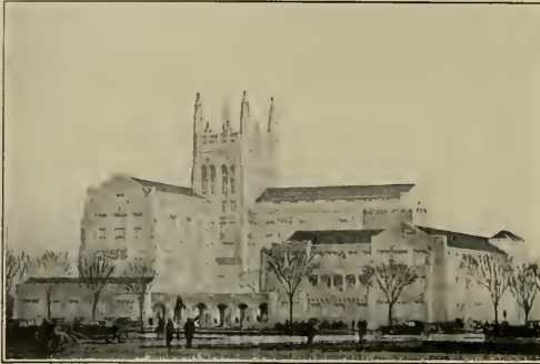
The Chicago Lying-in Hospital and Dispensary. Architects: Schmidt, Gordon and Erikson. General Contractor: H. B. Barnard. Electrical Contractor: Lab Electric Company.
