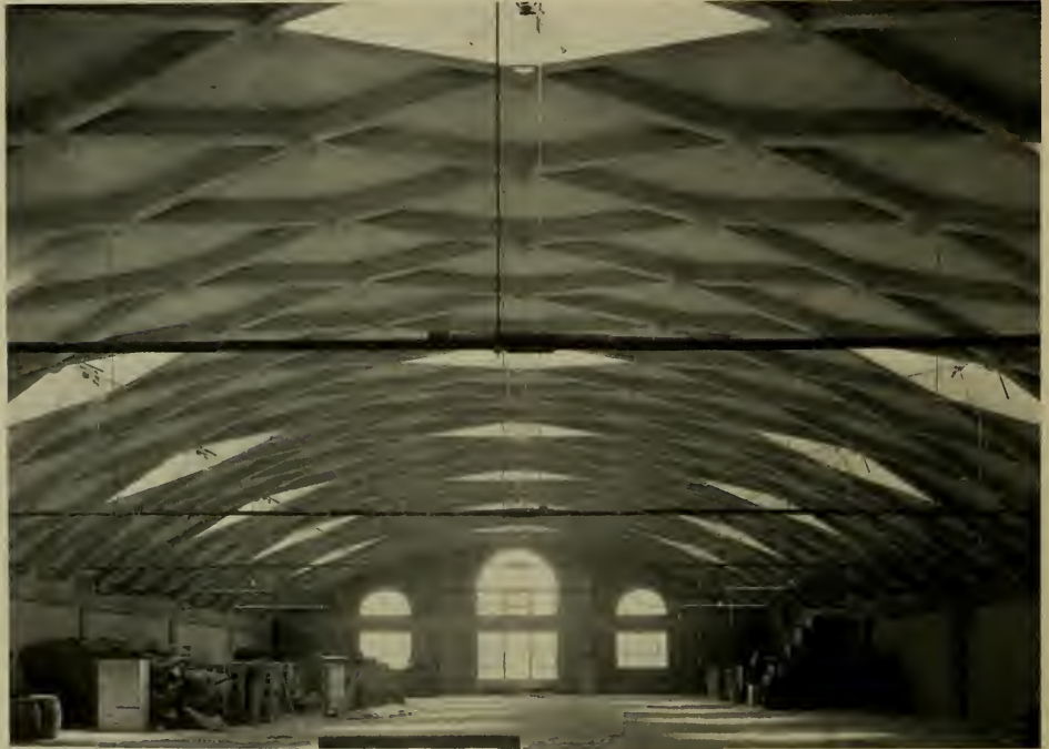
GENERAL VIEW OF INTERIOR, COCO COLA PLANT, LOS ANGELES, SHOWING ROOF CONSTRUCTION IN COMPLETED STATE
