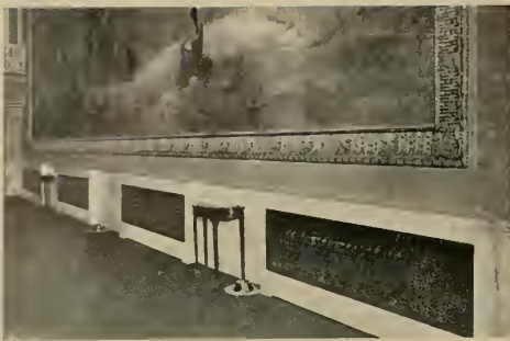
Installation of Wickwire-Spencer Grilles, Metropolitan Theater, Brooklyn, N. Y.
