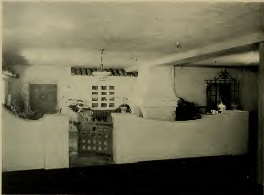
ENTRANCE TO BUNGALOW, BREINER BUILDING, OAKLAND, CALIFORNIA Albert F. Roller, Architect
