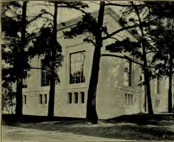
BUILDING FOR HOUSING HEATING EQUIPMENT UNIVERSITY OF CALIFORNIA, BERKELEY George W. Kelham, Architect
