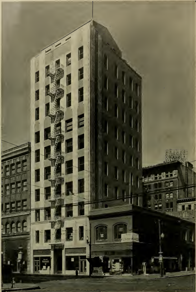
F. R. Siegrist, General Contractor
