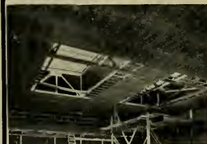
Ribbed STEELEX Lath for plaster is used for school ceilings, either nailed to wood joists or screw-tied to steel joists or suspended ceilings.
