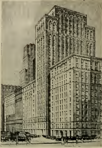
Another Lindgren & Swinerton, Inc. Contract Completed 22 STORY MILLS TOWER, SAN FRANCISCO LEWIS P. HOBART, Architect
