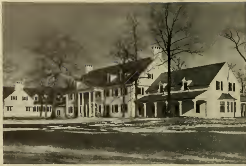
Milwaukee Country Club, Milwaukee, Wis. Architects: Fitzhugh Scott and Roger H. Ballard, Milwaukee. Walls, brick and woodwork finished with Cabot's DOUBLE-WHITE Collopakes
