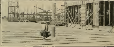
Above: Sisalkraft being used for curing and protecting concrete in the Rigler School, Portland, Ore. Architect, George Jones, Contractor, Ross B. Hammond. Cement Finisher, V. C. McCormick.
