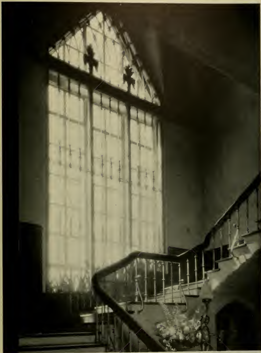
GRAND STAIRCASE, HOUSE OF E. J. SWEETLAND, PIEDMONT, CALIFORNIA FREDERICK H. REIMERS, ARCHITECT
