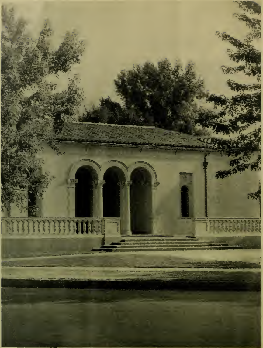
OAKDALE ELEMENTARY SCHOOL, CHICO, CALIFORNIA CHESTER COLE, ARCHITECT; LOUIS L. BROUCHOUD
