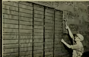
Ribbed STEELEX Lath for plaster and STEELEX Channels form a practical and modern method of constructing school partitions.
