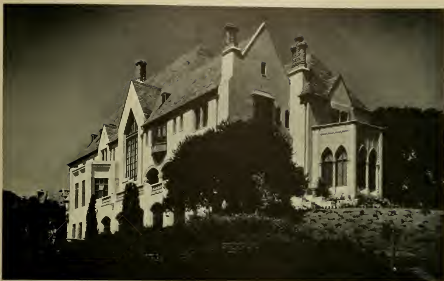
HOUSE OF E. J. SWEETLAND, PIEDMONT, CALIFORNIA Frederick H. Reimers, Architect
