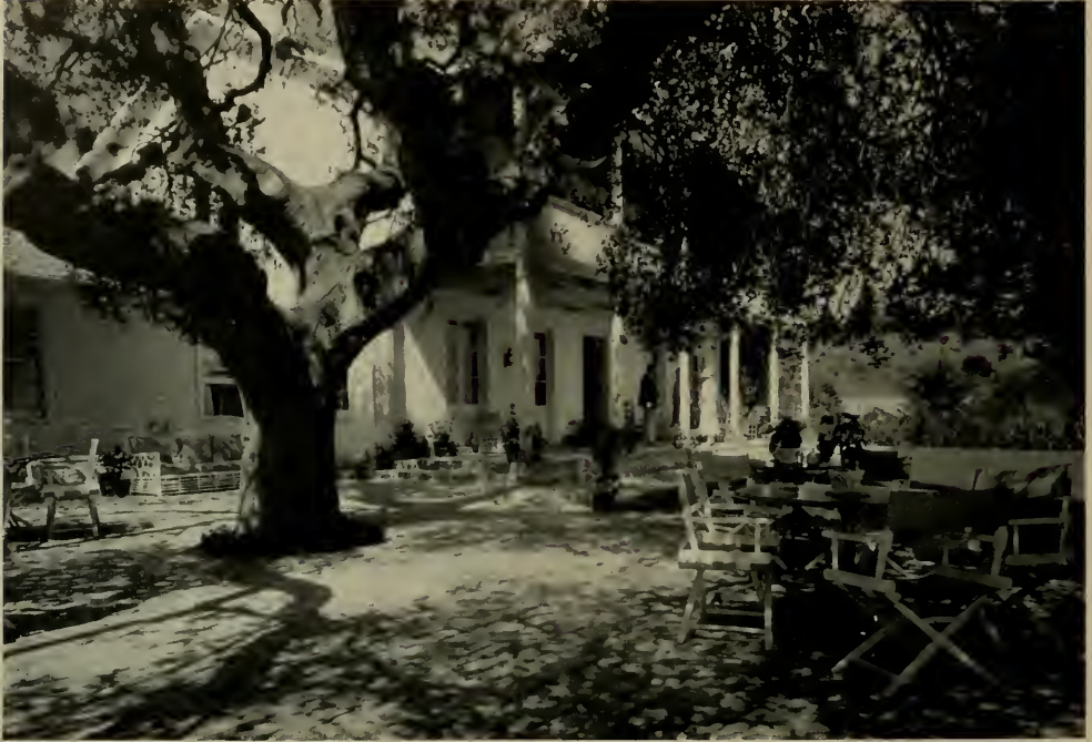
GUEST HOUSE OF PASATIEMPO CLUB, SANTA CRUZ, CALIFORNIA Clarence A. Tantau, Architect
