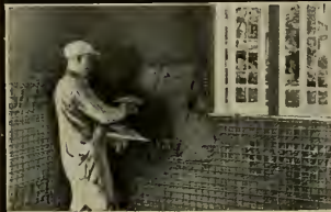
As the plaster is applied against the fibrous backing of Ribbed STEELEX Lath, the copper-bearing steel wire network becomes automatically embedded in the plaster.
