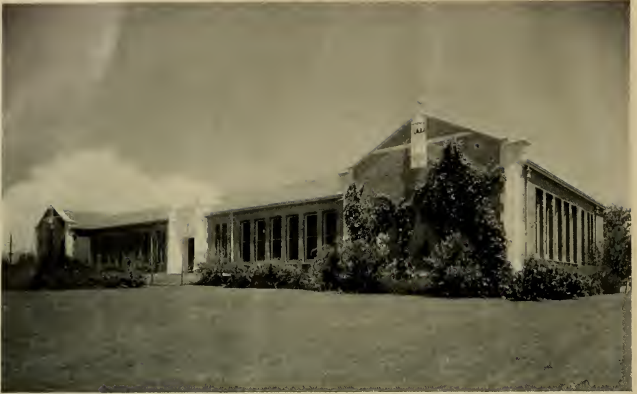
SCHOOL BUILDING, OROVILLE, CALIFORNIA Chester Cole, Architect; Louis L. Brouchoud
