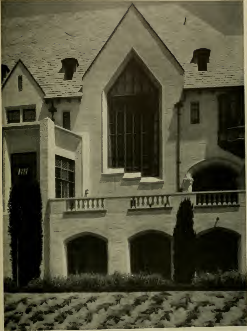
DETAIL, HOUSE OF E. J. SWEETLAND, PIEDMONT, CALIFORNIA FREDERICK H. REIMERS, ARCHITECT
