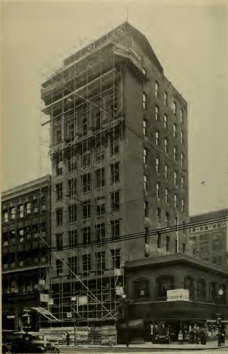
Steel Scaffolding by Patent Scaffolding Company
