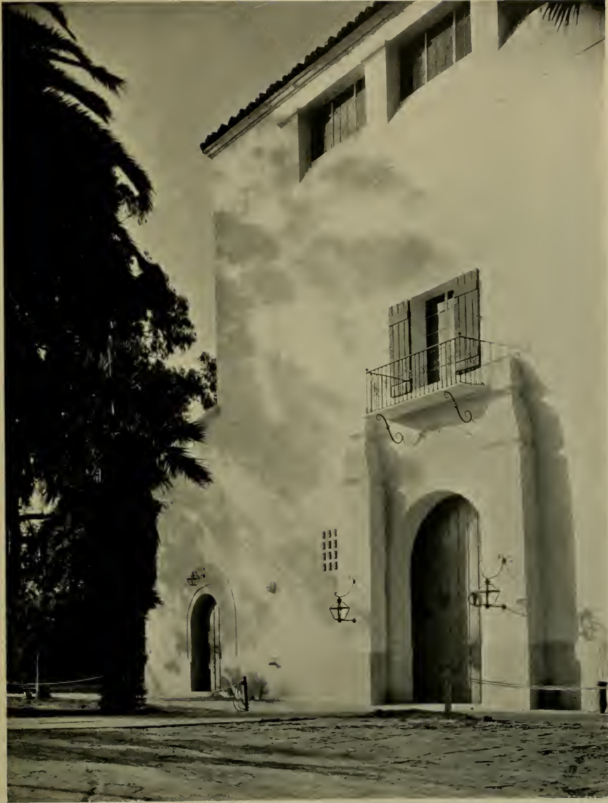
STAGE ENTRANCE, FOX ARLINGTON THEATER, SANTA BARBARA, CALIFORNIA WILLIAM A. EDWARDS, ARCHITECT; J. J. PLUNKETT
