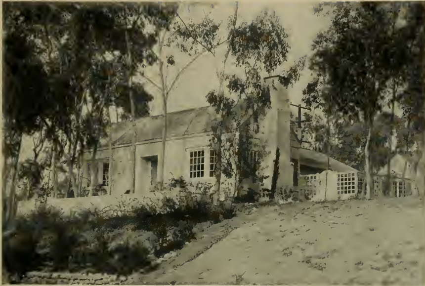
Courtesy Southwest Builder and Contractor
