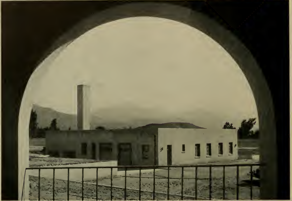
GAS FIRED BOILER PLANT, ST. BERNARDINE HOSPITAL I. E. Loveless, Architect and Engineer
