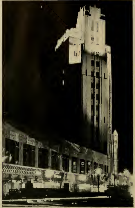
PELESSIER BUILDING, LOS ANGELES Seventy-three General Electric flood lights create the effect
