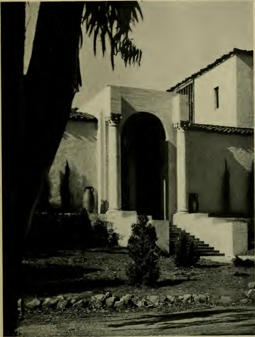
ENTRANCE, EBBETT HALL OF DOMESTIC SCIENCE, STATE TEACHERS COLLEGE, SANTA BARBARA GEORGE B. McDOUGALL, STATE ARCHITECT
