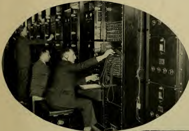
Room 615 in the Waldorf-Astoria, where programs are switched from radio to public rooms to phonographs, and the quality of reproduction is supervised
