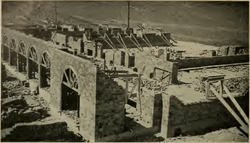
BOULDER CITY, NEVADA General view of a dormitory building under construction.
