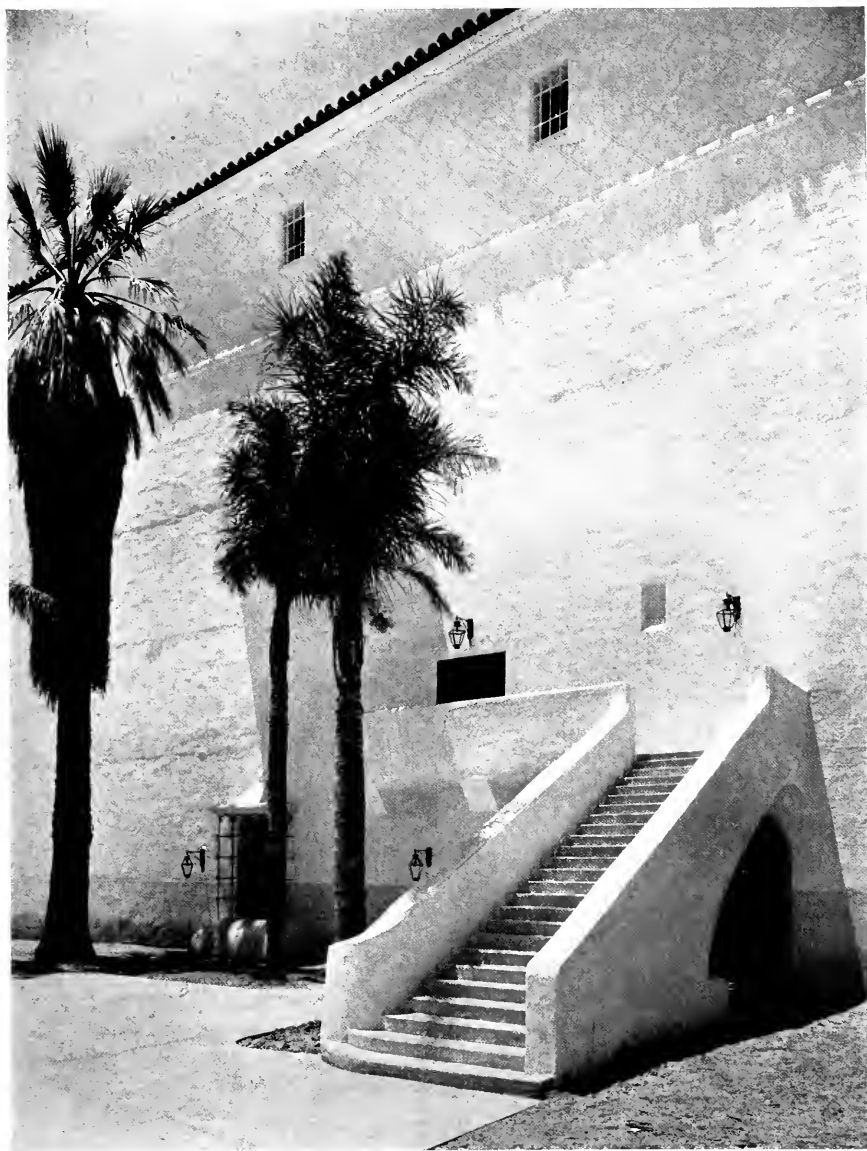
FOX ARLINGTON THEATER. SANTA BARBARA, CALIFORNIA WILLIAM A. EDWARDS, ARCHITECT; J. J. PLUNKETT
