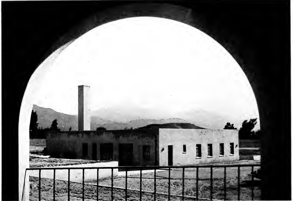
GAS FIRED BOILER PLANT, ST. BERNARDINE HOSPITAL I. E. Loveless, Architect and Engineer
