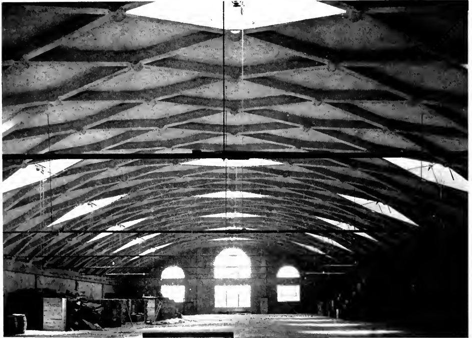
GENERAL VIEW OF INTERIOR, COCO COLA PLANT, LOS ANGELES, SHOWING ROOF CONSTRUCTION IN COMPLETED STATE
