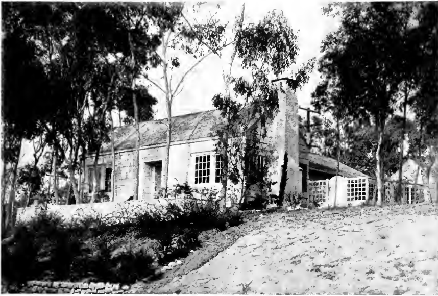
Courtesy Southwest Builder and Contractor
