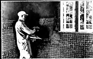
As the plaster is applied against the fibrous backing of Ribbed STEELTEX Lath, the copper-bearing steel wire network becomes automatically embedded in the plaster.
