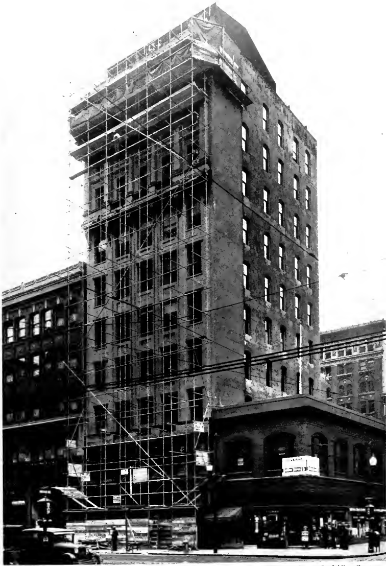
Steel Scaffolding by Patent Scaffolding Company
