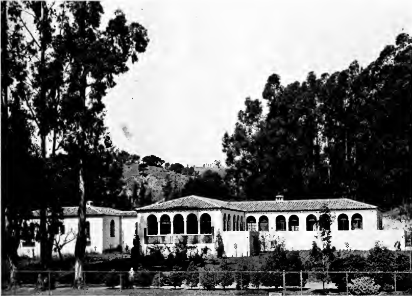
MUSIC BUILDING, MILLS COLLEGE, OAKLAND Walter H. Ratcliff, Architect
