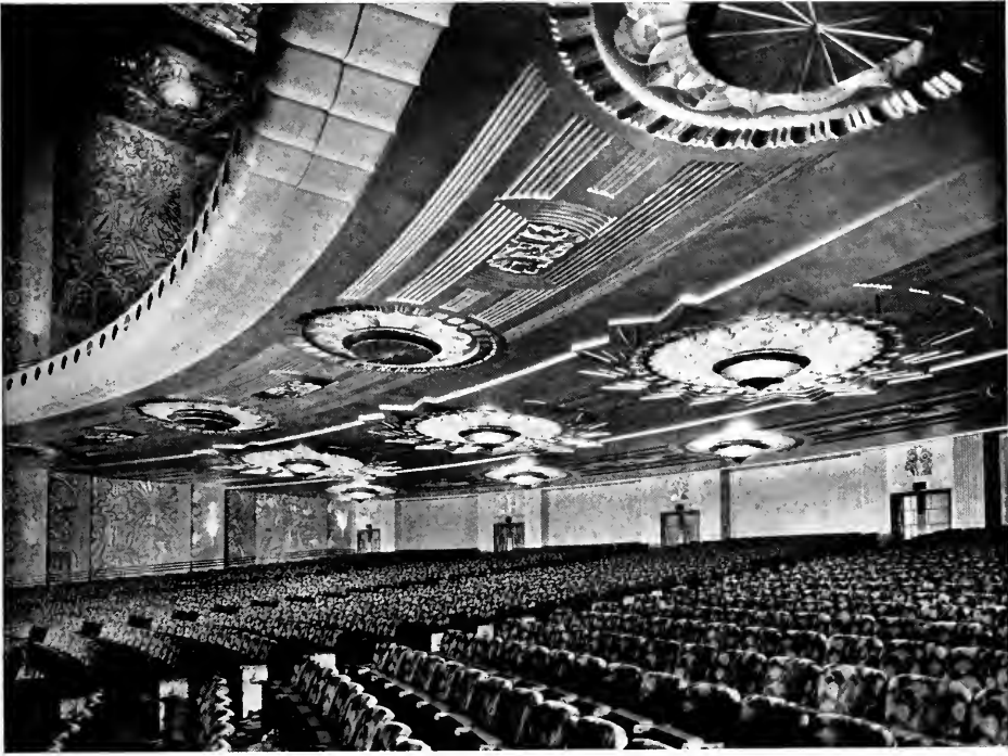
Color scheme same as on walls. Recessed fixtures are of "fin" construction similar to main ceiling.
