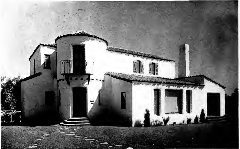
RESIDENCE OF LAURENCE KENNEDY, REDDING, CALIFORNIA Chester Cole, Architect; Louis L. Brouchoud
