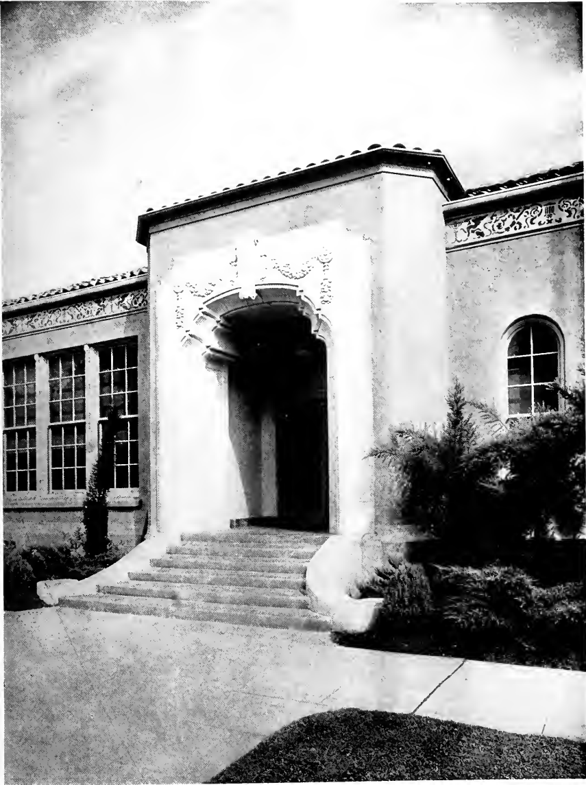
DETAIL OF ENTRANCE, LINDEN SCHOOL, CHICO, CALIFORNIA CHESTER COLE, ARCHITECT; LOUIS L. BROUCHOUD
