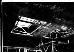
Ribbed STEELTEX Lath for plaster is used for school ceilings, either nailed to wood joists or screw-tied to steel joists or suspended ceilings.
