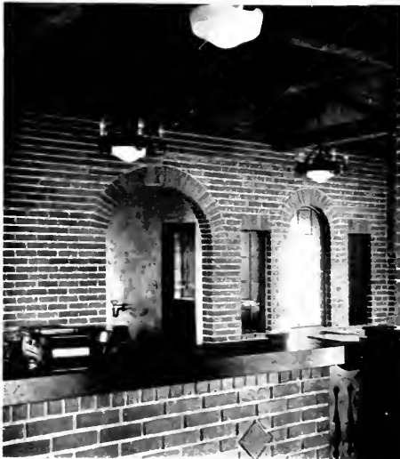
INTERIOR VIEW FROM ENTRANCE LOBBY
