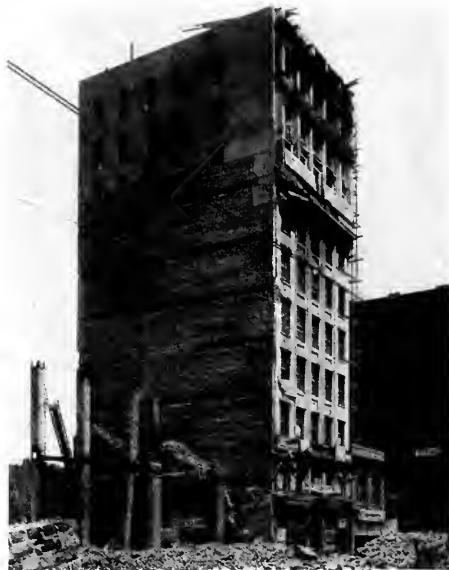
ATLAS BUILDING AFTER THE SAN FRANCISCO EARTHQUAKE AND FIRE
