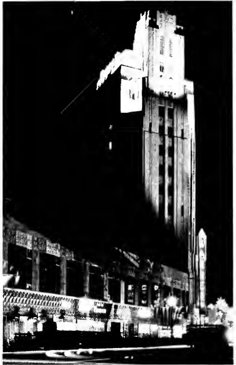
PELLESSIER BUILDING, LOS ANGELES Seventy-three General Electric flood lights create the effect
