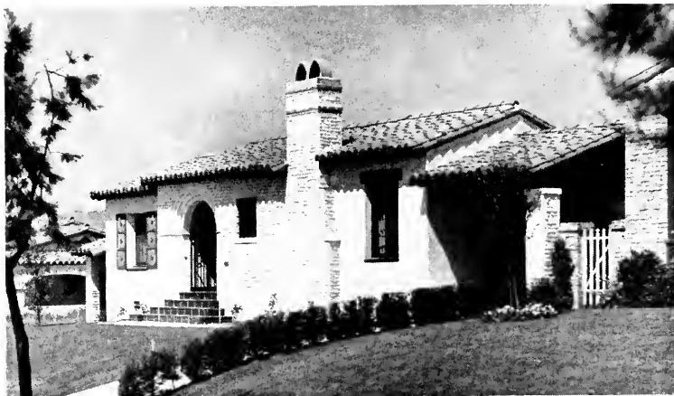
HOUSE OF MR. AND MRS. T. J. PARKER, LOS ANGELES Gable and Wyant, Architects
