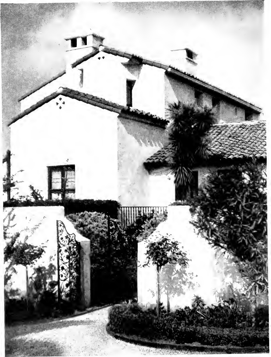
A STUDY IN ROOF LINES
