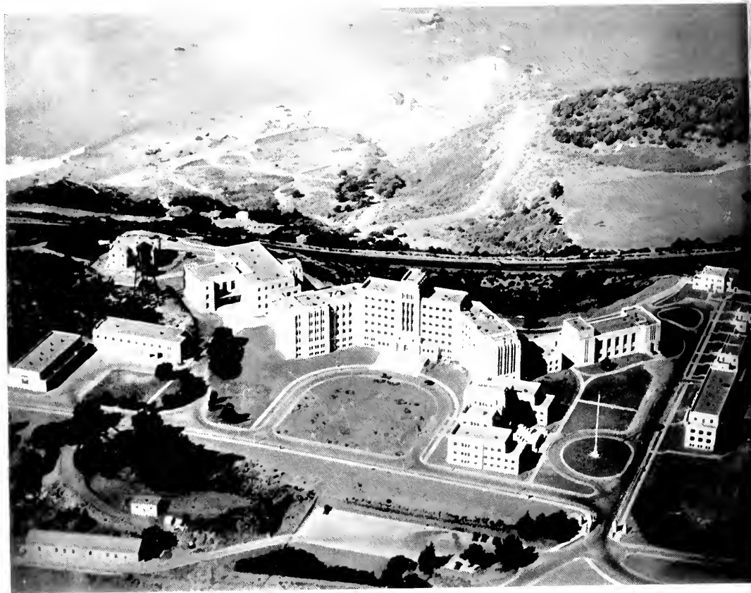
AIRPLANE VIEW, VETERANS ADMINISTRATION FACILITY, FORT MILEY, SAN FRANCISCO, CALIFORNIA
