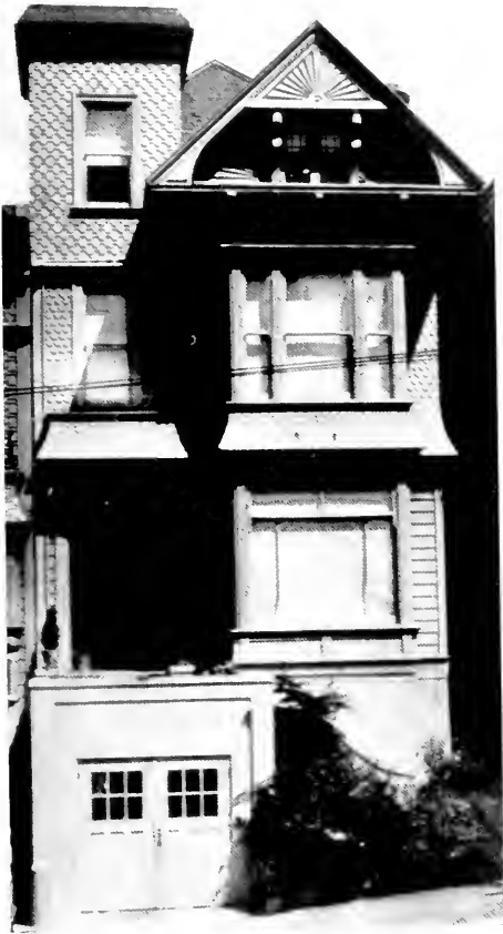
LEFT—HOUSE AT 2618 BUCHANAN STREET, SAN FRANCISCO, BEFORE ALTERATIONS
