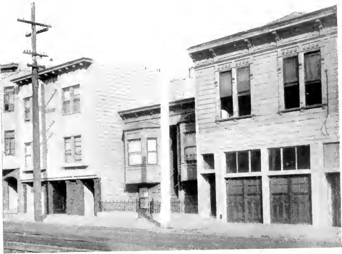
BUILDINGS, NORTH SIDE OF GREENWICH STREET, BETWEEN SCOTT AND PIERCE, SAN FRANCISCO
