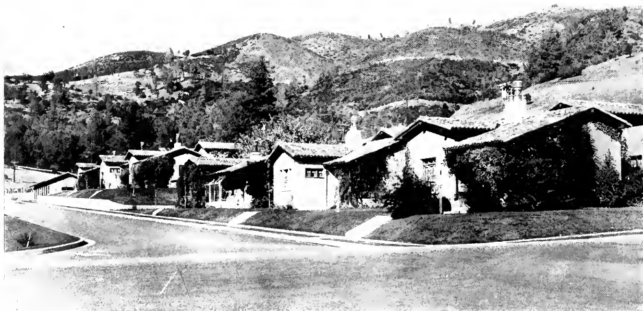
CONCRETE BUNGALOWS FOR POWER HOUSE EMPLOYEES AT MOCCASIN
