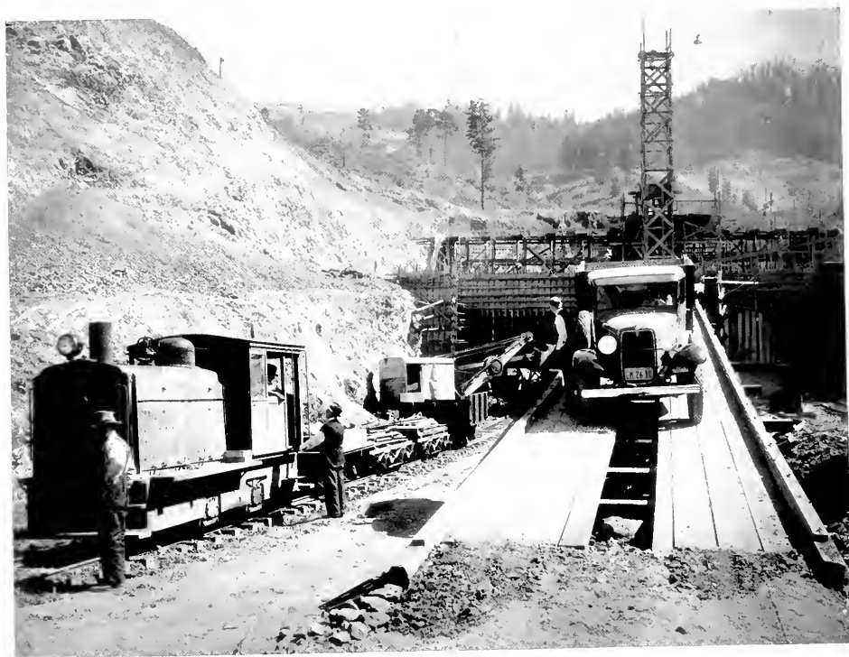
SPEED WORK ON HUGE CONTRA COSTA TUNNEL PROJECT Here is a section of the Broadway low-level tunnel project, near Oakland, California, where a new traffic link between Alameda and Contra Costa Counties is being constructed, with two huge one-way tunnels, each 3,168 feet long
