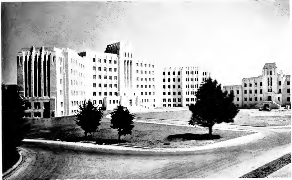
MAIN GROUP OF VETERANS ADMINISTRATION FACILITY, WITH HOSPITAL UNIT (Left) AND ADMINISTRATION BUILDING (Right)
