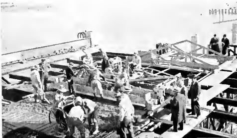
PLACING GRAVELITE CONCRETE IN UPPER DECK OF BRIDGE
