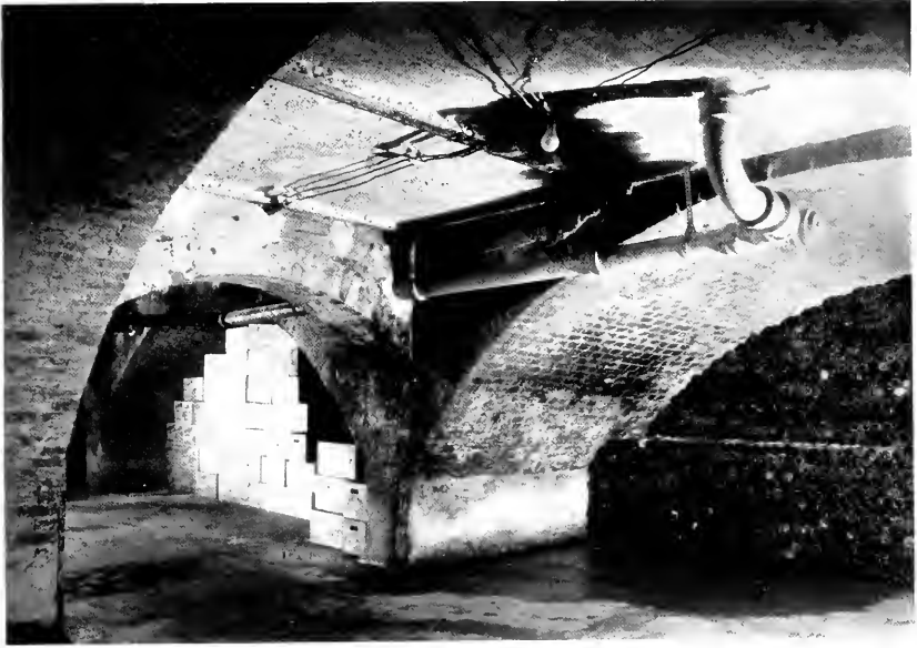
ANOTHER VIEW OF BRICK VAULTS IN BASEMENT OF GLOBE BREWERY, BALTIMORE
