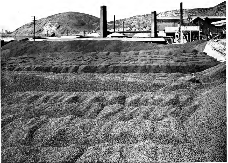
STOCK PILE OF GRAVELITE AT PLANT, POINT RICHMOND, CALIFORNIA This material mixed with cement makes a light weight concrete that is destined to revolutionize the present method of making structural concrete. Engineers say its use on the upper deck of the Bay Bridge will mean a saving of 20,000 tons in dead weight
