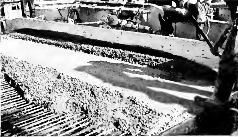
CLOSE-UP, SHOWING VIBRATING SCREEN IN OPERATION AND STEEL REINFORCEMENT
