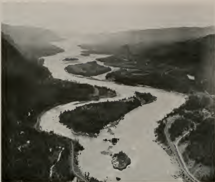
Looking west, downstream, from the Oregon side of the Columbia River, this view shows the site of the Bonneville project before work was started. The river may seem docile, but its volume of water makes this dam construction one of the most difficult ever attempted. (Photograph by Photo-Art Studios)
