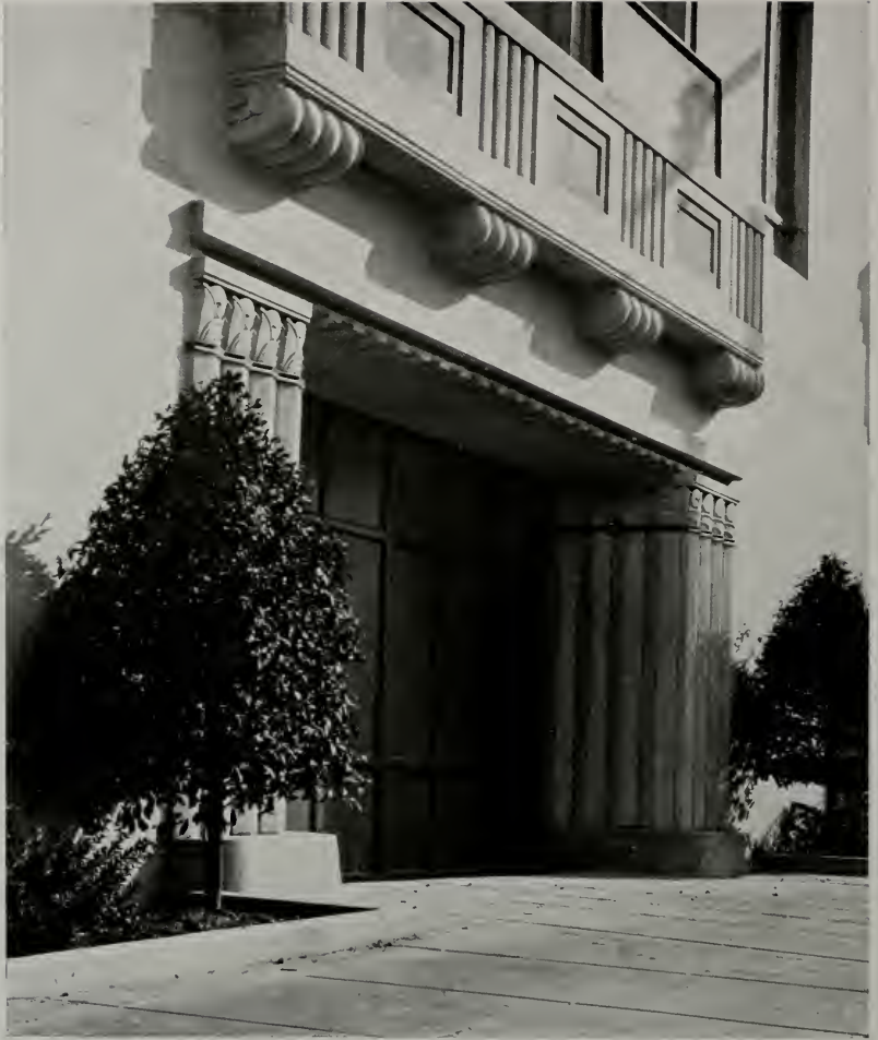
GARAGE ENTRANCE, SUNKIST BUILDING, LOS ANGELES Walker and Eisen, Architects
