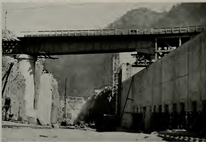
One view of the navigation locks being built between Bradford Island and the Oregon shore of the river. Above is seen the present Union Pacific Railroad right-of-way. The tracks of this line will be relocated, moved higher up the canon slope so big ships may pass where trains now run.
