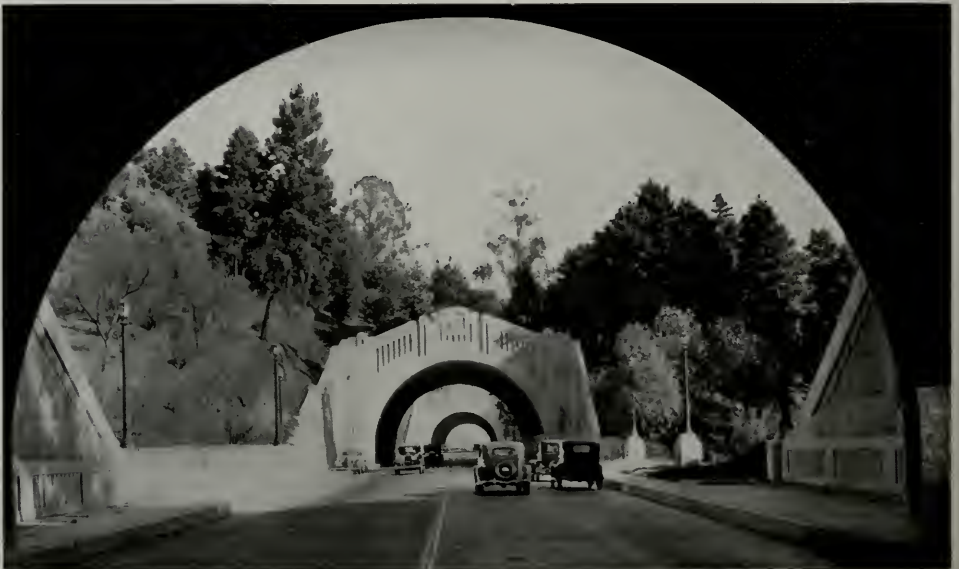
Courtesy California Highways and Public Works
