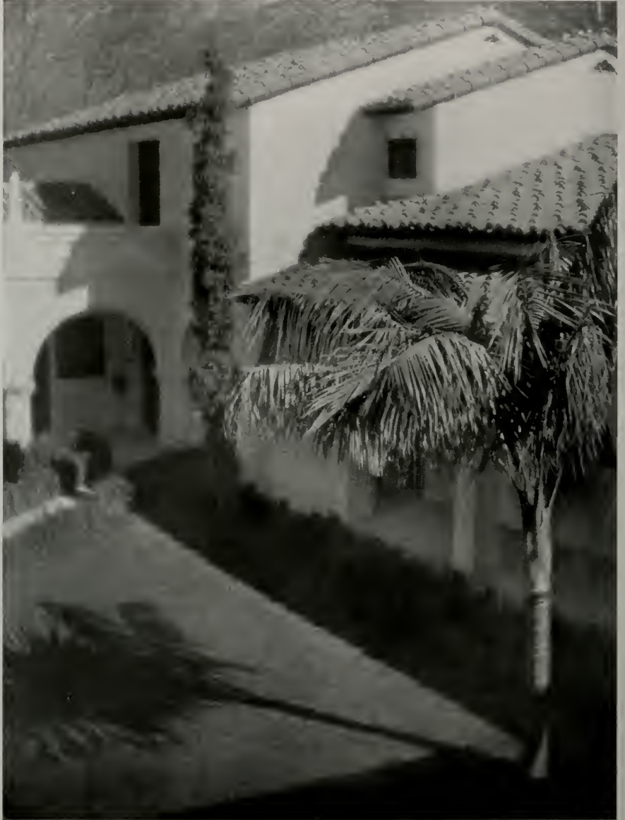
A STUDY IN ROOF LINES
