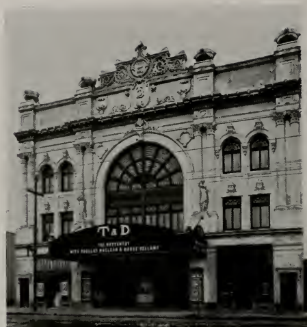
FOX THEATER, RICHMOND, BEFORE ALTERATIONS F. Frederic Amandes, Architect
