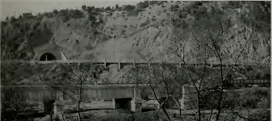
TUNNEL PORTAL AT ELYSIAN PARK AND RIVERSIDE DRIVE, LOS ANGELES, WHERE VIADUCT WILL CONNECT
