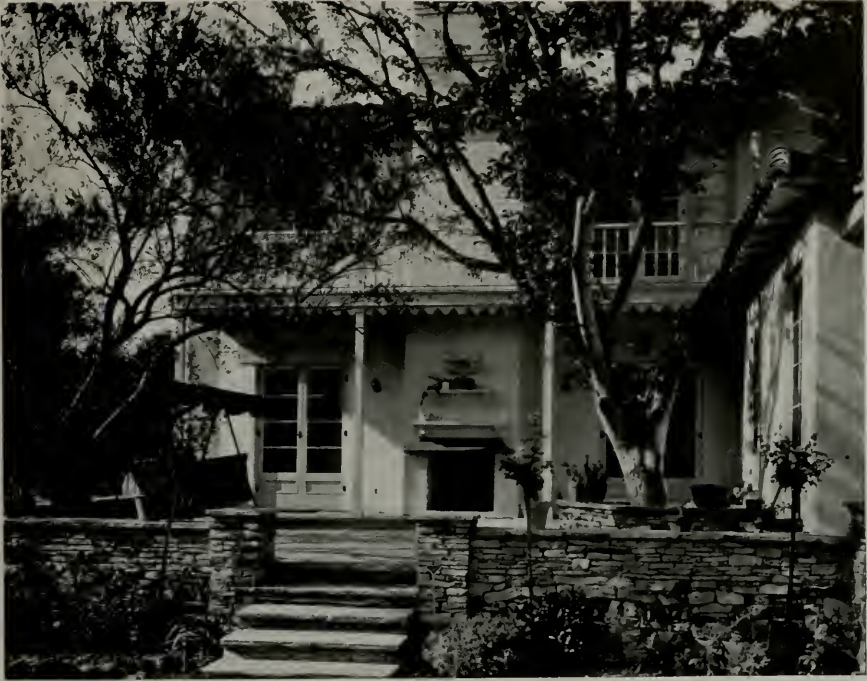
OUTDOOR LIVING ROOM, RESIDENCE FOR E. F. MARSHALL, TOLUCA LAKE, CALIFORNIA Henry Carlton Newton and Robert Dennis Murray, Architects
