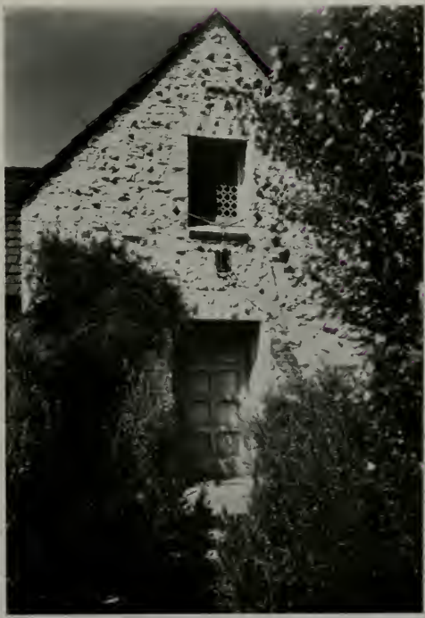
ENTRANCE DETAIL, RESIDENCE FOR CLARK DOWNEY, BRENTWOOD CALIFORNIA Henry Carlton Newton and Robert Dennis Murray, Architects
