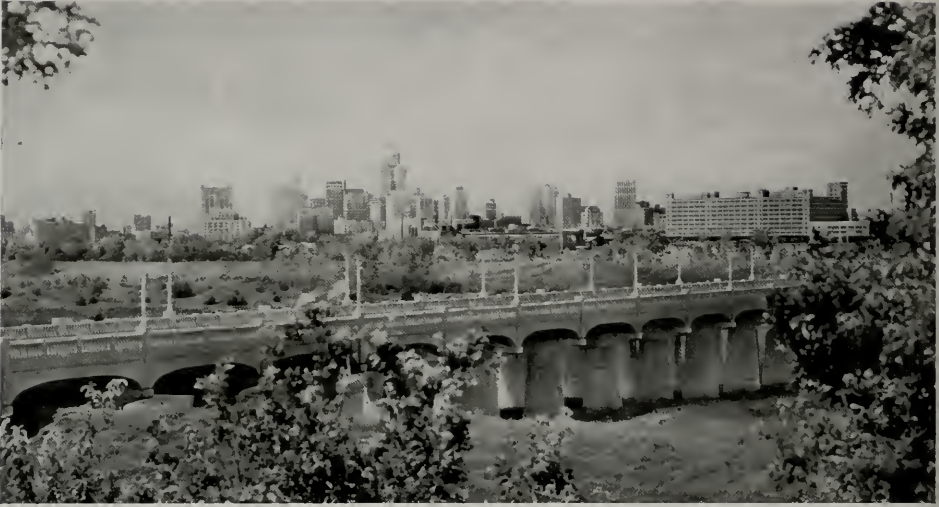
DALLAS SKYLINE FROM WEST CORINTH STREET VIADUCT
