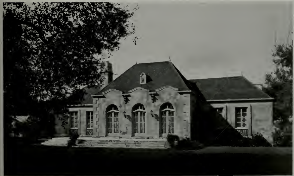
FACADE, RESIDENCE OF MRS. A. BROWN ATHERTON, CALIFORNIA F. Frederic Amandes, Architect
