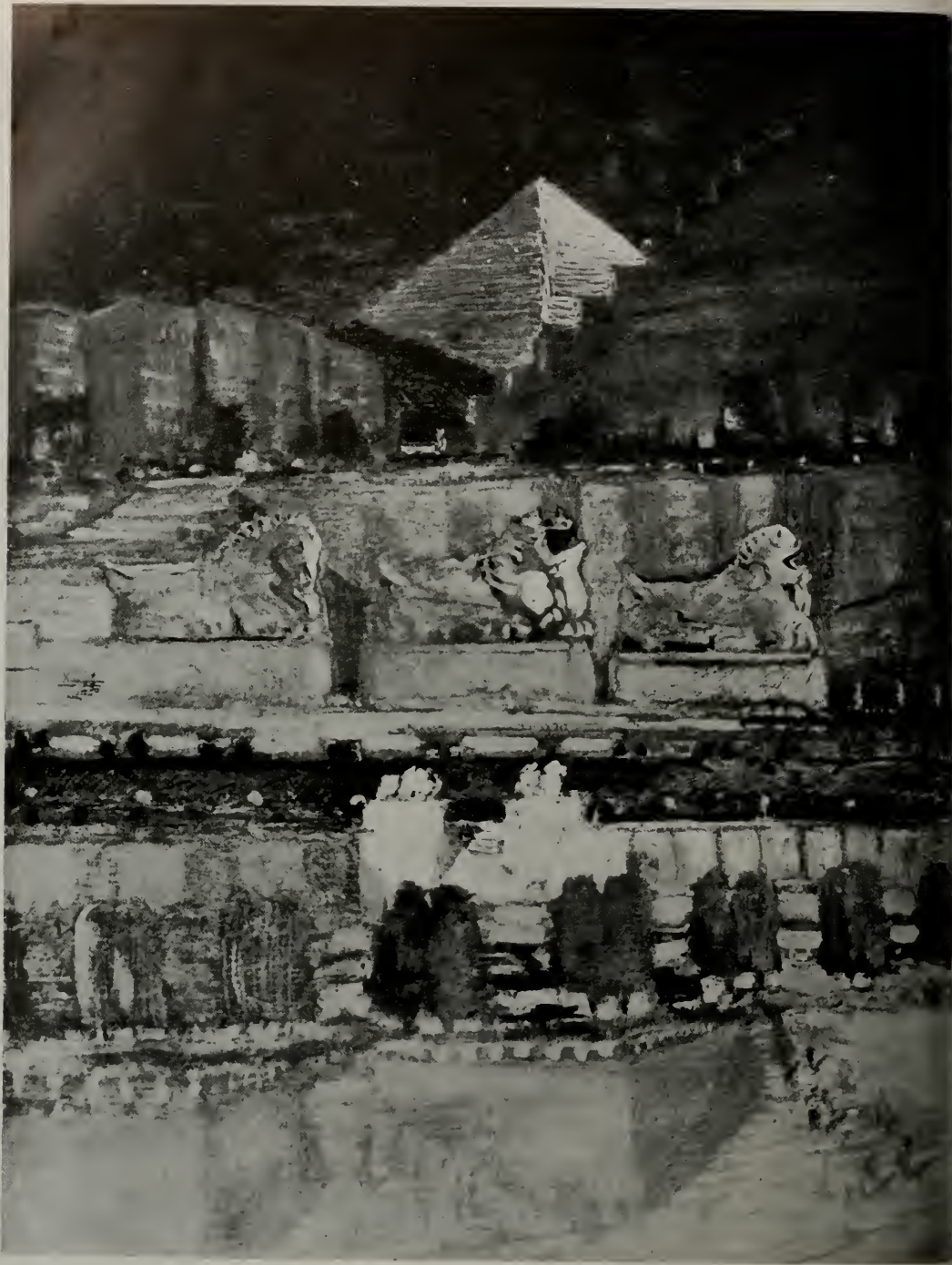
TERRACES AND GARDENS, ADMINISTRATION CENTER LOS ANGELES
