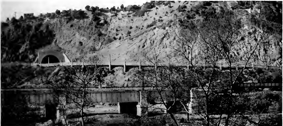
TUNNEL PORTAL AT ELYSIAN PARK AND RIVERSIDE DRIVE, LOS ANGELES, WHERE VIADUCT WILL CONNECT
