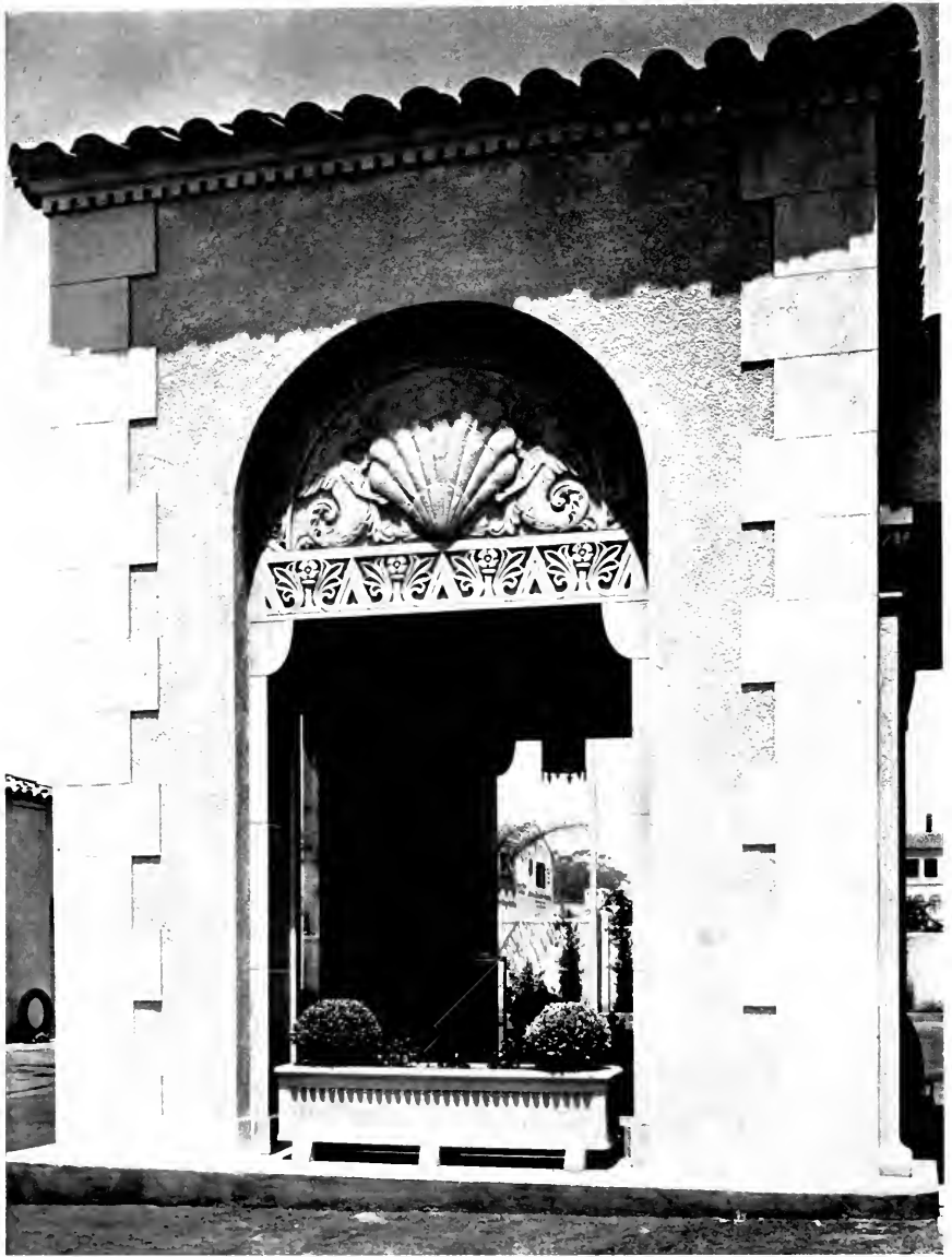
DETAIL OF STATION IN WESTWOOD, LOS ANGELES. DESIGNED TO HARMONIZE WITH ARCHITECTURE OF UNIVERSITY H. O. ALDEN, ARCHITECT
