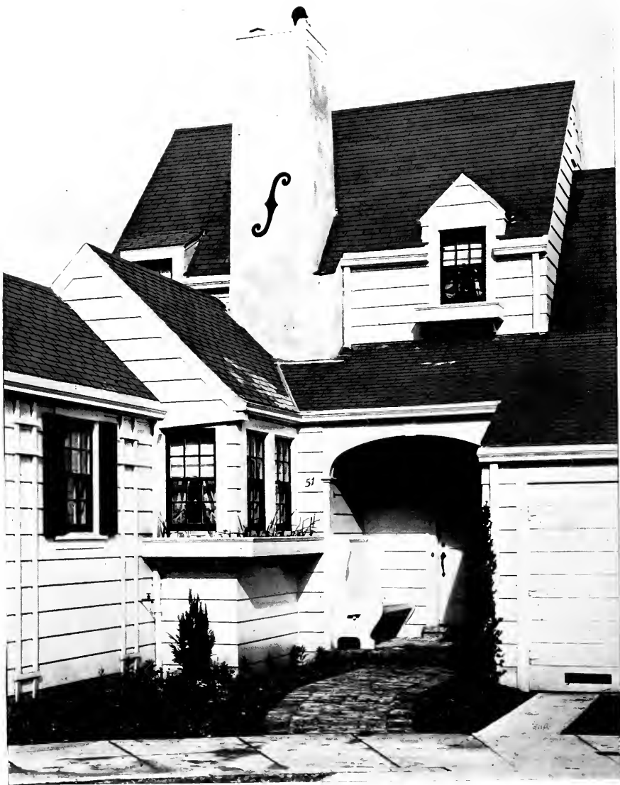
RESIDENCE OF DR. AND MRS. HAMILTON H. ANDERSON, SAN FRANCISCO F. FREDERIC AMANDES, ARCHITECT
