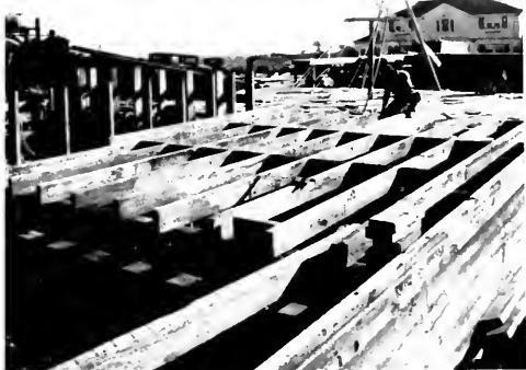
Pressure treated lumber for home of Dr. John L. Pomeroy at Brentwood being placed.
