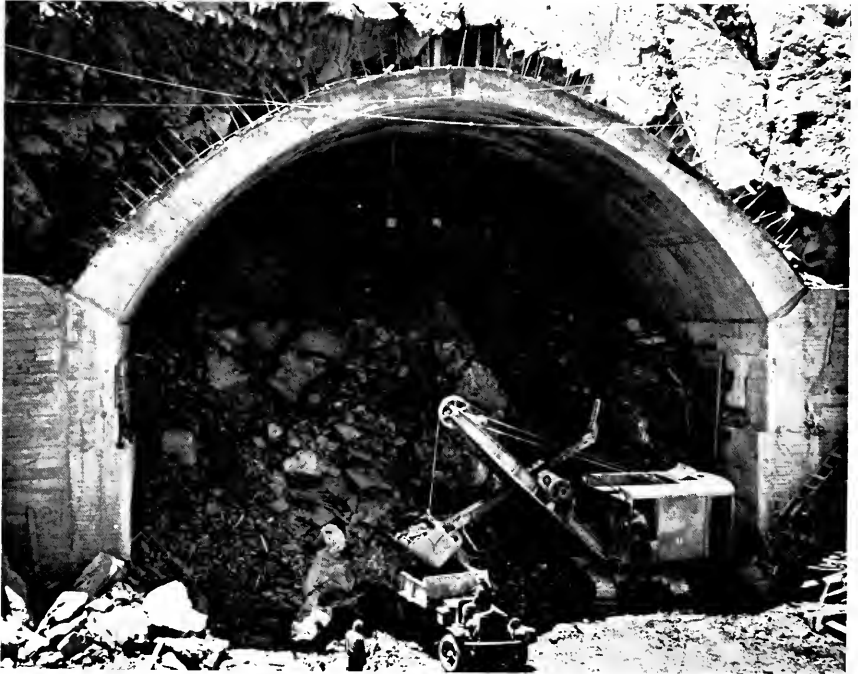
DOWN TO THE CORE. With the tunnel completely concreted and steel lined by novel construction methods, a steam shovel begins removal of thousands of cubic yards of rock from 58 by 76-foot bore. Article on Page 58.
