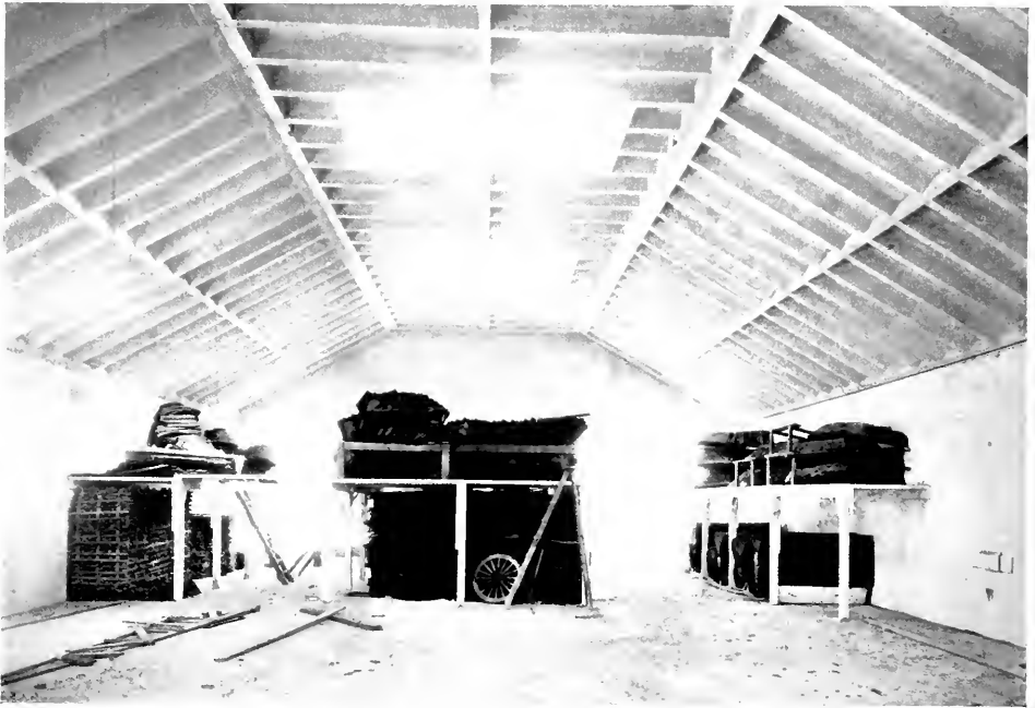
INTERIOR REINFORCED CONCRETE BUILDING FOR STEEL FORM CONTRACTING COMPANY, SAN FRANCISCO, SHOWING NEW TYPE OF ROOF CONSTRUCTION. L. H. Nishkian, C.E.
