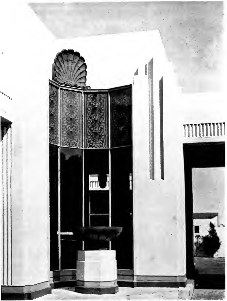
DETAIL OF STATION IN SAN FRANCISCO, SHOWING SHELL MOTIF
