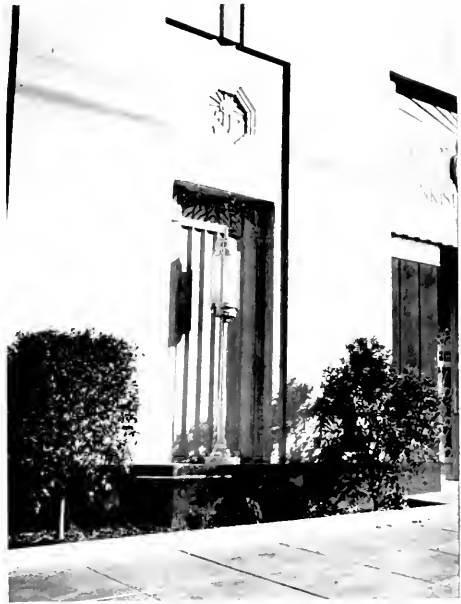
DETAIL OF ELECTROLIER SUNKIST BUILDING
