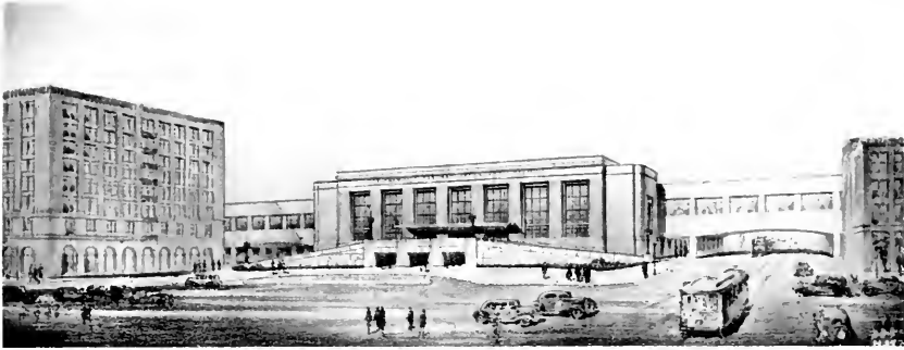
FRONT OF SAN FRANCISCO TERMINAL showing elevated ramp for three tracks of street cars. The building provides a waiting room 135 feet wide by 220 feet long
