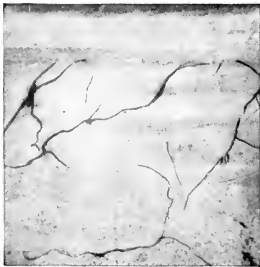
Tan Plastic helps to prevent cracks like these.
