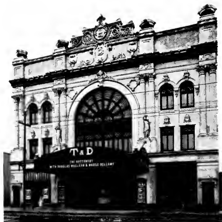
FOX THEATER, RICHMOND, BEFORE ALTERATIONS F. Frederic Amandes, Architect
