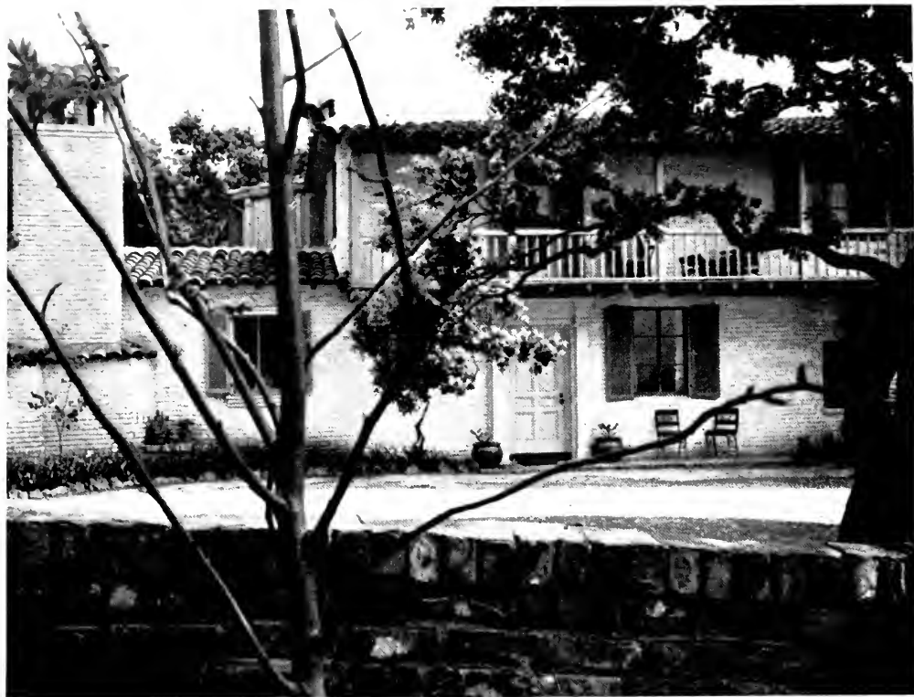
HOUSE FOR DR. T. E. REYNOLDS, PIEDMONT, CALIFORNIA John Knox Ballantine, Jr., Architect
