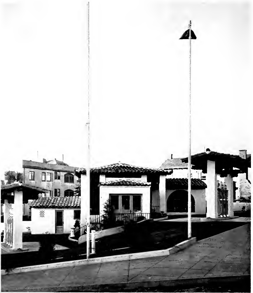
SPANISH TYPE STATION, CLAREMONT DISTRICT, BERKELEY, CALIFORNIA
