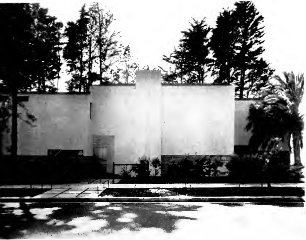
STREET VIEW OF RESIDENCE OF MR. AND MRS. CEDRIC GIBBONS, SANTA MONICA, CALIFORNIA DOUGLAS HONNOLD, ARCHITECT
