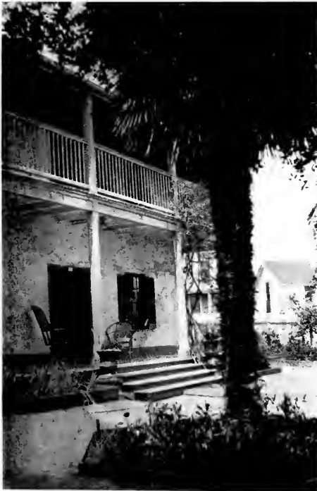
OLD HOUSE IN MONTEREY, CALIFORNIA
