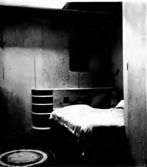
INTERIOR, EDGAR D. TAYLOR STUDIO. MICHAEL GOODMAN, ARCHITECT.
