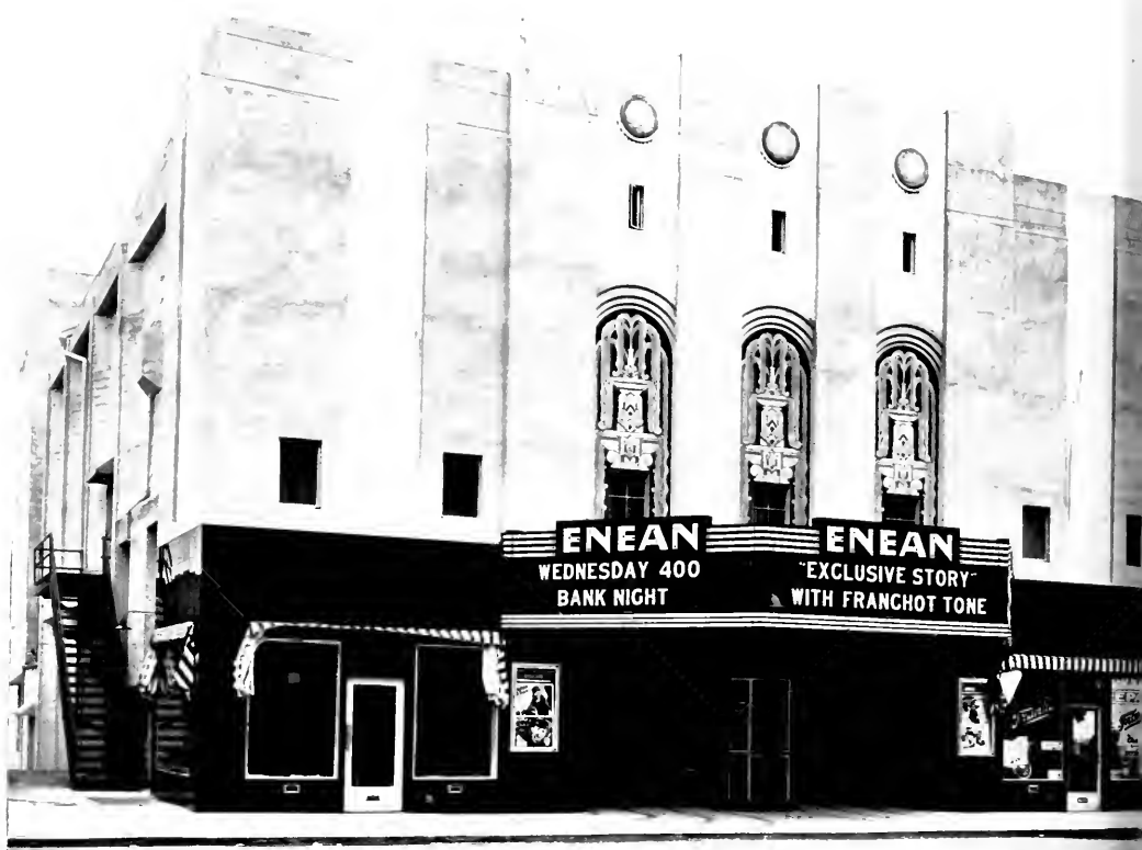
ENEAN THEATER, PITTSBURG, CALIFORNIA F. FREDERIC AMANDES, ARCHITECT
