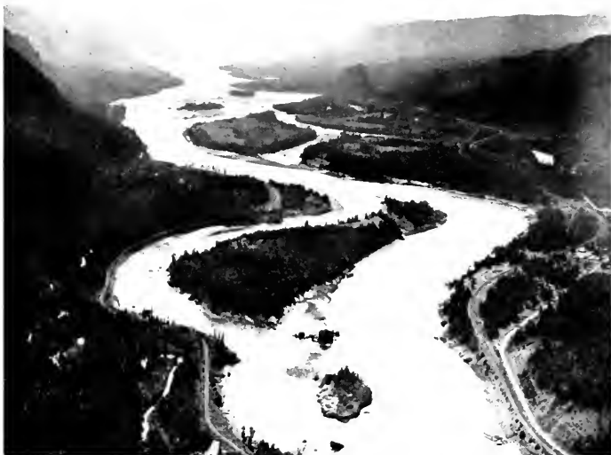
Looking west, down-stream, from the Oregon side of the Columbia River, this view shows the site of the Bonneville project before work was started. The river may seem docile, but its volume of water makes this dam construction one of the most difficult ever attempted. (Photograph by Photo-Art Studios)
