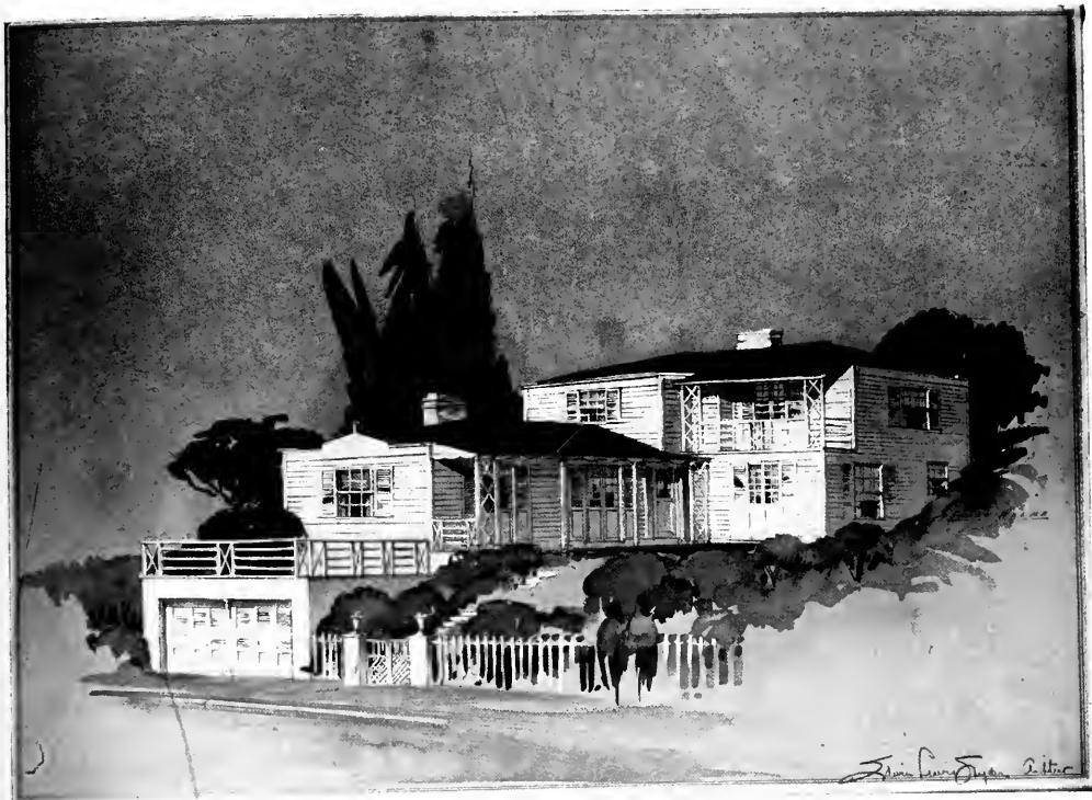
HOUSE FOR GEORGE FREDERICK BRUNS, MORAGA ROAD, OAKLAND, CALIFORNIA EDWIN LEWIS SNYDER, ARCHITECT
