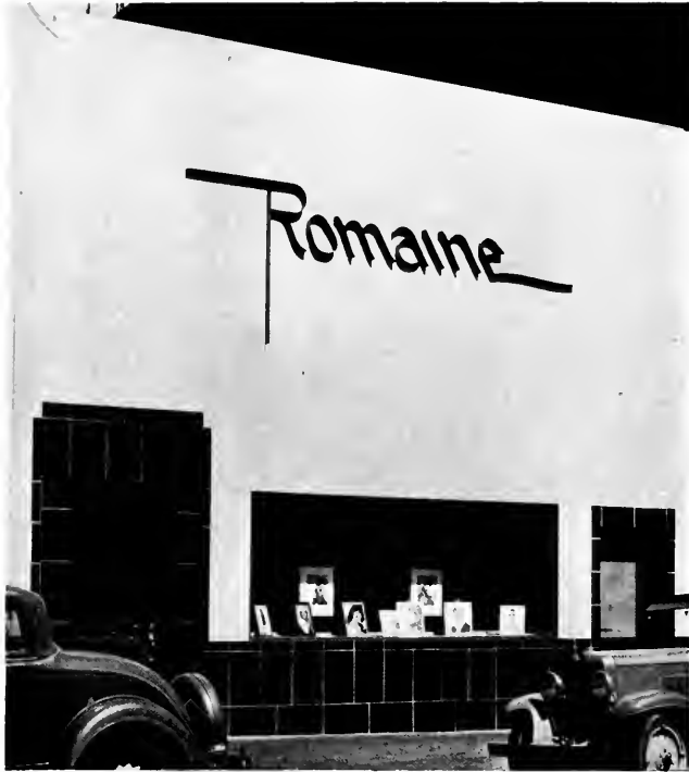
THEATRICAL PICTURE STUDIO, SAN FRANCISCO Bliss and Fairweather, Architects Exterior white and black unit tile
