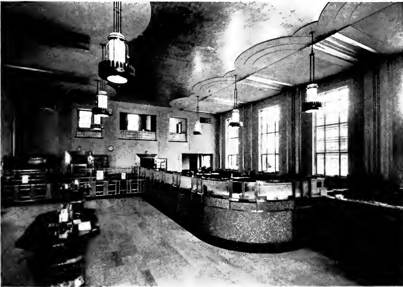
INTERIOR, WEST PORTAL BRANCH, SAN FRANCISCO BANK Wilbur D. Peugh, Architect Note interesting treatment of ceiling
