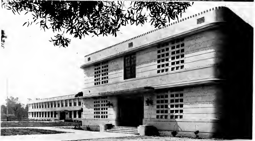
MANUAL ARTS HIGH SCHOOL GROUP, LOS ANGELES, CALIFORNIA JOHN PARKINSON AND DONALD B. PARKINSON, ARCHITECTS
