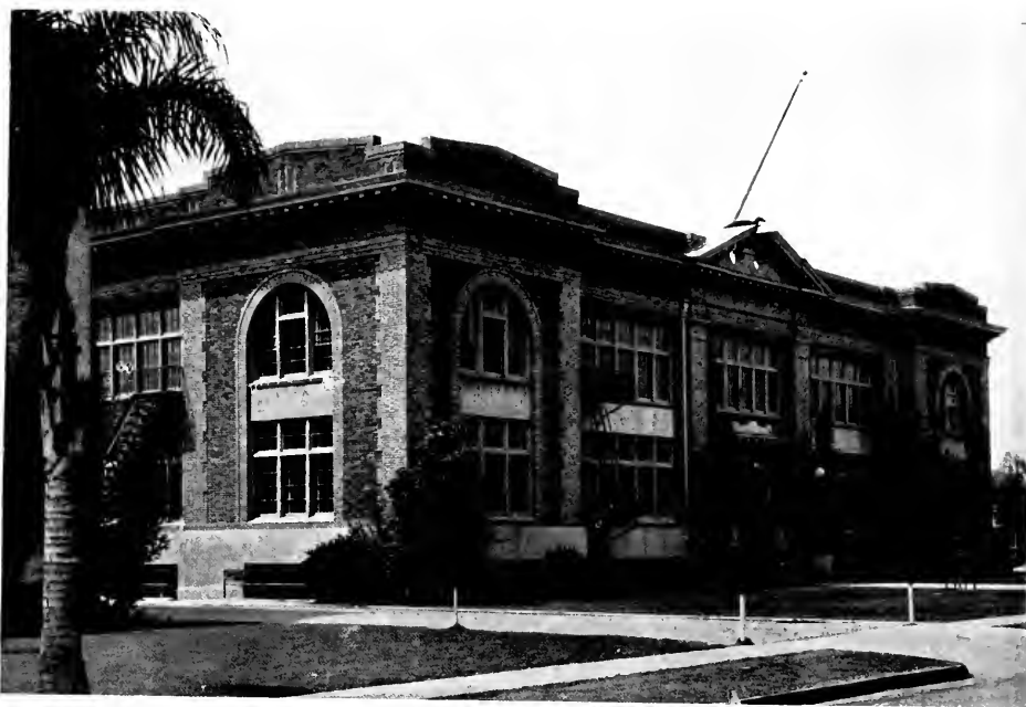
BEFORE ALTERATIONS—BUILT IN 1924 FINE ARTS BUILDING, INGLEWOOD UNION HIGH SCHOOL, INGLEWOOD, CALIFORNIA
