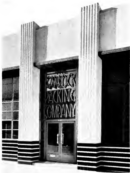
DETAIL OF ENTRANCE, BUILDING FOR GARLOCK PACKING COMPANY, SAN FRANCISCO
