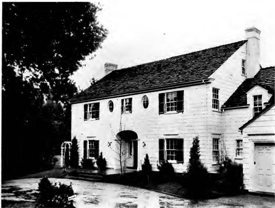
RESIDENCE OF JOHN M. HOLMES, HILLSBOROUGH, CALIFORNIA Noble Newsom and Archie T. Newsom, Architects
