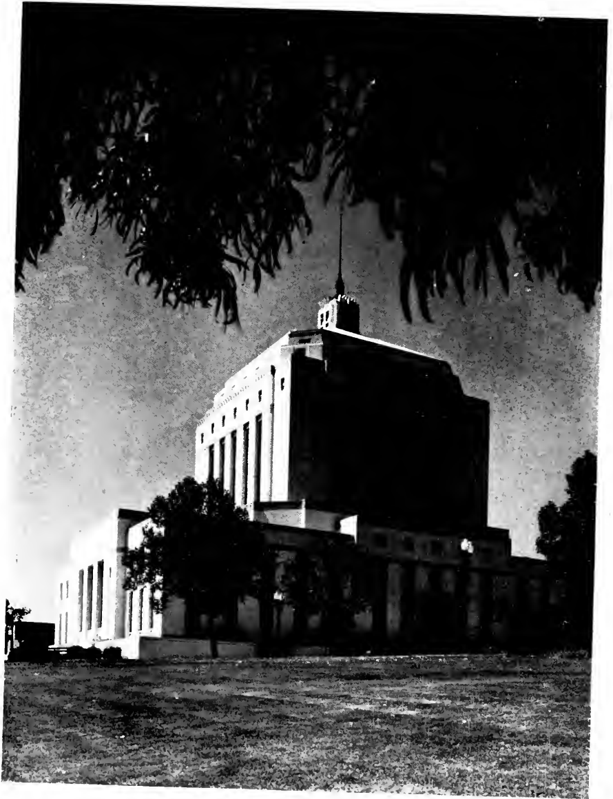
GEORGE WAGNER AND K. E. PARKER COMPANY, GENERAL CONTRACTORS COURT HOUSE AND HALL OF RECORDS, OAKLAND, CALIFORNIA W. G. CORLETT, J. W. PLACHEK, H. A. MINTON, W. E. SCHIRMER AND CARL WERNER, ARCHITECTS
