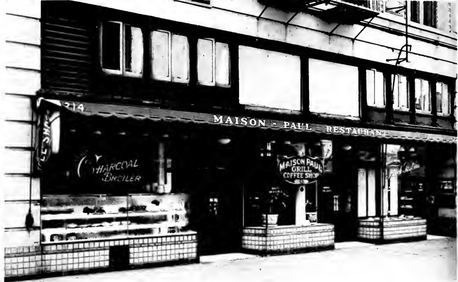
MAISON-PAUL RESTAURANT, SAN FRANCISCO Dodge A. Riedy, Architect View before remodeling
