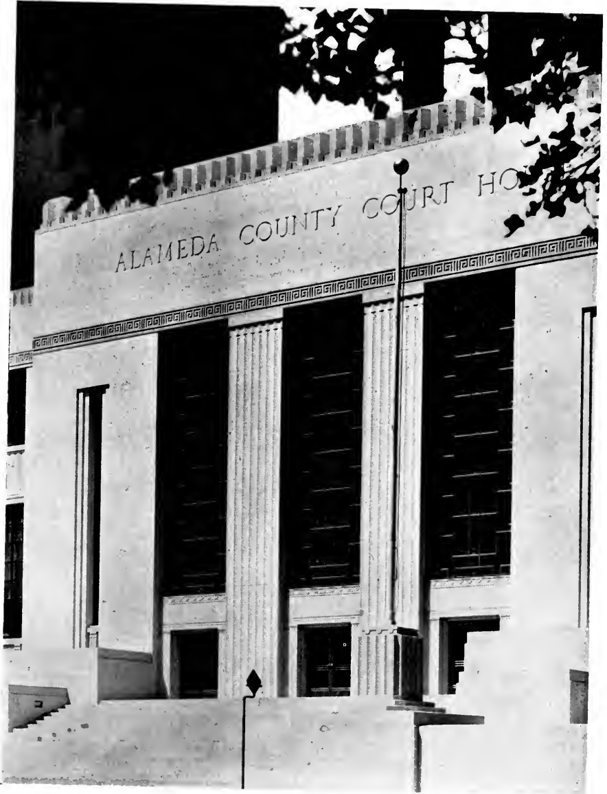
DETAIL OF FALLON STREET FRONT, COURT HOUSE AND HALL OF RECORDS, OAKLAND, CALIFORNIA
