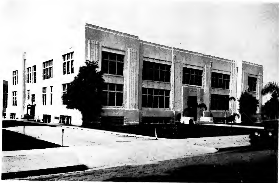
AFTER ALTERATIONS—COMPLETED 1936 FINE ARTS BUILDING, INGLEWOOD UNION HIGH SCHOOL, INGLEWOOD, CALIFORNIA T. C. Kistner, Architect
