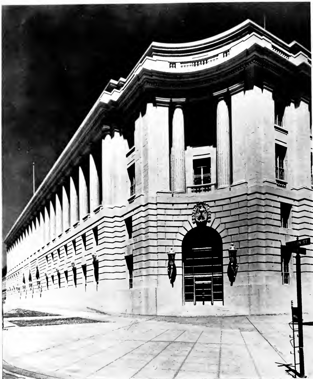
DETAIL OF FACADE, FEDERAL OFFICE BUILDING, SAN FRANCISCO ARTHUR BROWN, JR., ARCHITECT General Direction of the Treasury Department
