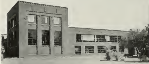
West Unit, Engineering Bldg.
