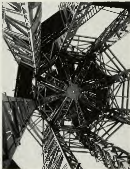
Detail of Tower Framework, Looking Up.
