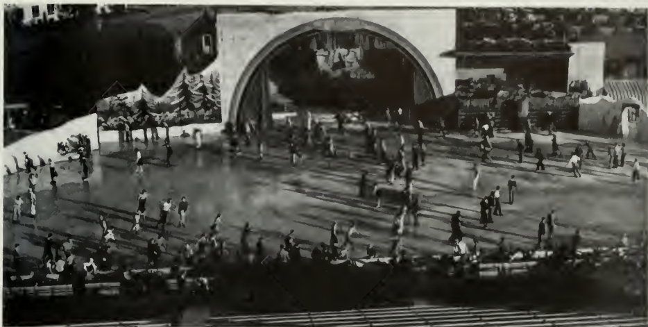
SOUTHERN CALIFORNIA'S LATEST RECREATION SPOT—MADE POSSIBLE BY USING NATURAL GAS AS FUEL FOR DRIVING AMMONIA COMPRESSOR UNITS
