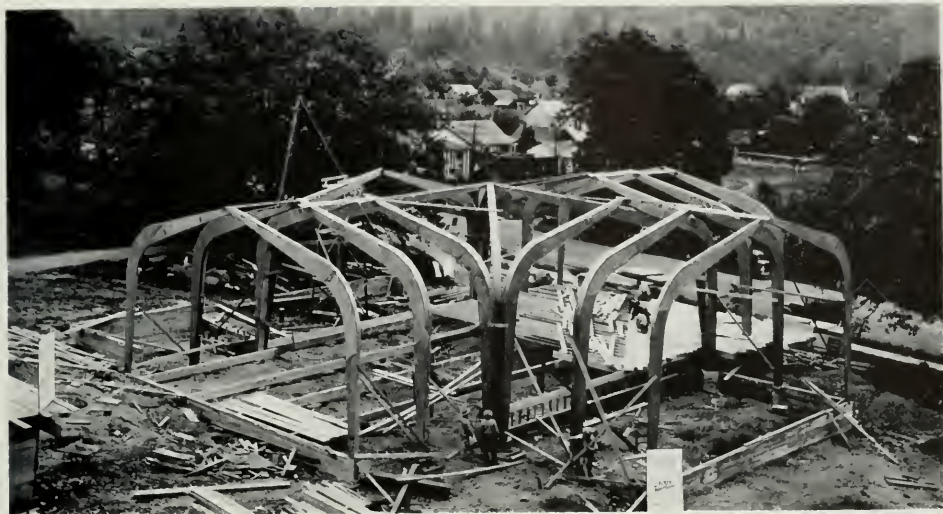
VIEW OF FRAMEWORK, COMBINATION AUDITORIUM AND GYMNASIUM, WHITE SALMON, WASHINGTON
