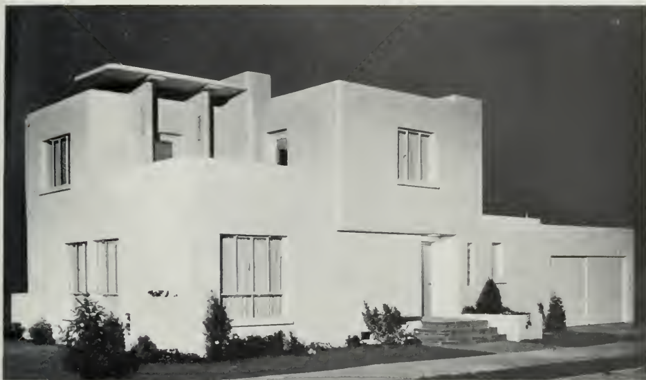
NEW TYPE OF CONCRETE HOUSE, ALAMEDA, CALIFORNIA Frederick H. Slocombe, Architect
