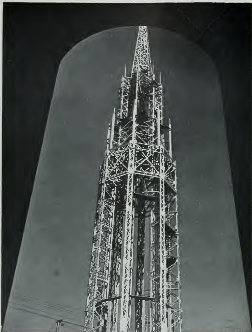
Structural steel fabricated and erected by Judson Pacific Company
