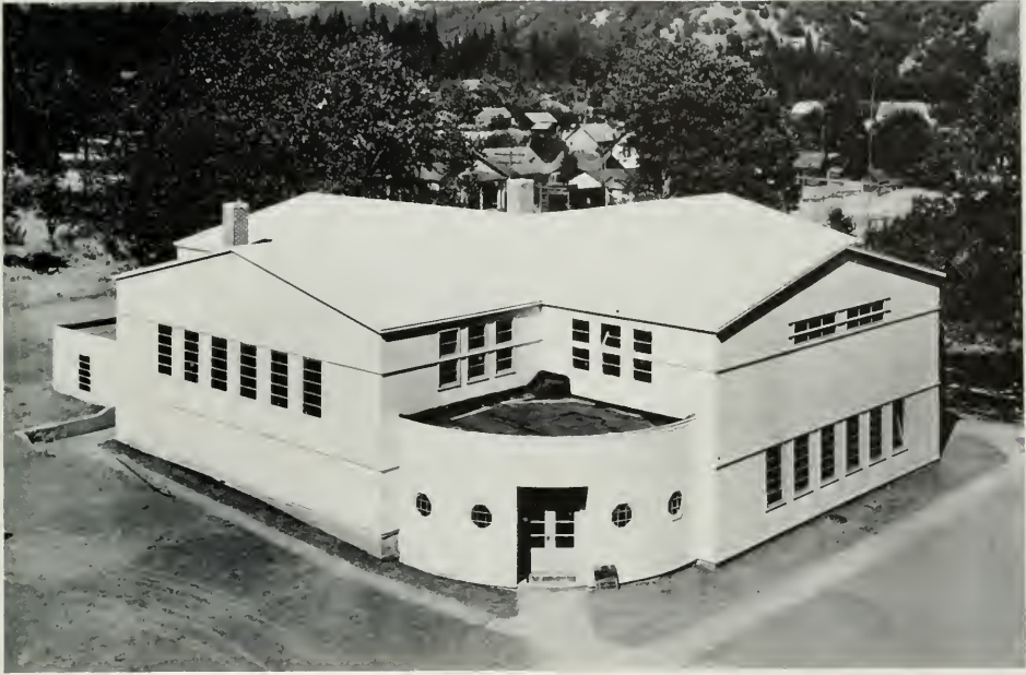
COMBINATION SCHOOL, AUDITORIUM AND GYMNASIUM, WHITE SALMON, WASHINGTON Walter H. Rothe, Architect
