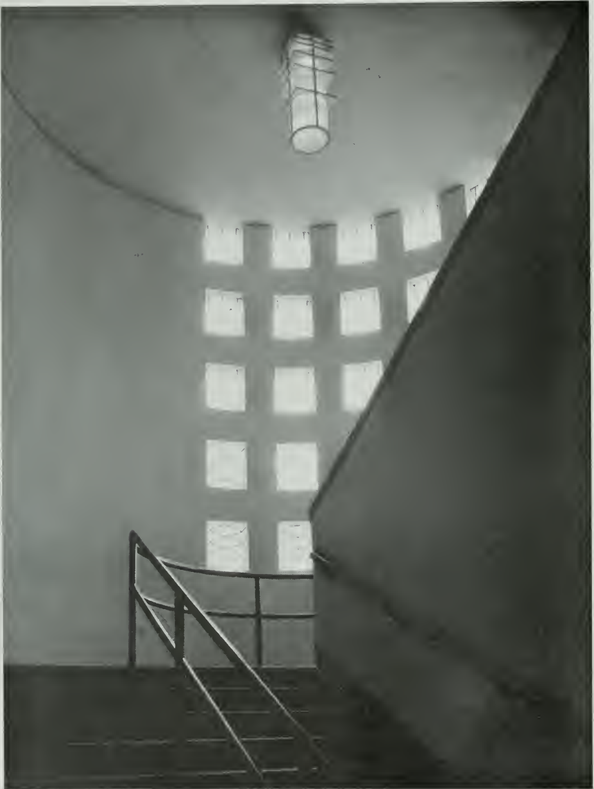
CONCRETE GRILLE WHICH LIGHTS THE MAIN STAIR HALL OF HOLLYWOOD HIGH SCHOOL MARSH, SMITH & POWELL, ARCHITECTS
