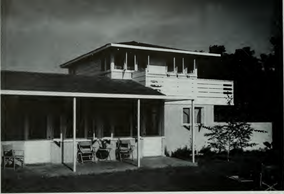
GARDEN VIEW, HOUSE FOR DR. IAN CAMPBELL, PASADENA, CALIFORNIA Erle Webster and Adrian Wilson, Architects
