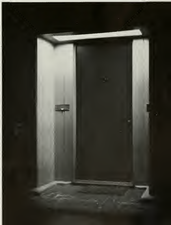
ENTRANCE, RESIDENCE OF MR. AND MRS. FOSTER K. SAMPSON THEODORE CRILEY, JR., ARCHITECT
