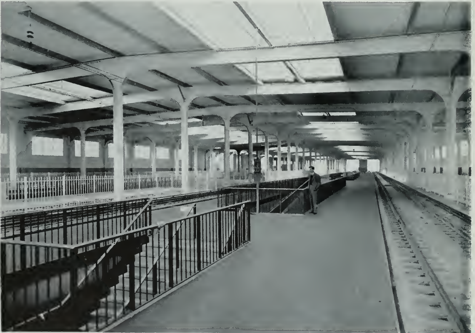
Bay Bridge electric railway trains enter and leave over this track level in the Terminal Building. Six tracks have been provided for Interurban (S. P.), Key System, and Sacramento Northern trains. Eleven ramps and fourteen stairways afford ample access to and from trains.
