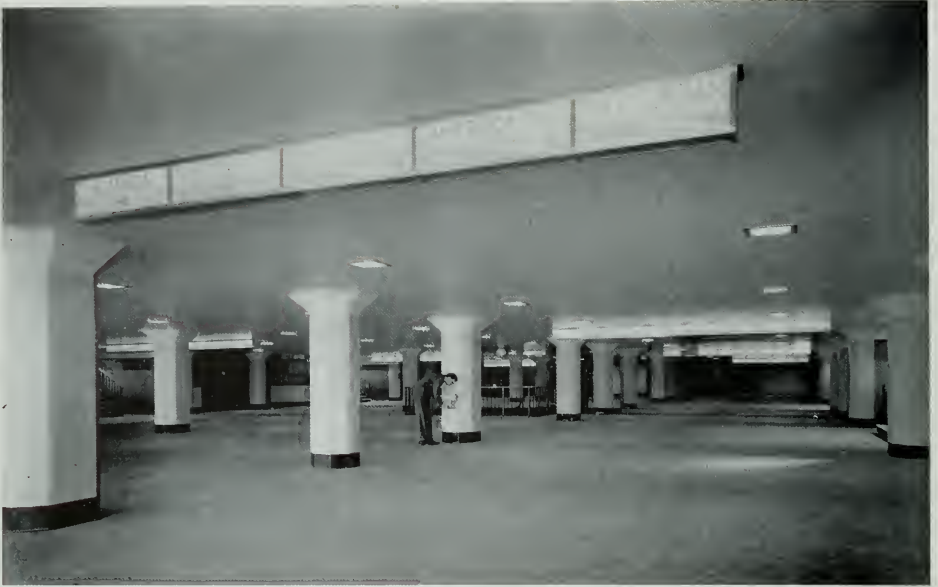
Passengers for the Bay Bridge electric railway find their trains through means of directional signs placed on the mezzanine floor of the Terminal Building. Floors are terrazzo with tile columns and specially-treated ceilings. Ticket offices are visible in the left center.
