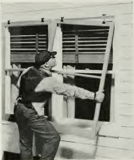
Window Conditioning (double-glass insulation) may be accomplished with storm sash or winter windows which hang from the same fastenings used to support screens in summer. Note how readily the storm sash "blends" in with its surroundings.
