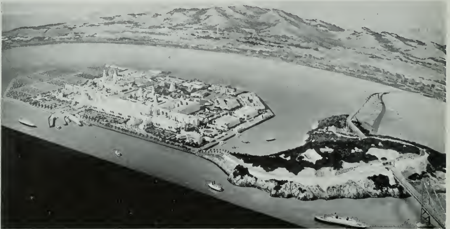
VIEW OF EXPOSITION ON MAN-MADE ISLAND. SAN FRANCISCO BAY BRIDGE ON RIGHT.
