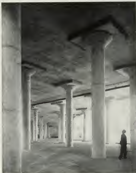
PARKING AREA UNDER THE BRIDGE VIADUCT, WESTERLY END OF TERMINAL BUILDING
