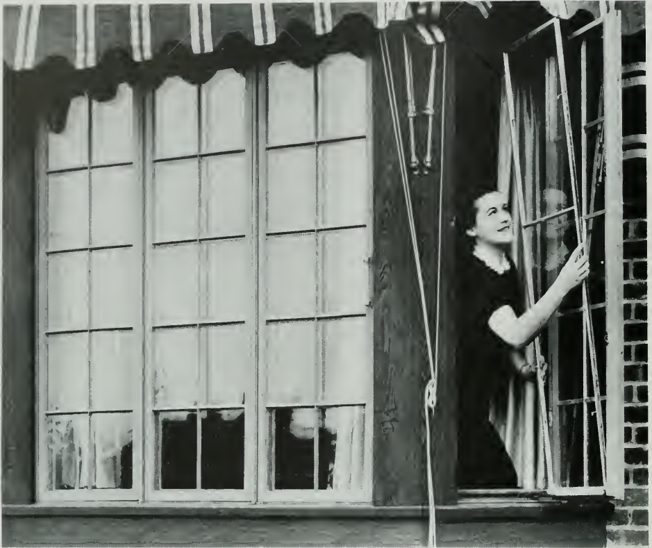
It requires only a few minutes to Window Condition a home that is equipped with modern prefabricated double-glazed sash. The glass is quickly and securely fastened into a special recess provided to receive it.
