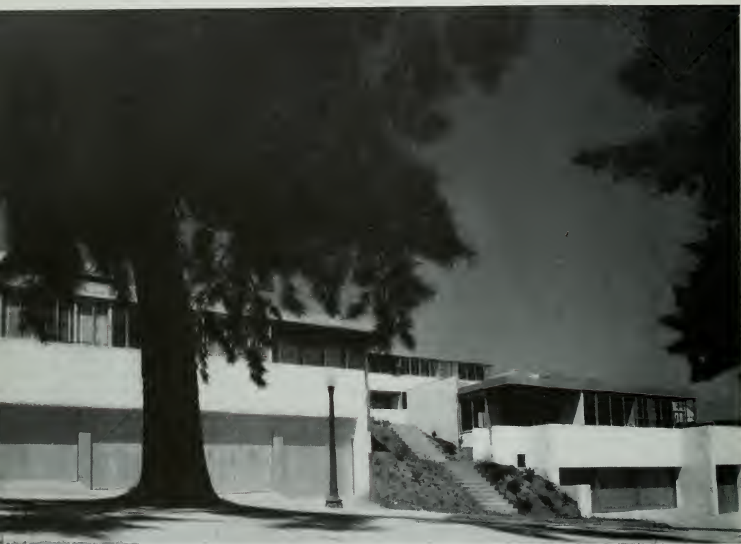
STRATHMORE DWELLINGS, LOS ANGELES RICHARD J. NEUTRA, ARCHITECT
