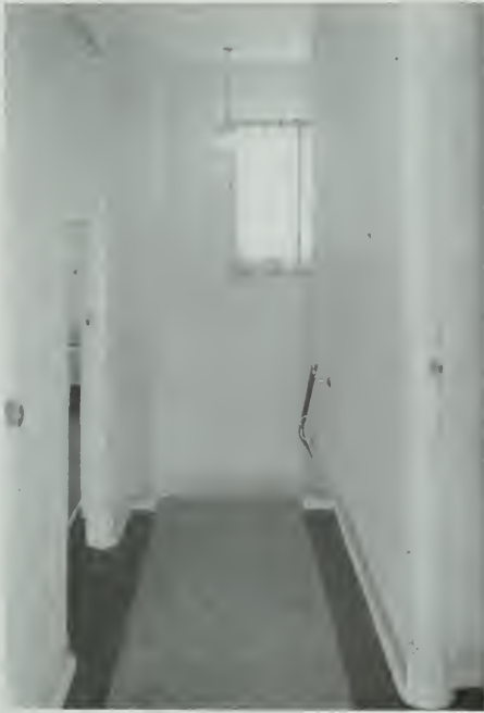
INTERIOR VIEW OF ALAMEDA CONCRETE HOUSE, showing trim and base moulds in cast concrete.
