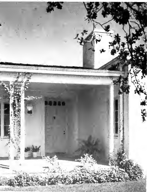
DETAIL OF ENTRANCE
