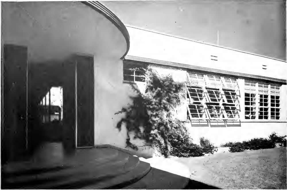
SOUTH PASADENA HIGH SCHOOL—ENTRANCE TO SCIENCE BUILDING
