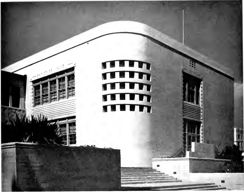
Millwork by Graves
