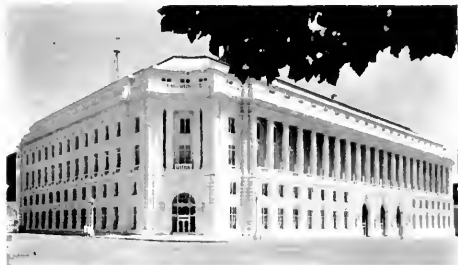
FEDERAL BUILDING • CIVIC CENTER • SAN FRANCISCO
