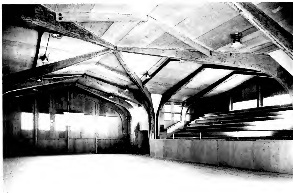
INTERIOR OF AUDITORIUM—NOTE USABLE CUBIC AREA WITH NO WASTE SPACE TO HEAT AND LIGHT. ACOUSTICAL PROPERTIES IDEAL
