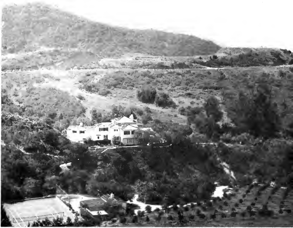
AERIAL VIEW OF HOUSE AND GROUNDS, RESIDENCE OF MR. AND MRS. ARTHUR HORNBLow, JR.
