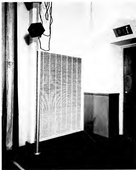
CORNER OF THE STAGE OF STUDIO D, N. B. C.'S NEW HOLLYWOOD RADIO CITY. THE GRILLING HIDES A HUGE AIR DUCT
