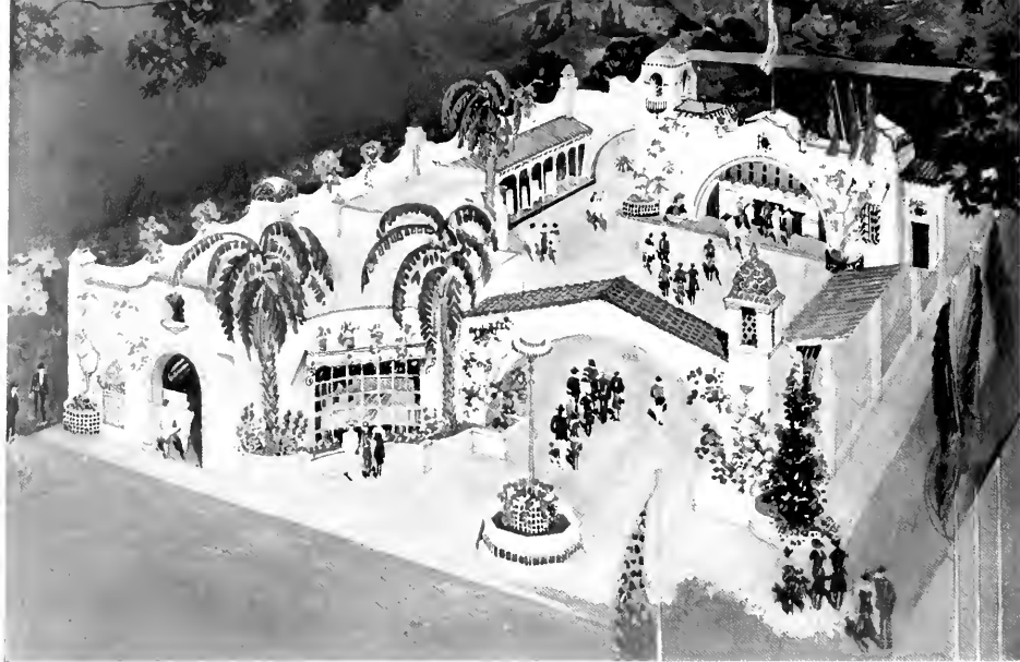
COOPERATIVE GAS INDUSTRY BUILDING AT TREASURE ISLAND
