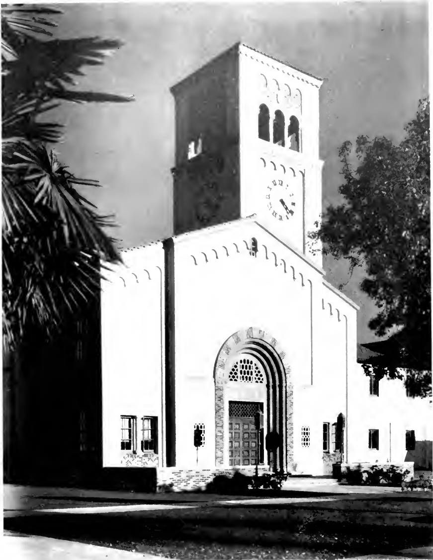
THE picture shows the main building of an interesting educational group which Marsh, Smith & Powell have built at a cost of $410,000. The structure is of reinforced concrete, style "California Romanesque," with an unusual use of tapestry brick inserts and panels in the concrete.
