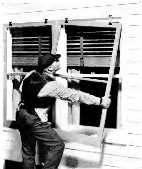
Window Conditioning (double-glass insulation) may be accomplished with storm sash or winter windows which hang from the same fastenings used to support screens in summer. Note how readily the storm sash "blends" in with its surroundings.
