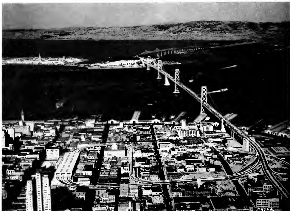
Graphic combination aerial view and artist's drawing illustrating how the San Francisco Bay will look when the Exposition opens in February. Front foreground is the viaduct and the Bridge Terminal Building extending to the great 4\frac{1}{2} -mile steel span. Left center is the completed Treasure Island showing the roadway connections via Yerba Buena Island to the Bay Bridge. The photograph, taken from San Francisco, looks eastward to Berkeley and Oakland.
