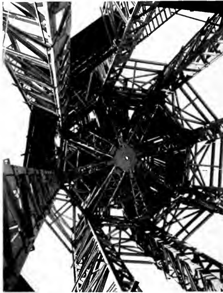
Detail of Tower Framework, Looking Up.
