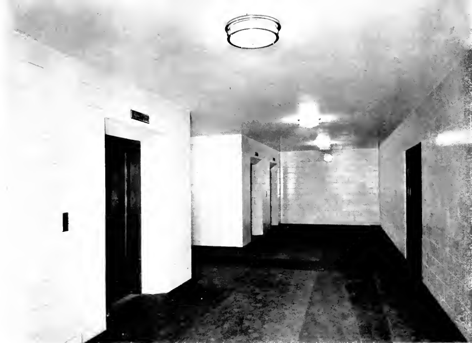
VIEW IN SUBBASEMENT OF LIBRARY OF CONGRESS ANNEX, WASHINGTON, D. C., SHOWING ELEVATOR TERMINALS AND END OF CORRIDOR THAT JOINS THE ANNEX TO THE MAIN LIBRARY OF CONGRESS. GLAZED TERRA COTTA WALL UNITS ARE OF KRAFTILE. THE PRODUCT OF THE COMPANY AT NILES, CALIFORNIA, WAS SELECTED AFTER NATION-WIDE BIDDING.
