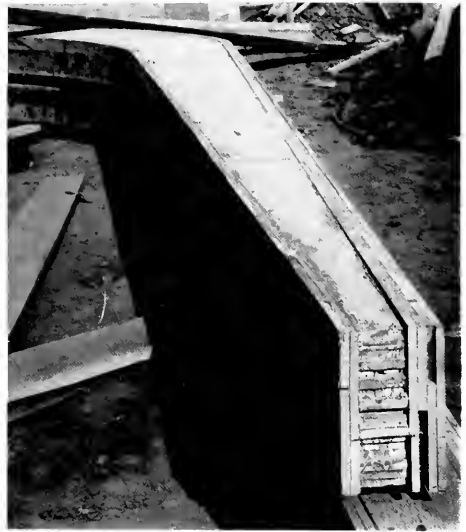
SHOWING TAPERED END OF STRESS-COVERED PLYWOOD, LAMINATED BENT BEFORE THE END WAS TRIMMED
