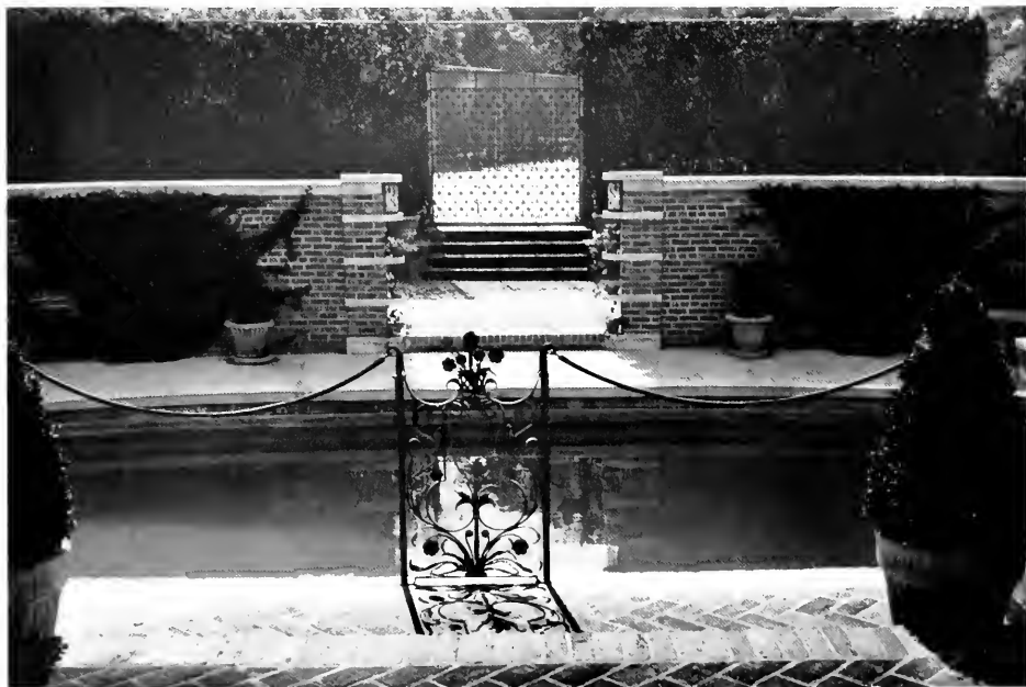
SWIMMING POOL, RESIDENCE OF A. H. BRAWNER James H. Mitchell, Architect
