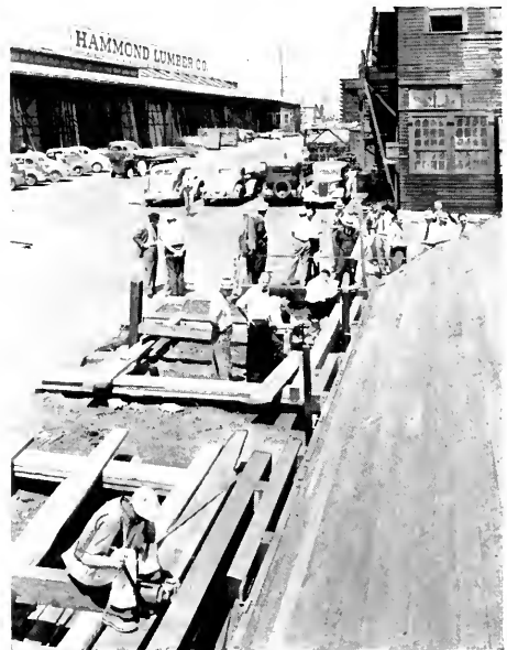
APPLYING LATERAL LOAD ON WEST SILL ONLY BY MEANS OF HYDRAULIC JACKS. DISTRIBUTING BEAM SYSTEM FOR EVEN APPLICATION OF LOAD TO SILL IS SEEN IN FOREGROUND.
