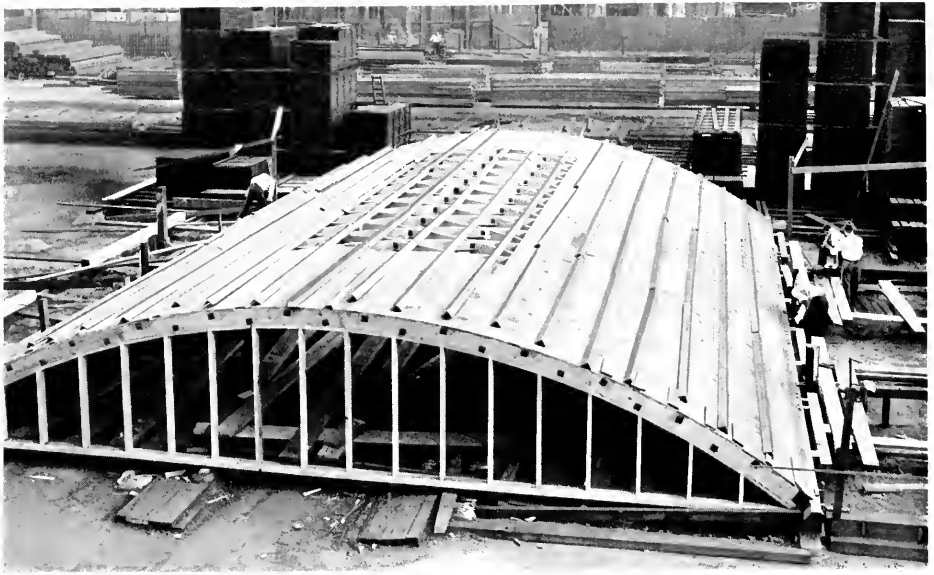
LAMELLA TEST ROOF DURING FINAL EXPERIMENT. SHEATHING REMOVED ON CENTER OF ROOF. END DIAPHRAGM SHEATHING REMOVED LEAVING ENDS UNSUPPORTED. STEEL ANGLES APPROXIMATE WEIGHT OF ROOFING. IN THIS TEST A LATERAL LOAD OF 390 POUNDS PER LINEAL FOOT OF SILL WAS APPLIED ON THE WEST SILL ONLY.
