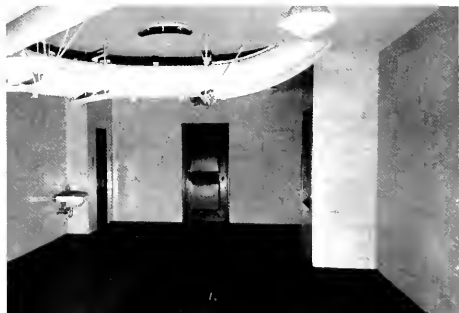
SUBBASEMENT OF LIBRARY OF CONGRESS ANNEX, WASHINGTON, D. C., SHOWING INSTALLATION OF 8 x 16 GLAZED TERRA COTTA WALL UNITS, STANDARD SIZE OF KRAFTILE COMPANY OF NILES, CALIFORNIA. JUTTING FROM WALL AT RIGHT IS SPECIAL "DUMB-WAITER" FOR TRANSPORTING BOOKS.
