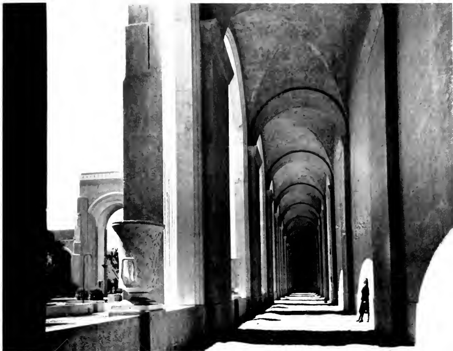
DETAIL OF CLOISTER, COURT OF FLOWERS, TREASURE ISLAND LEWIS P. HOBART, ARCHITECT
