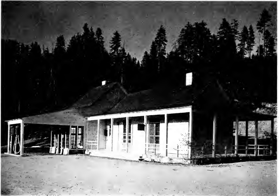
NOTE SIMILARITY OF COMPLETED BUILDING TO MR. BLANCHARD'S PERSPECTIVE OF CHINQUAPIN STATION
