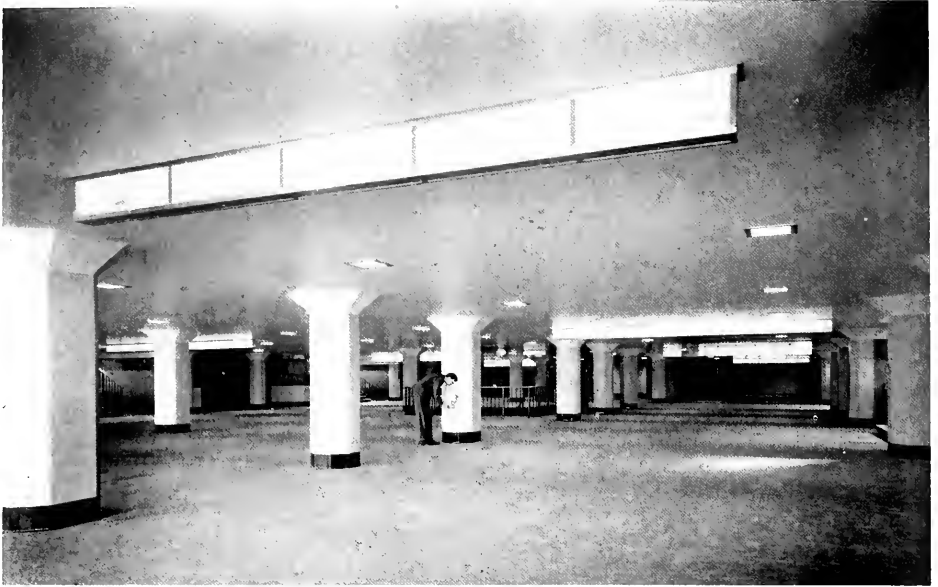
Passengers for the Bay Bridge electric railway find their trains through means of directional signs placed on the mezzanine floor of the Terminal Building. Floors are terrazzo with tile columns and specially-treated ceilings. Ticket offices are visible in the left center.
