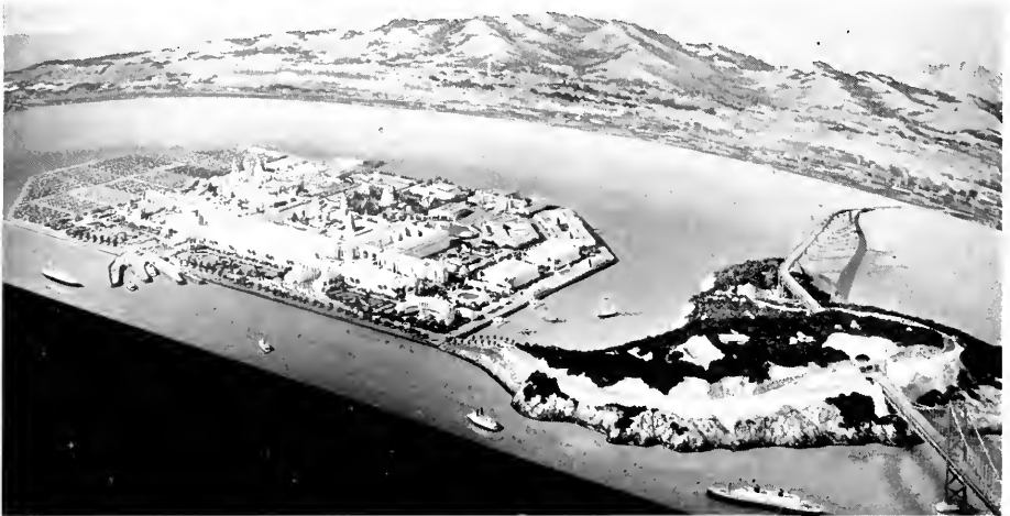
VIEW OF EXPOSITION ON MAN-MADE ISLAND. SAN FRANCISCO BAY BRIDGE ON RIGHT.
