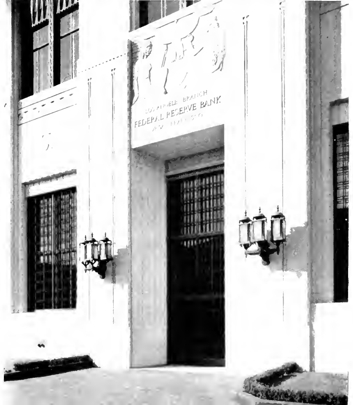
LOS ANGELES BRANCH, FEDERAL RESERVE BANK OF SAN FRANCISCO
