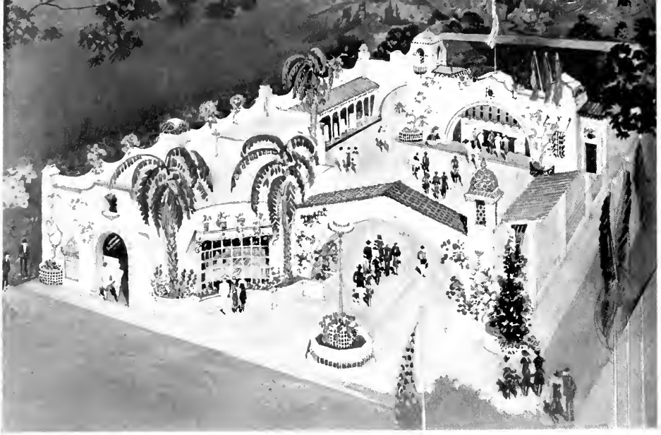
COOPERATIVE GAS INDUSTRY BUILDING AT TREASURE ISLAND
