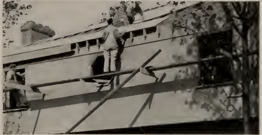
The Plyscord-sheathed walls of this residence in Seattle, Wash., are 40% more rigid than if diagonal board sheathing had been used. The big panels also save up to 80% on sawing, fitting and joining... 50% on nailing. Tenny Francis Bellamy was the architect on this residence.
