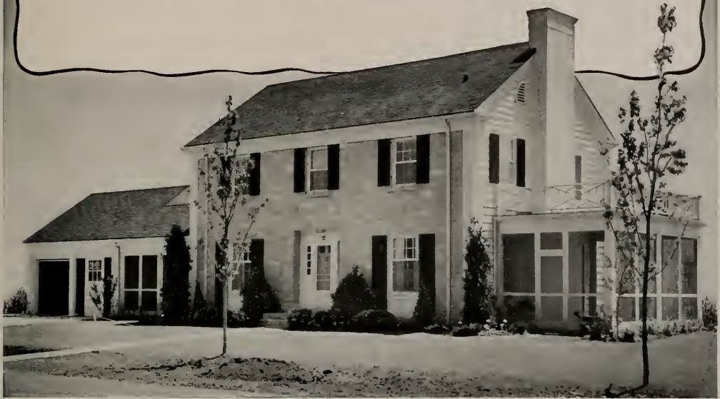
W. C. Tackett, Inc., Builders, Chicago Herman Brunt, Architect
