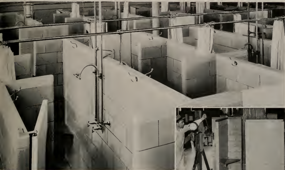
Vallejo, California. High School. John J. Donovan, architect. Reed & Reed, masonry contractors. Inset photograph shows preliminary testing of Kraftile Terra Cotta Wall Unit reinforced partitions in Kraftile plant at Niles, California
