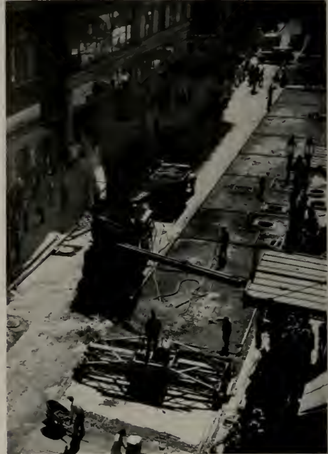
PAVING PLANT AT WORK ON POST STREET, SAN FRANCISCO
