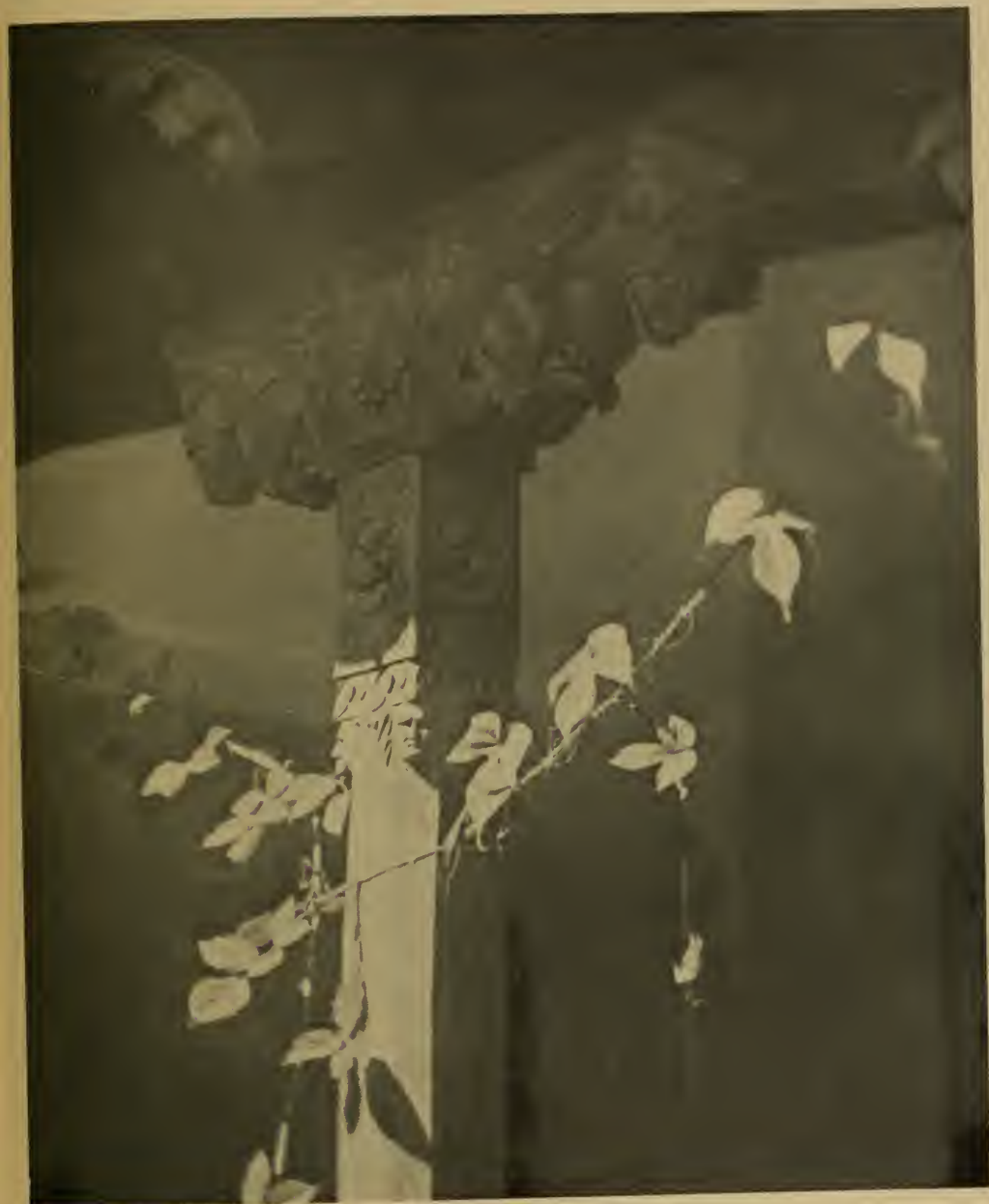
LOGGIA POSTS AND BRACKETS
