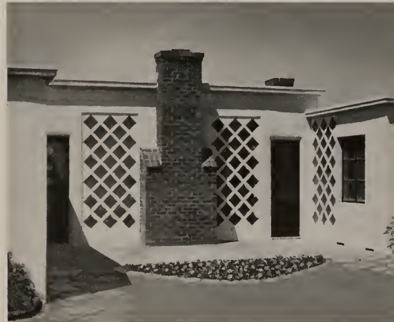
Patio view, showing interesting treatment of diamond "Grid Forms."
