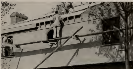
WALL SHEATHING The Plyscord-sheathed walls of this residence in Seattle, Wash., are 40% more rigid than if diagonal board sheathing had been used. The big panels also save up to 50% on sawing, fitting and joining... 50% on nailing. Tezaya Francis Bellamy was the architect on this residence.
