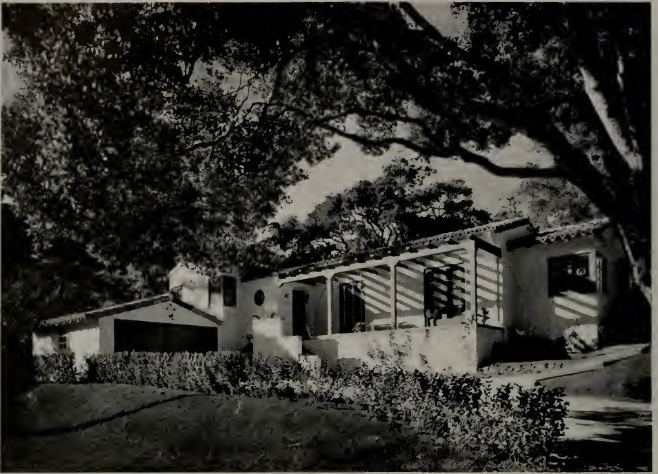
RESIDENCE OF HARRY R. BUTLER, HILLSBOROUGH, CALIFORNIA
