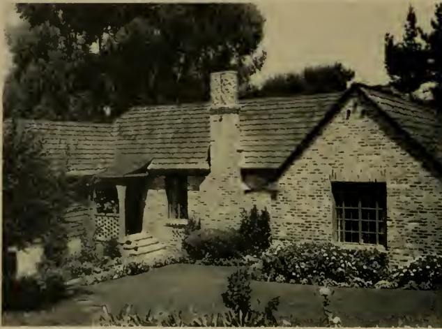
HOUSE FOR CHARLES H. ACKERSON, BURLINGAME HILLS, CALIFORNIA William Henry Rowe, Architect
