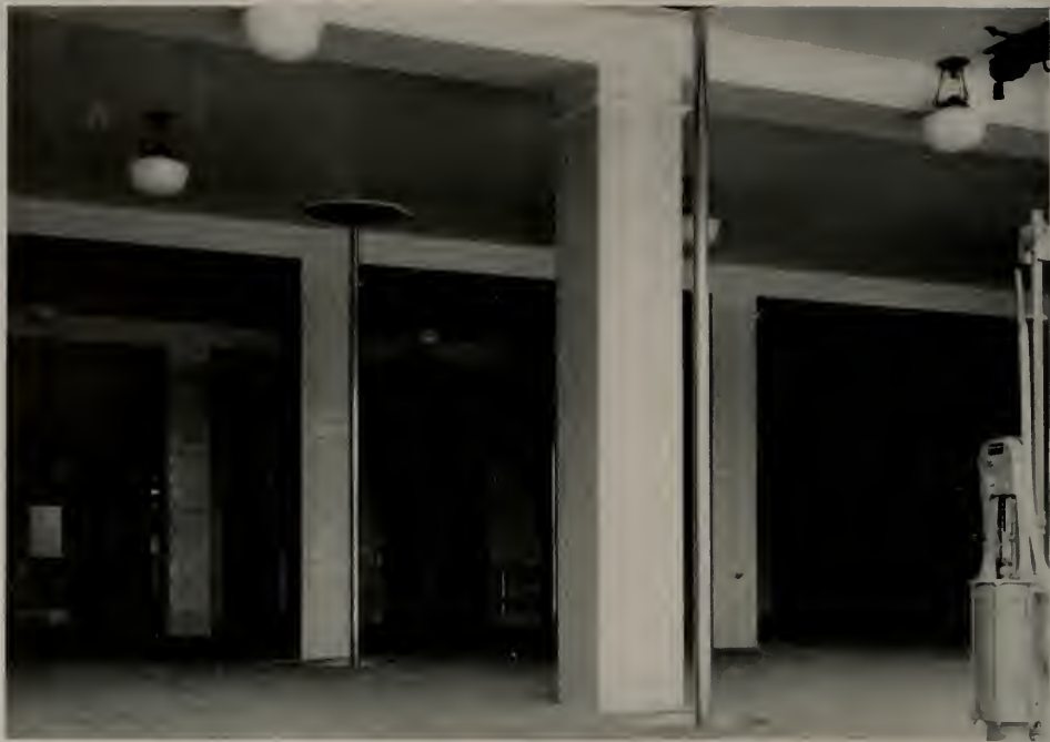
Glazed terra cotta wall units, Krafftile's 6 x 12's, precision sized, were specified for San Francisco's newest fire house, Number 35, in Bluxome Street, near Fourth Street. Designed and constructed by Bureau of Architecture, Board of Public Works, San Francisco; Dodge A. Riedy, City Architect.
