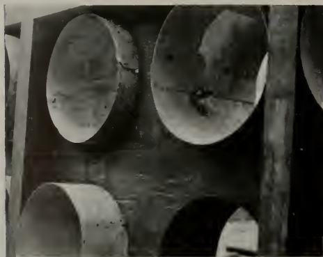
DETAILS OF CIRCULAR GRID FORM ASSEMBLY
