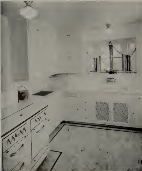
ALL-GAS KITCHEN IN HARRY L. BUTLER HOUSE, HILLSBOROUGH, CALIFORNIA
