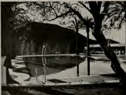
Arrowhead Springs Hotel Swimming Pool—Paul R. Williams and Gordon B. Kaufman, Architects. Builder: Paddock Engineering Company.
