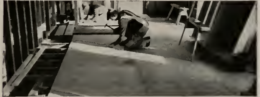
In this Stamford, Conn., home designed by Provest and Edwards, Plyscord provided a smooth base for finish flooring and linoleum—insulates and protects against drafts from below—gives a horizontal diaphragm to resist earthquakes and high winds. Recommended thicknesses are 1/2" and 5/8".
