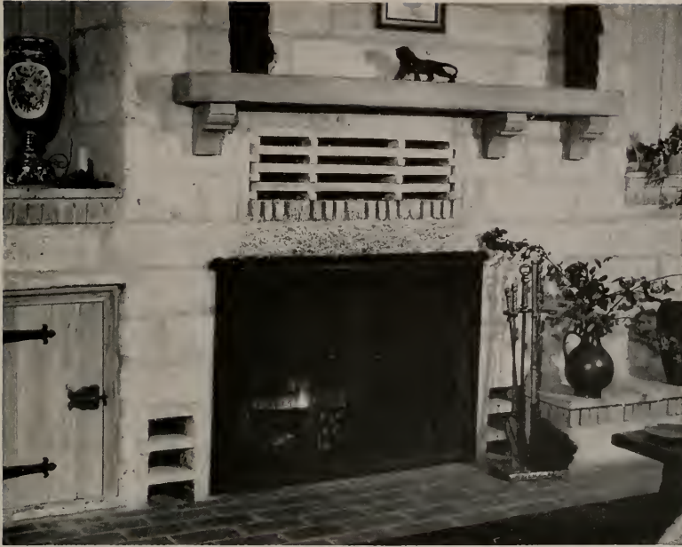
The Spanish influence is reflected in the fireplace pictured above. The bricks are of native California adobe, painted white. Intakes and outlet are formed of masonry.
