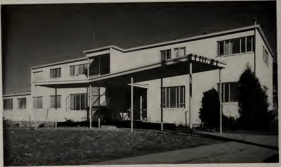
EXTERIOR FROM TELEGRAPH AVENUE
