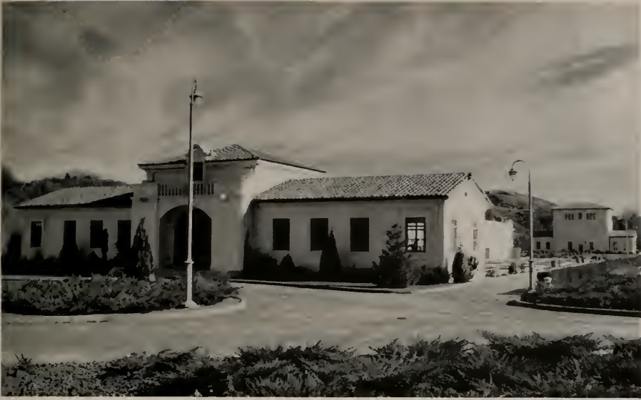
ADMINISTRATION BUILDING . . . CHEMICAL BUILDING IN DISTANCE
