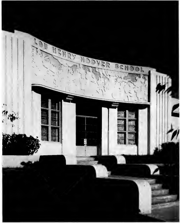
Close up of main entrance, Lou Henry Hoover School, Whittier, California.
