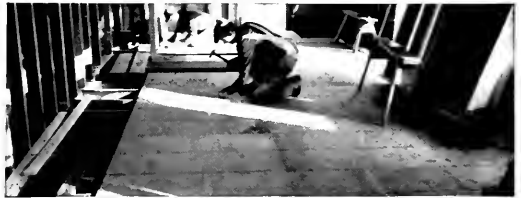
In this Stamford, Conn., home designed by Provost and Edwards, Plyscord provided a smooth base for finish flooring and linoleum—insulates and protects against drafts from below—gives a horizontal diaphragm to resist earthquakes and high winds. Recommended thicknesses are 1/2" and 5/8".
