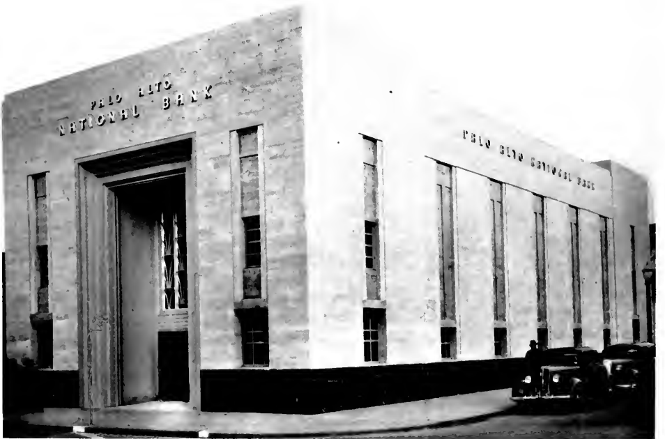
PALO ALTO NATIONAL BANK, PALO ALTO, CALIFORNIA Birge M. Clark and David B. Clark, Architects Classic in feeling, yet modern in detail.
