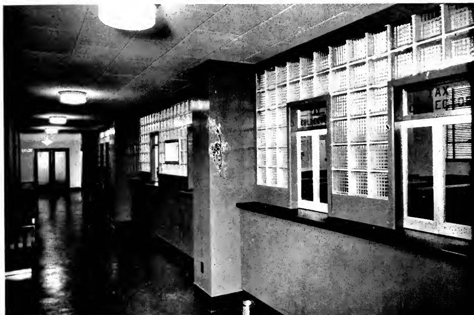
FIRST FLOOR CORRIDOR
