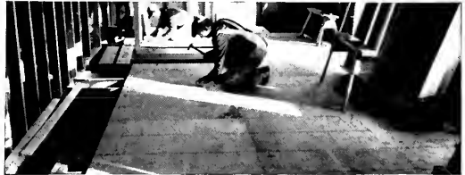
SUB-FLOORING In this Stamford, Conn., home designed by Provost and Edwards, Plyscord provided a smooth base for finish flooring and linoleum—insulates and protects against drafts from below—gives a horizontal diaphragm to resist earthquakes and high winds. Recommended thicknesses are 1/2" and 5/8".
