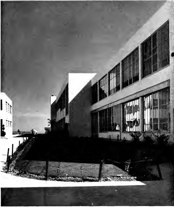
EMERSON JUNIOR HIGH SCHOOL, LOS ANGELES Richard J. Neutra, Architect
