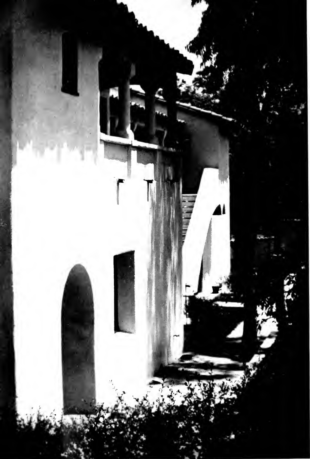
EXECUTIVE WING, BEL-AIR ADMINISTRATION BUILDING, LOS ANGELES, CALIFORNIA
