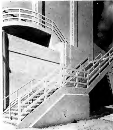
DETAIL OF BALCONY EXIT STAIRWAY
