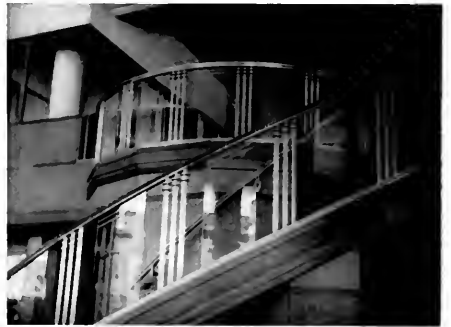
STAIRWAY TO MEZZANINE
