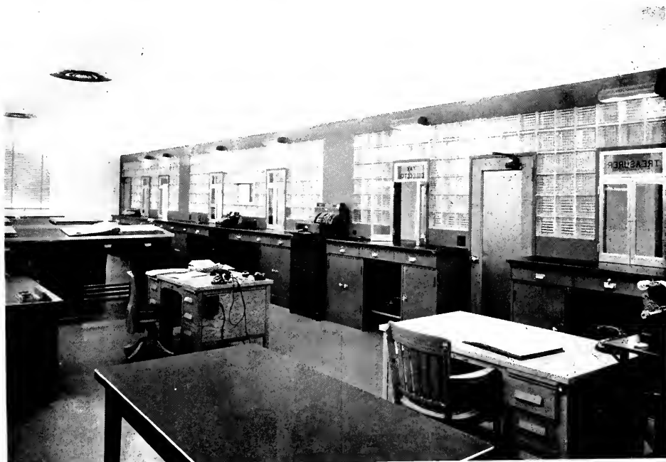
OFFICE SPACE WITH GLASS BLOCK PARTITION
