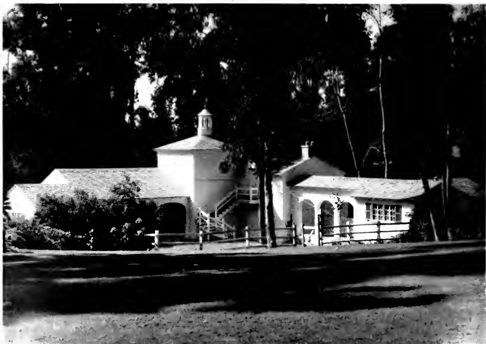
STABLES ON PRIVATE ESTATE, LOS ANGELES
