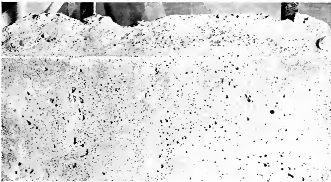
Surface voids disclosed by stoning the surface of a laboratory specimen cast under a sloping wood form. These voids are often hidden by a thin film of cement and fine sand; do not show up when forms are stripped in ordinary field operations.
