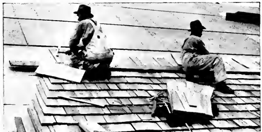
ROOF SHEATHING Plyscord is suitable for any type of roofing—shingles, composition roofing, asbestos tile or slate. Illustration shows Plyscord roof sheathing on a Portland, Ore., residence designed by Richard Sundeleaf.
