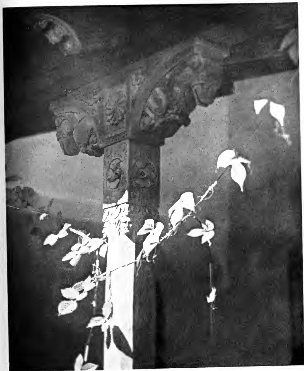
LOGGIA POSTS AND BRACKETS
