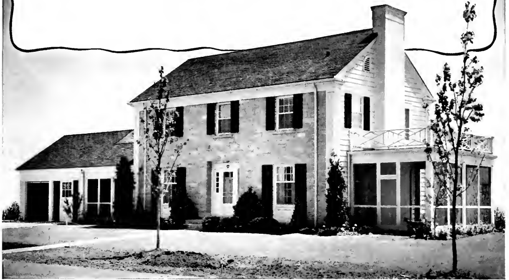
W. C. Tackett, Inc., Builders, Chicago Herman Bruns, Architect
