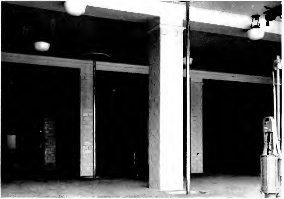
Glazed terra cotta wall units, Krafftile's 6 x 12's, precision sized, were specified for San Francisco's newest fire house, Number 35, in Bluxome Street, near Fourth Street. Designed and constructed by Bureau of Architecture, Board of Public Works, San Francisco; Dodge A. Riedy, City Architect.
