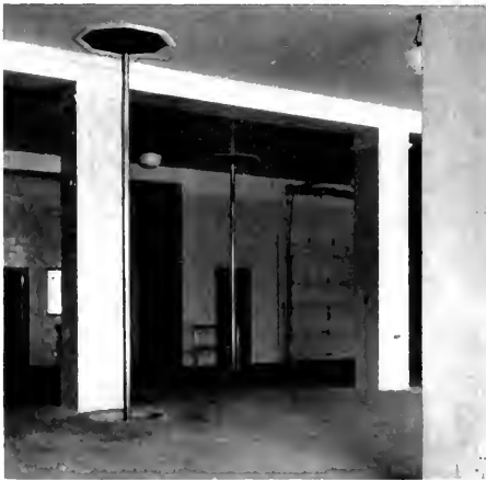
"Monterey Buff" was selected as the color for this installation which assures resistance to fire, acid stains, moistures, and other hard usage and at the same time affords a surface easy to clean and one that need never be painted or otherwise reconditioned.
