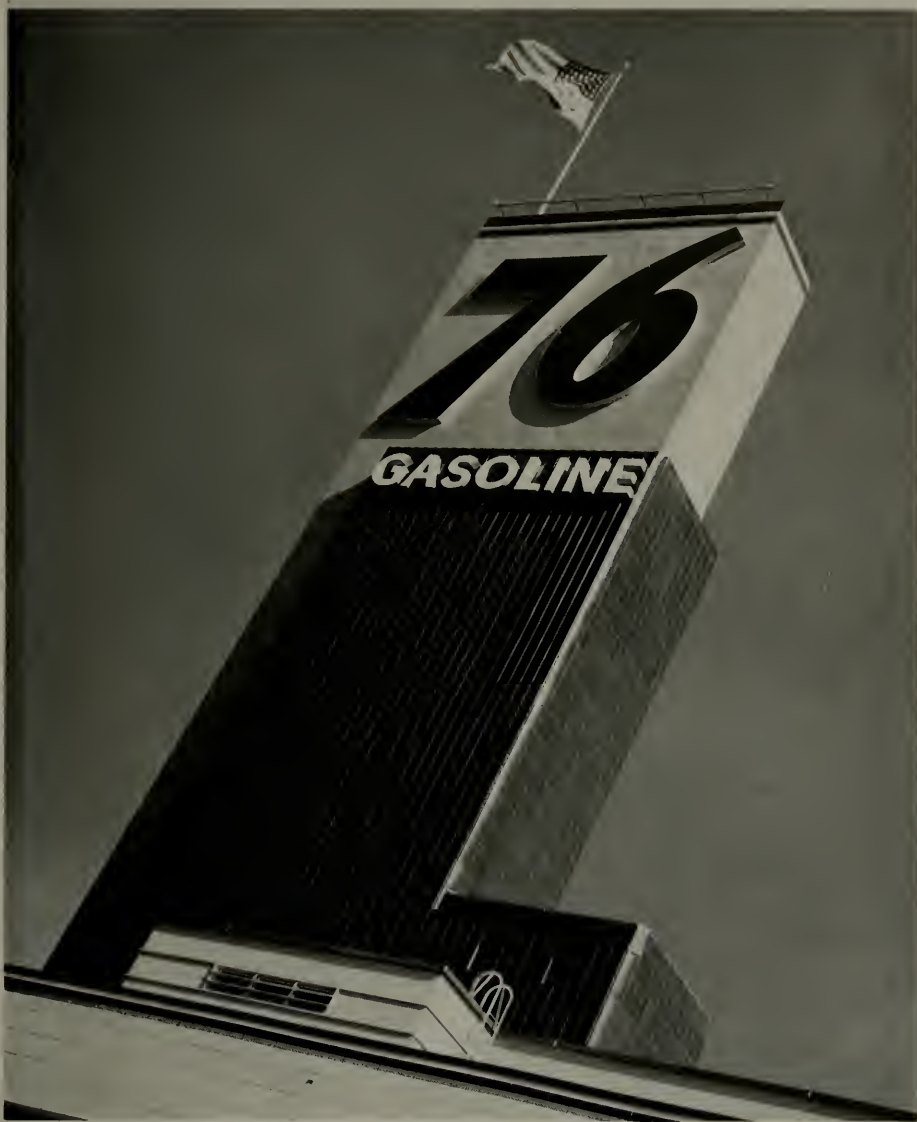
UNION OIL COMPANY BUILDING, SAN FRANCISCO, CALIFORNIA. THIS BUILDING IS ALSO SHOWN IN THE FRONTISPIECE TO THIS ISSUE. THE MAIN BUILDING IS PALE BUFF ADHESION TYPE CERAMIC VENEER; THE FLUTED PORTION OF THE TOWER IS DEEP BLUE ADHESION TYPE CERAMIC VENEER; THE PLAIN PORTION OF THE TOWER IS BRILLIANT ORANGE HERMOSA VENEER. LEWIS P. HOBART, ARCHITECT.
