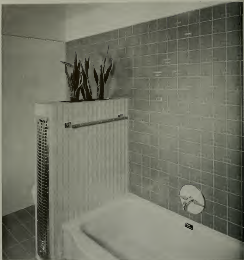
A LOS ANGELES BATH ROOM IN TILE. THIS SHOWS THE SUBTLE EFFECT OBTAINABLE FROM A SLIGHT FACE DEPRESSION, WHICH CATCHES THE LIGHT AT VARYING ANGLES.
