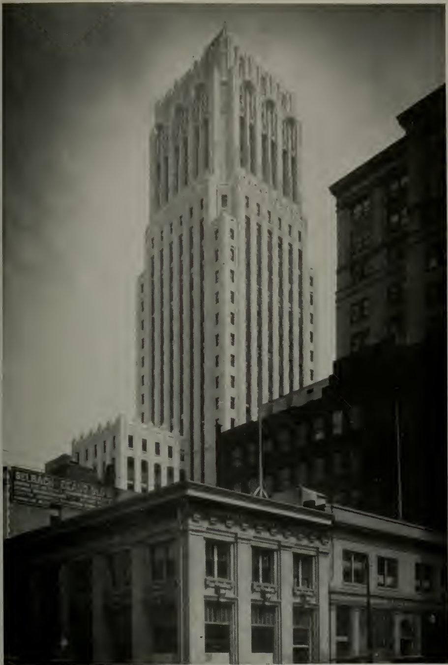
SHELL OIL BUILDING, SAN FRANCISCO, CALIFORNIA
