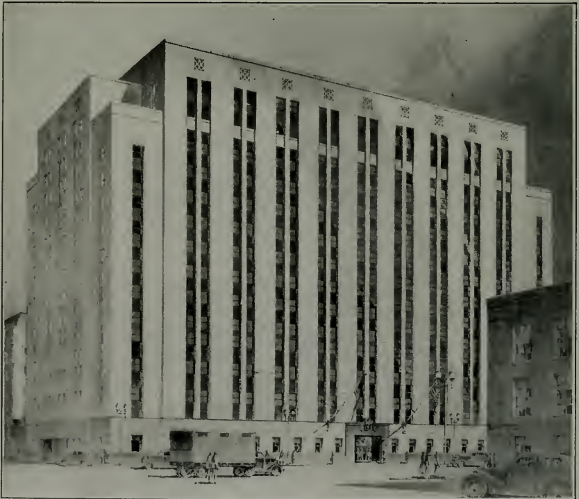
U. S. APPRAISERS STORES AND IMMIGRATION STATION UNDER CONSTRUCTION IN SAN FRANCISCO
