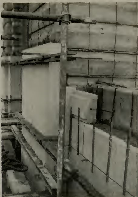
ANCHORED TYPE OF CERAMIC VENEER. ABOVE, UNITS IN PLACE AND GROUTED. BELOW, EXAMPLES OF THE SIZE OF UNIT THAT CAN BE PRODUCED BY MODERN TECHNICAL METHODS. NOTE ALSO THE PERFECTION OF SURFACES AND EDGES.
