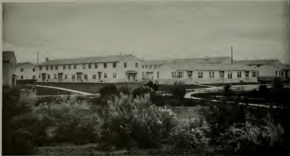
CARMELITOS HOUSING PROJECT, LONG BEACH, CALIFORNIA. KENNETH S. WING, ARCHITECT. ABOVE IS A GENERAL VIEW. ALL ROOFS ARE LIGHT WEIGHT INTERLOCKING SHINGLE TILE.
