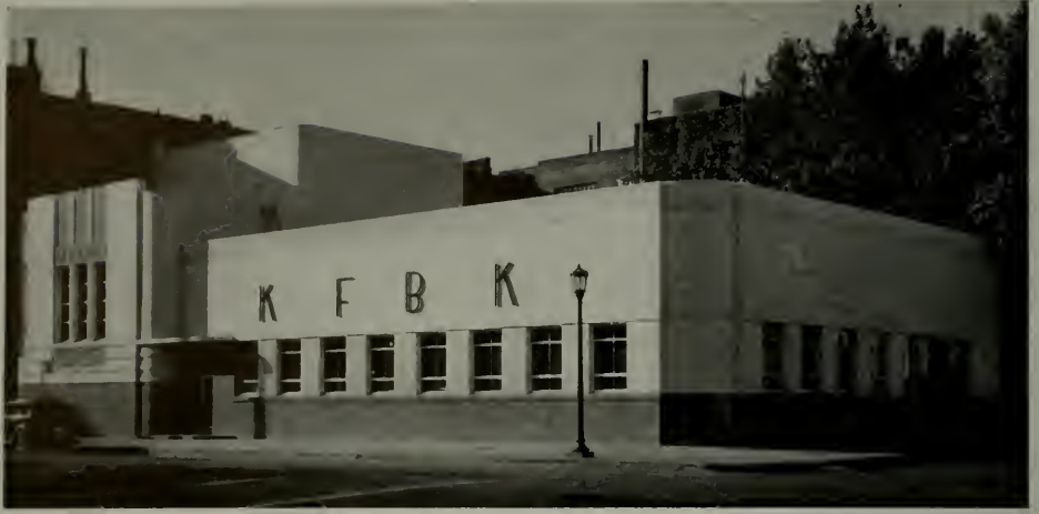
STUDIO OF KFBK, SACRAMENTO, CALIFORNIA. HARRY DEVINE, ARCHITECT. EXTERIOR WALLS VENEERED WITH N. CLARK & SONS' ADHESION TYPE CERAMIC UNITS.
