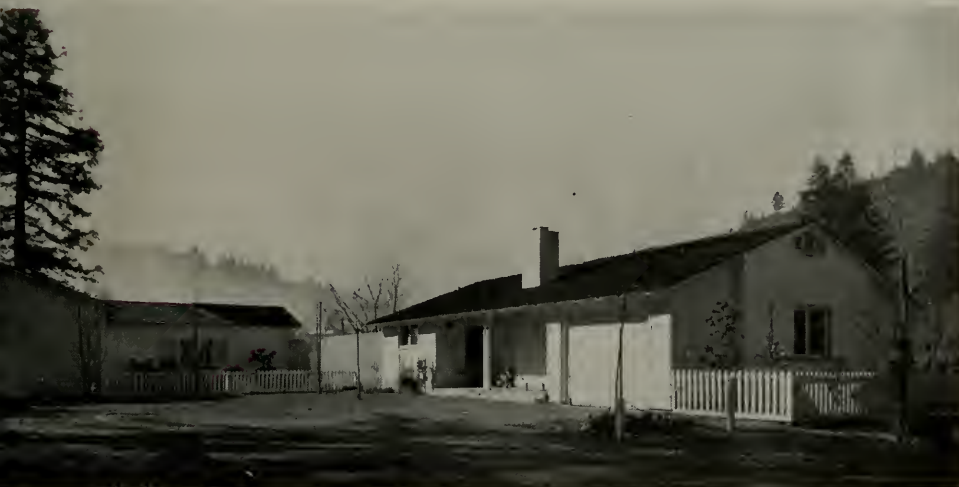
houses in Redwood City; designed for vacation use but adequate for all year living. Blanchard and Maher, Architects
