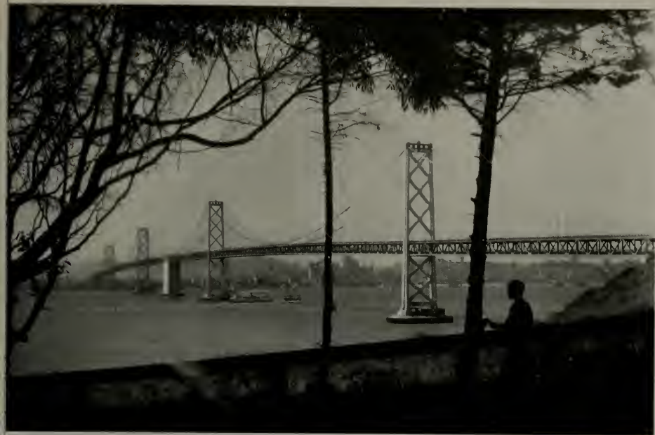
VIEW OF THE BAY BRIDGE LOOKING TOWARD SAN FRANCISCO FROM YERBA BUENA ISLAND
