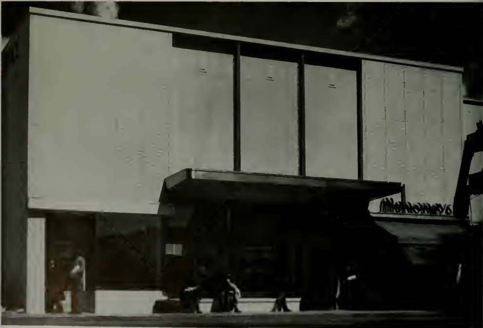
STORES AND TICKET OFFICE, BERKELEY, CALIFORNIA. HERTZKA & KNOWLES, ARCHITECTS. THE FLANKING PIERS ARE N. CLARK & SONS' CREAM FACE BRICK; THE CENTRAL PANELS YELLOW CERAMIC VENEER, ADHESION TYPE.
