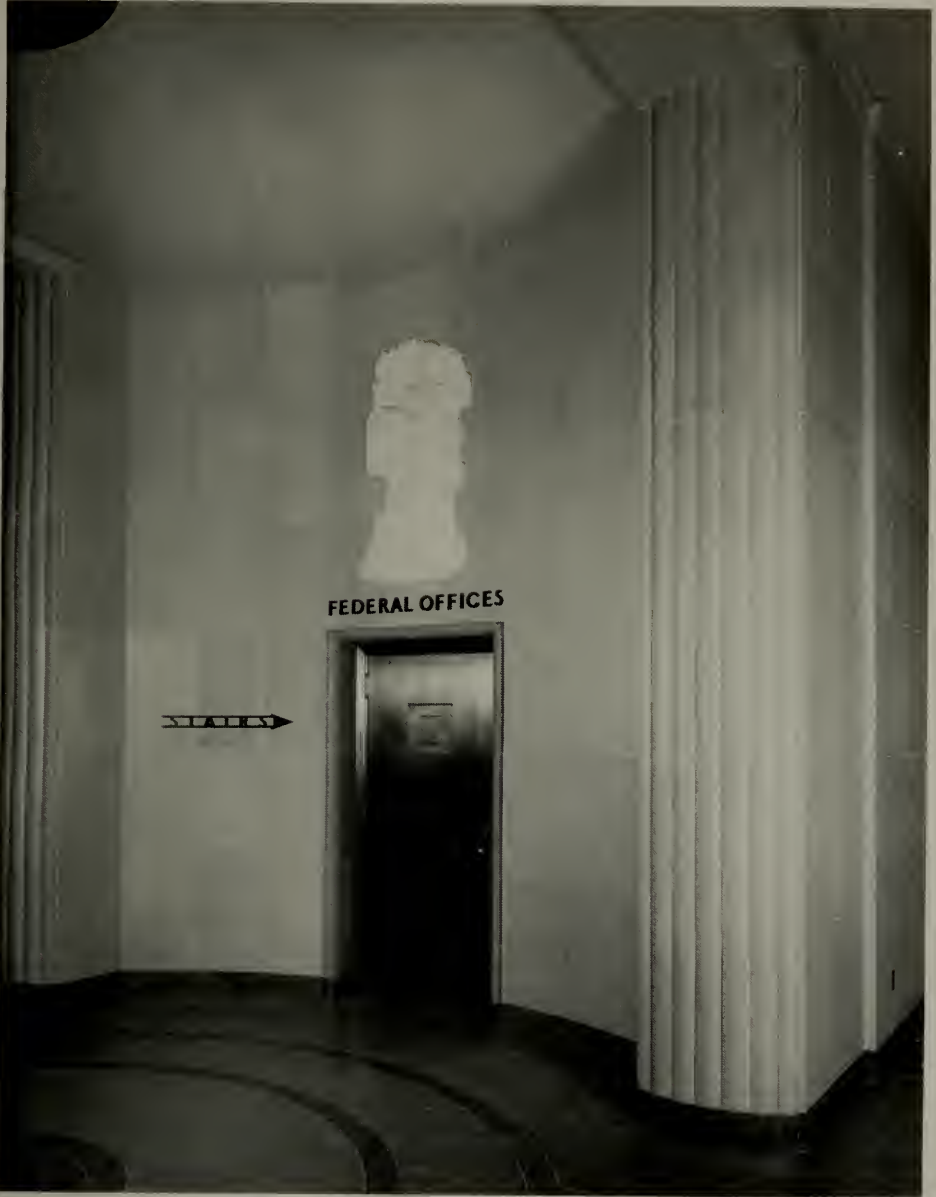
A VESTIBULE IN THE UNITED STATES POST OFFICE AT FRESNO, CALIFORNIA. THE WALLS ARE FINISHED IN ADHESION TYPE CERAMIC VENEER. THE UNITED STATES TREASURY DEPARTMENT IS ARCHITECT.
