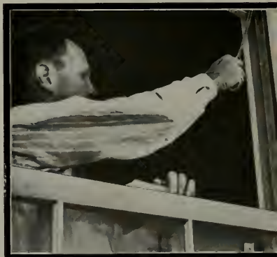
SHOWING EASE WITH WHICH WINDOW IS BALANCED
