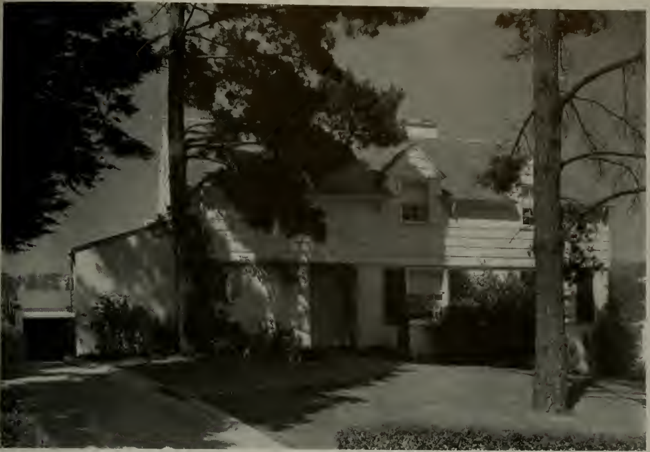
HOUSE FOR MR. AND MRS. FRED MONSEN, OAKLAND, CALIFORNIA Williams and Wastell, Architects
