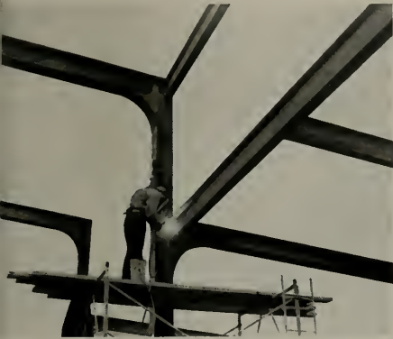
Welding steel frame of apprentice building
