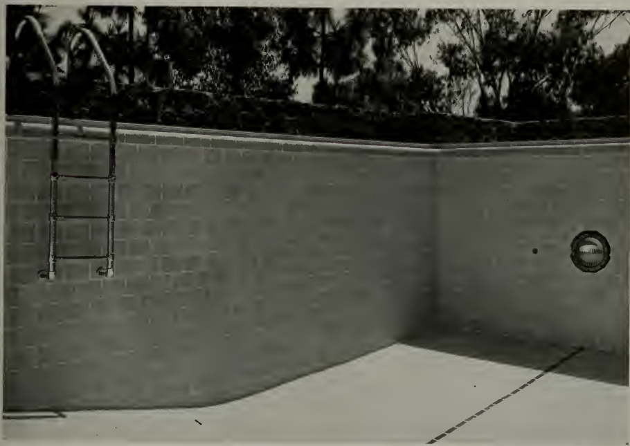
FLOOR AND SIDES OF POOL ARE 6X9 LAGUNA GREEN KRAFTILE. STEPS ARE A LIGHTER SHADE GREEN. THE 3-INCH LANE MARKERS ARE NIGHT BLACK.
