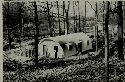
Construction methods: Pictured from top down— (1) Gunite or concrete shooting unit at left in background. Concrete base for half of housing unit in foreground; (2) Shooting Gunite onto chicken wire; (3-4) Front and side views of completed house.
