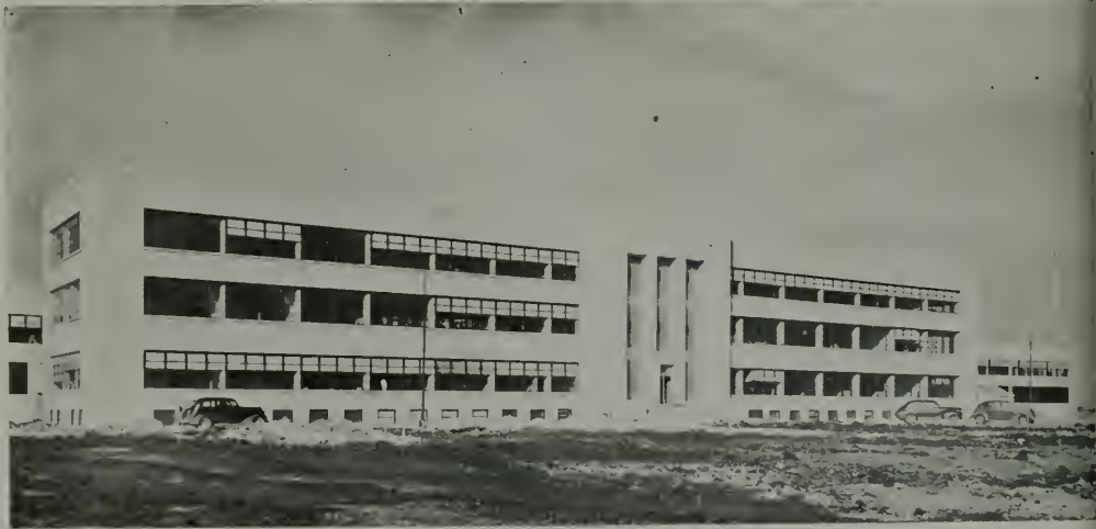
MAIN MANUFACTURING BUILDING, BUICK AVIATION ENGINE PLANT, MELROSE PARK, ILL.
