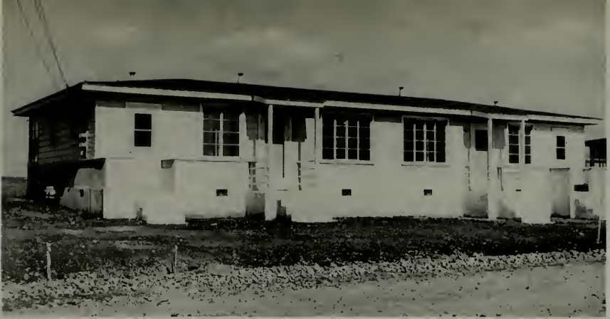
One of the completed two family dwellings
