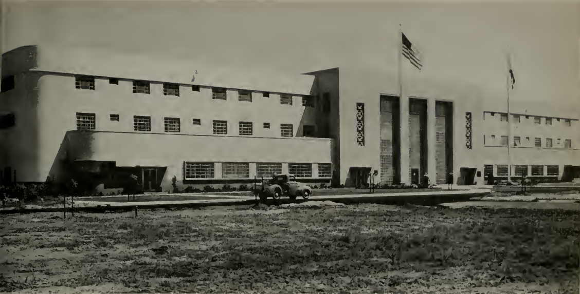
ADMINISTRATION BUILDING, STATE INSTITUTION FOR MEN, CHINO, CALIFORNIA
