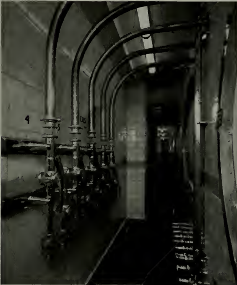
Government Celler contains four 100-barrel and eleven 250-barrel glass lined tanks. The Wall Units are Krafftile Ceramic Glazed, Cellular, they are ideal for a refrigerated room like this. Krafftile Vitreous 8 x 8 Quarry Tile is used to finish the floor here, in the Meter Room, and the entire working area of Machinery Hall. 13,300 square feet were used—the largest quarry tile installation in San Francisco last year
