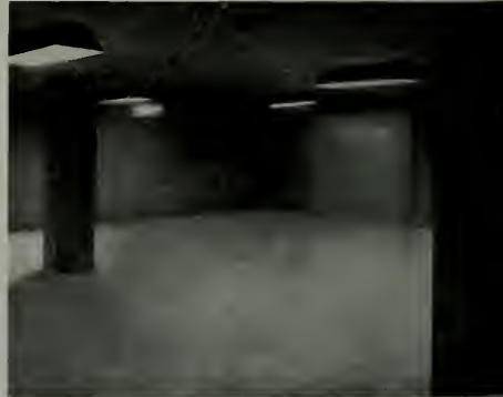
Above: Employees' Locker Room (before locker installation). Krafftile Structural Wall Units for personnel rooms and offices, employees' dressing rooms, lunch room are 6" x 12" Krafftile "Salt-Glazed" Structural Units thick with vertical cellular construction reinforced with grout where necessary. Partitions are glazed from floor to ceiling.
