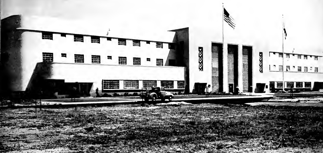
ADMINISTRATION BUILDING, STATE INSTITUTION FOR MEN, CHINO, CALIFORNIA
