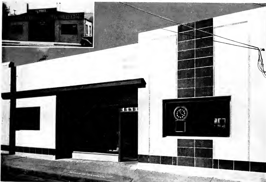
Small picture (upper left) shows neighborhood one story tire shop in Oakland, prior to converting into upholstery studio with Krafftile front.
