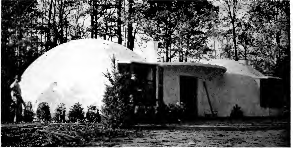
National Defense Homes Corporation of which Jesse Jones is head, is experimenting with this novel type of home at Falls Church, Va., from a patent applied-for design by Wallace Neff, architect, of Los Angeles.
