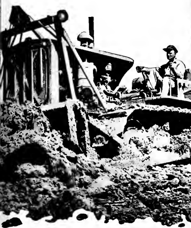
FOUNDATIONS FIRST. Before the airplane hangar (right) could go up, the hard-working bulldozer (above) had to dig up and level out the foundation. The bulldozer, with its tractor tread and colossal roar, is the building industry's private "tank."
