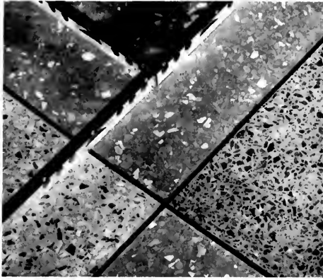
Plastic tenite for blocking off terrazzo floors and steps.
