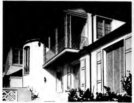
Balcony Detail, Residence of Felix Kahn, Seal Cliff, San Francisco Farr & Ward, Architects
