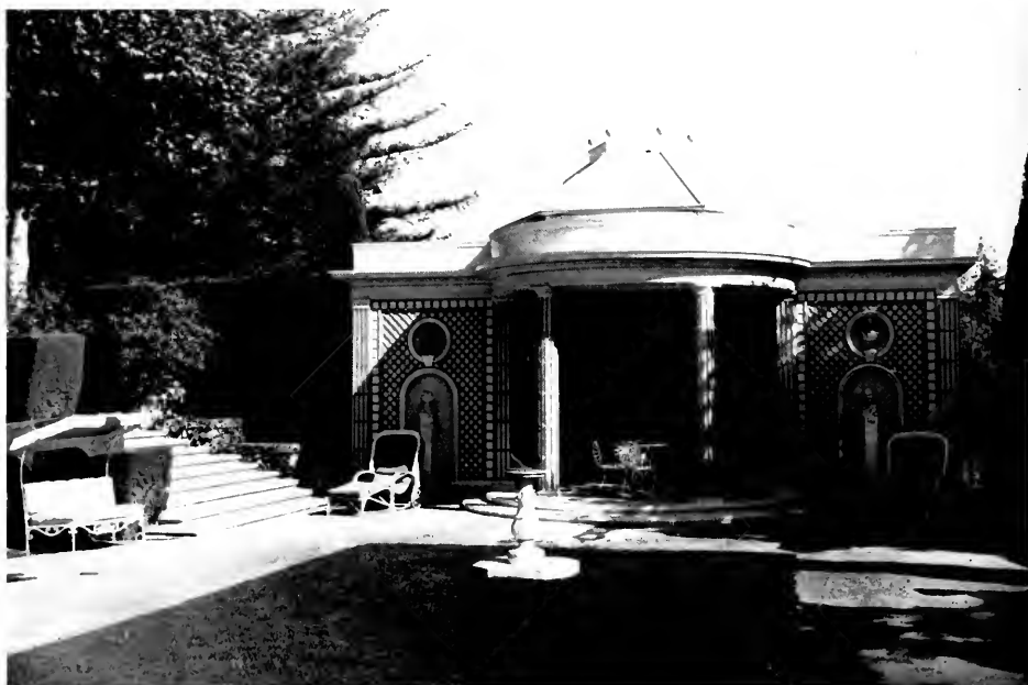
GARDEN AND SWIMMING POOL PAVILION, ESTATE OF MRS. DOROTHY SPRECKELS-McCARTHY, HILLSBOROUGH, CALIFORNIA
