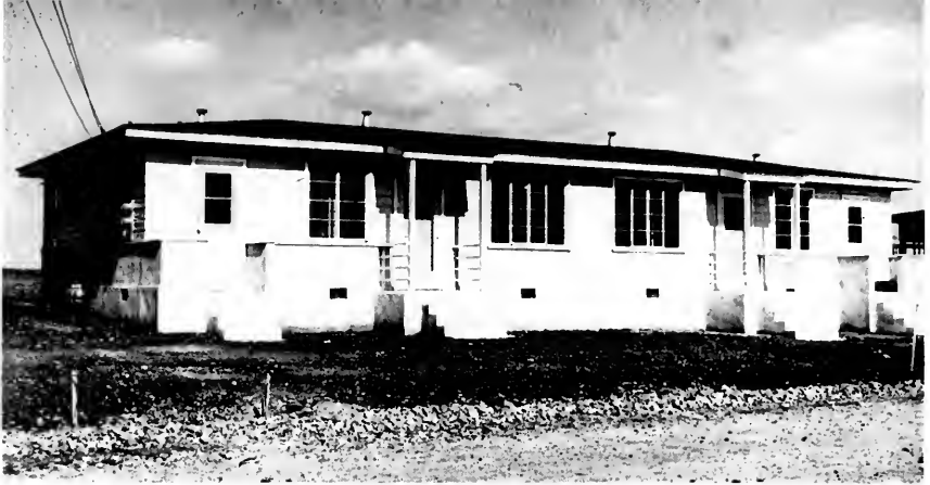
One of the completed two family dwellings
