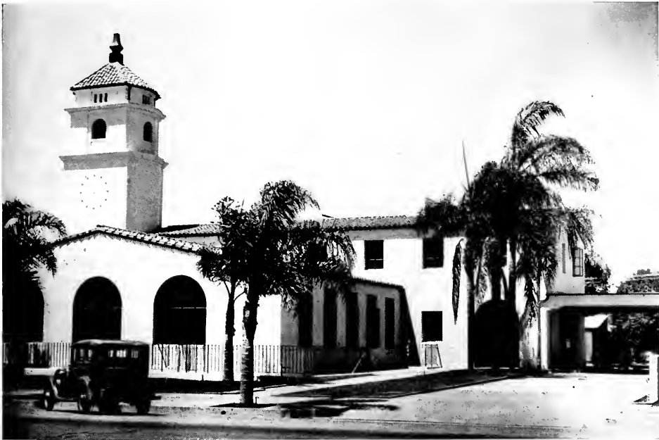
GENERAL VIEW OF FULLERTON CITY HALL, FULLERTON, CALIFORNIA
