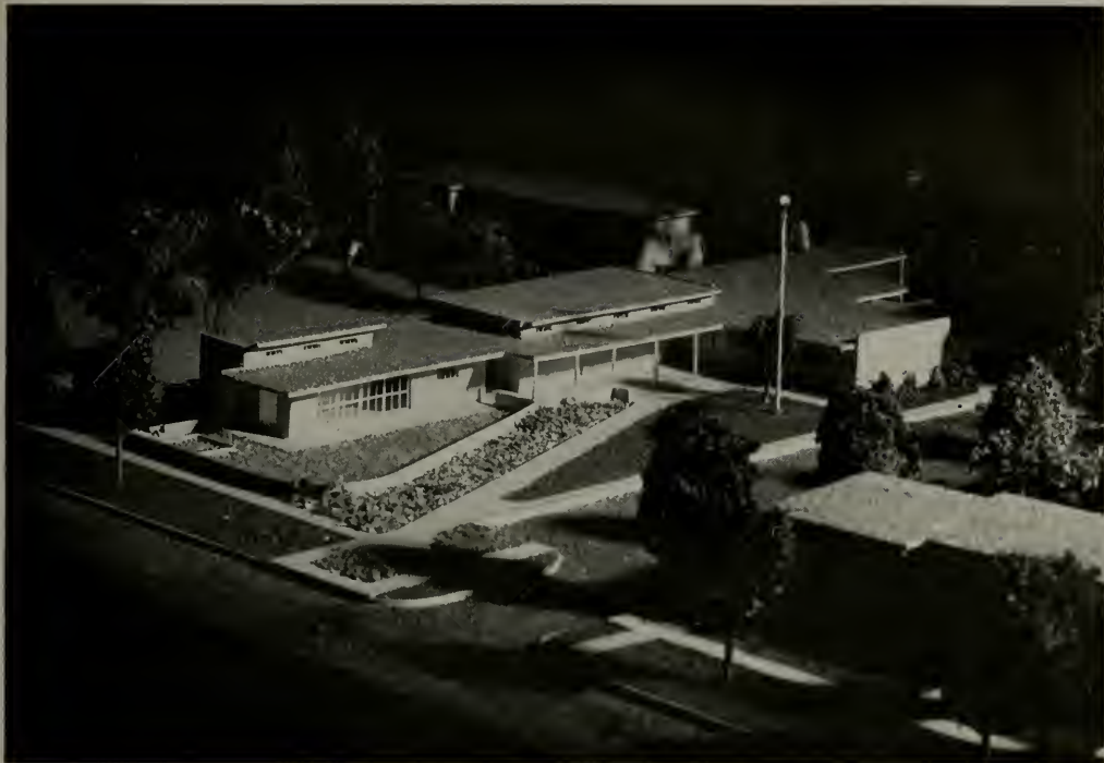
Administration building, a one-story structure with masonry walls. Building may also be used for community gatherings.
