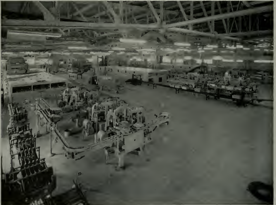
MACHINERY HALL, THE FIFTH FLOOR OF THE NEW BOTTLING PLANT, WHERE ALL BOTTLING, LABELING AND PACKAGING OPERATIONS ARE CONCENTRATED
