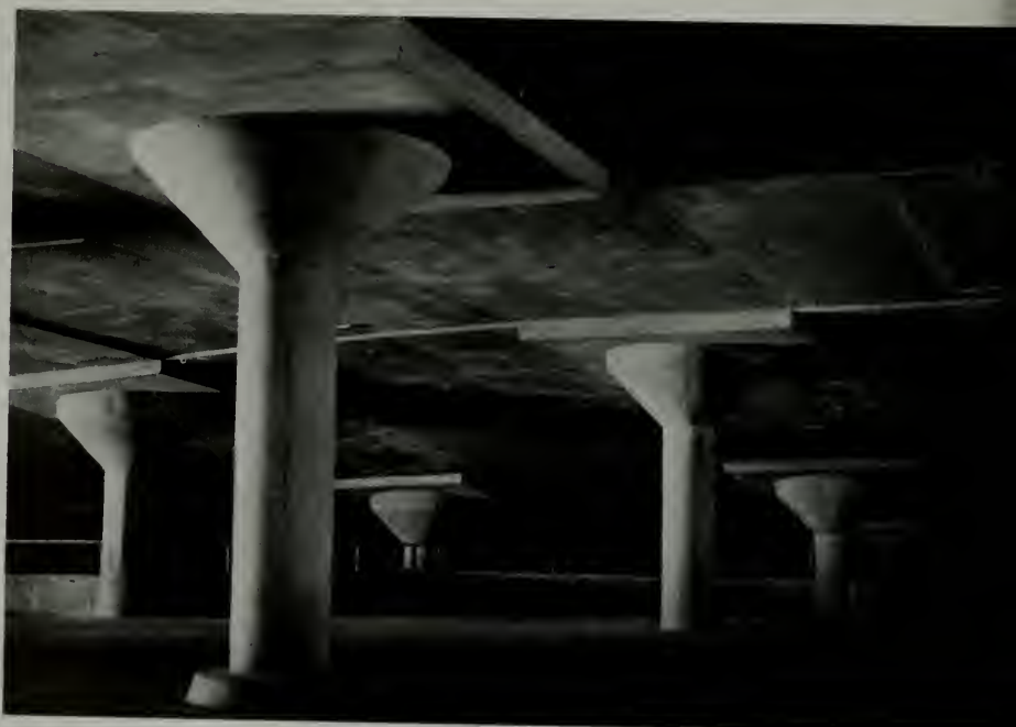
Irregular shaped columns, some 50 in number, serve as floor supports, formed in metal and installed by the Steel Form Contracting Company
