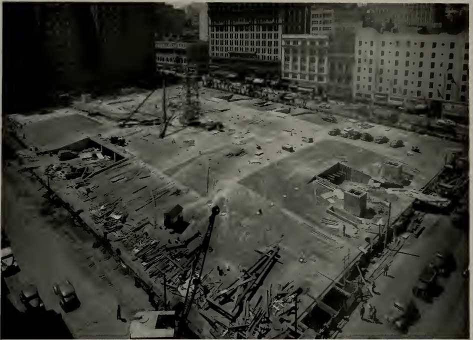
Union Square is 24 feet higher at the Powell-Post corner than at Stockton and Geary. The rise was gradual in the old park; in the new, a large level plaza necessitates this abrupt slope along Geary.
