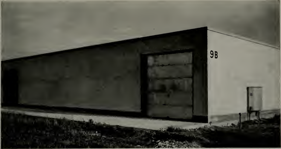
TYPICAL BUILDING OF INDUSTRIAL GROUP
